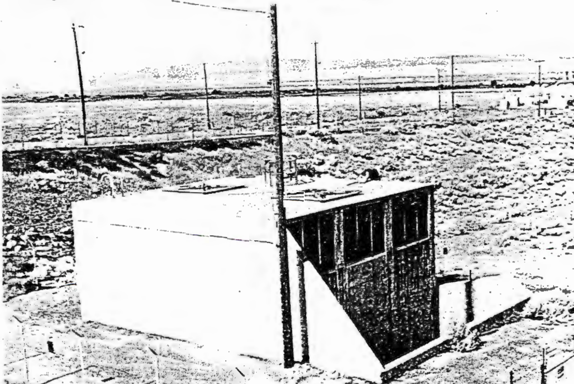
Figure 2-4. 1908-K Outfall (Only Outfall Currently in Use).
