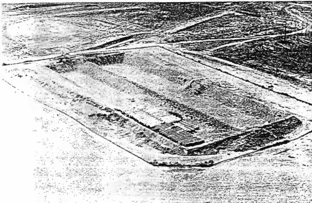
Figure 2-6. Sectioned Effluent Pipe Stored in 107-F Retention Basin.
