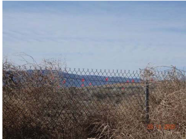
DSC# 02695 - Flags marking the exact location of the subsidence at NRDWL.
