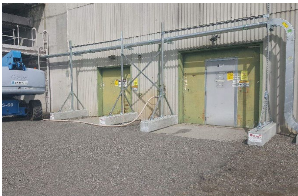
Conduit tray installation for routing power from the Skid-Mounted Substation to 105KW
