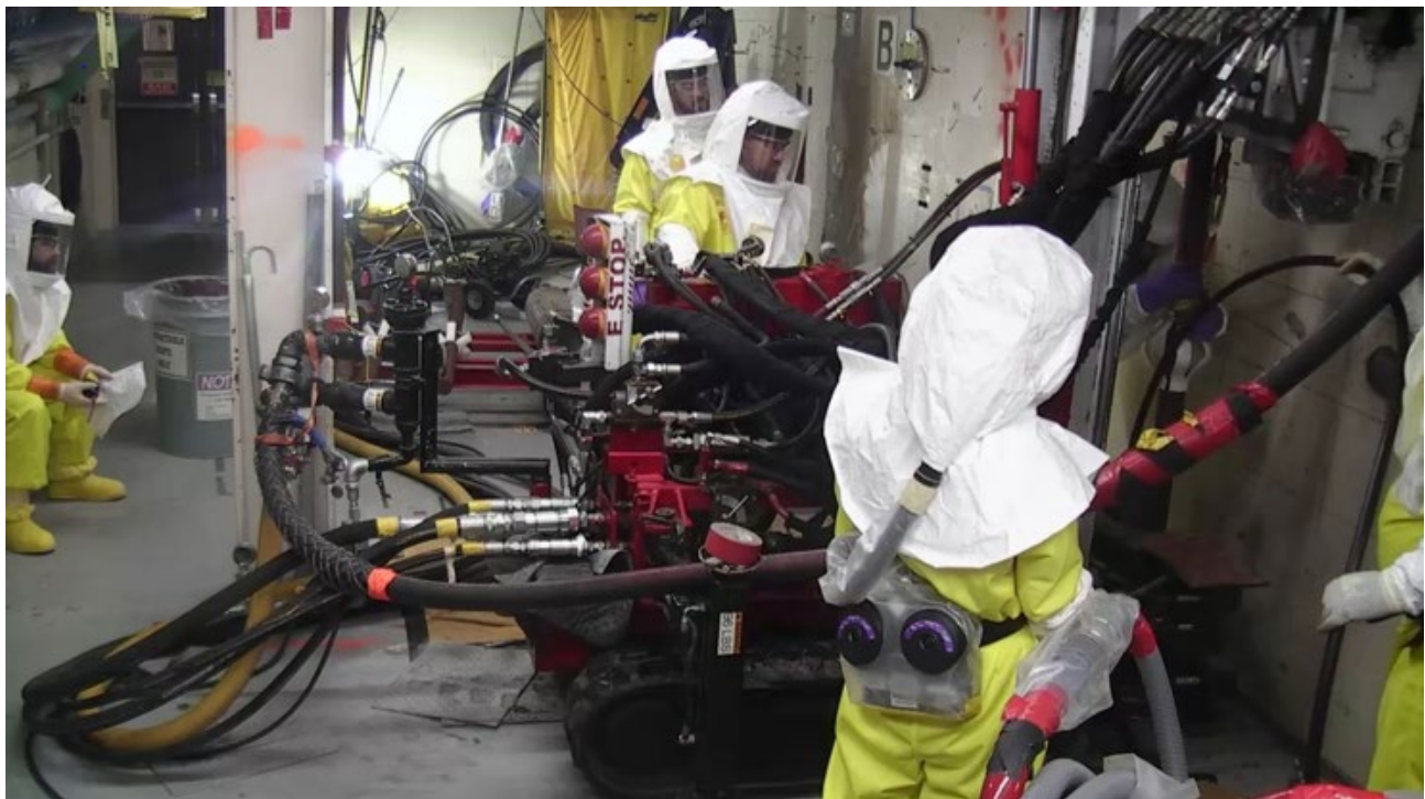
Installation of micropile steel core
