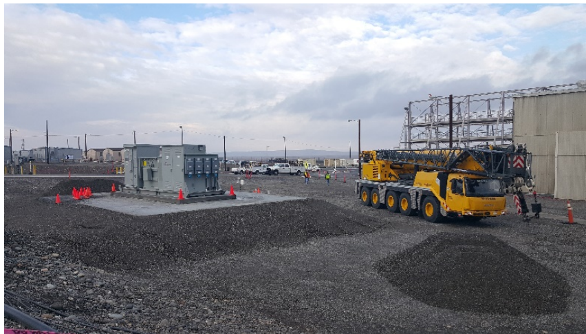
Skid-mounted substation placed onto constructed pad with crane
