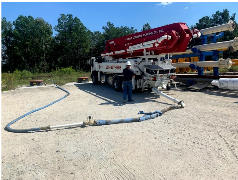
Filling practice VPC with grout at Contractor's facility in Texas
