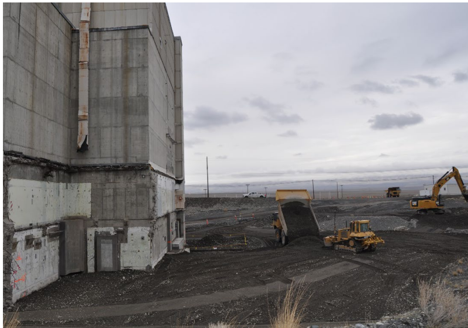
105KE ISS Foundation Backfill Operations
