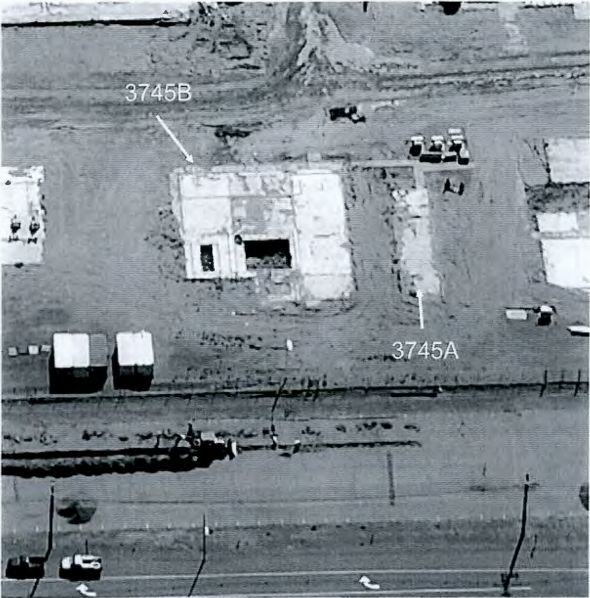
Figure 4. 3745A and 3745B after above-grade demolition on July 16, 2008
