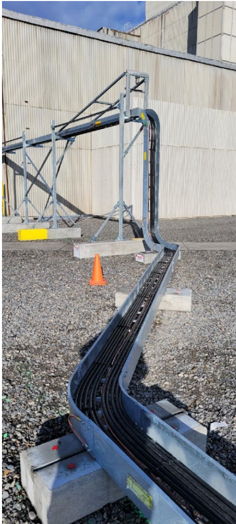
Secondary wiring installed from the Skid-Mounted Substation to the 105KW Electrical Room
