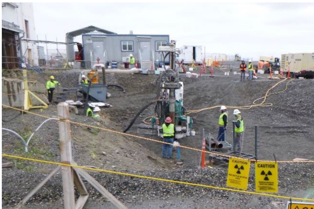
Drilling for Temp Shoring
