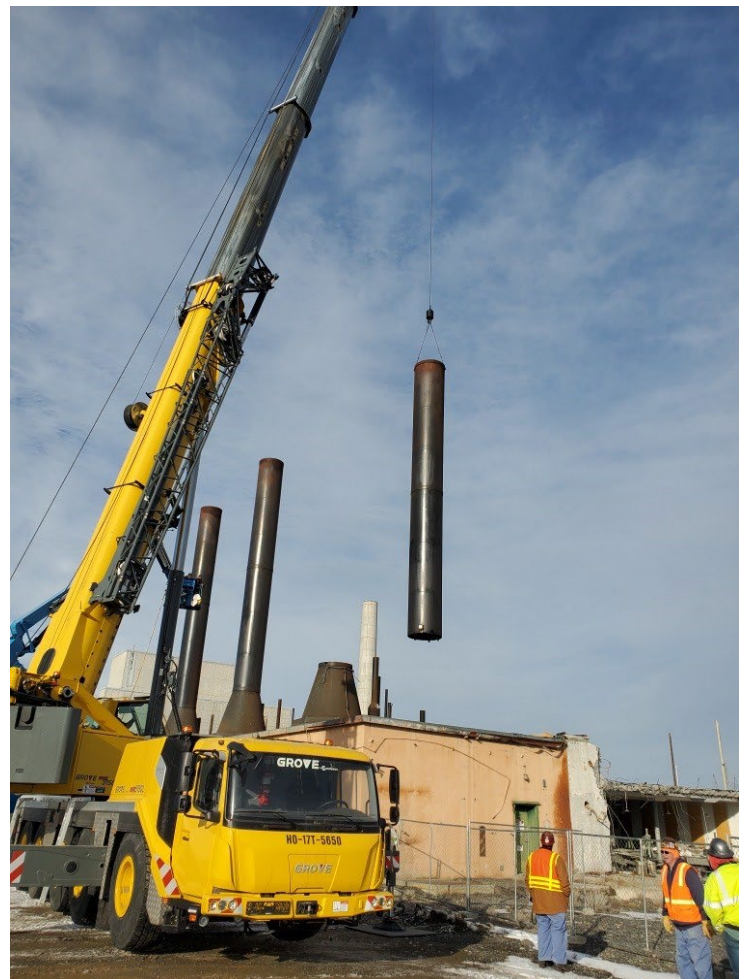
165KW Demolition Stack Removal Progress
