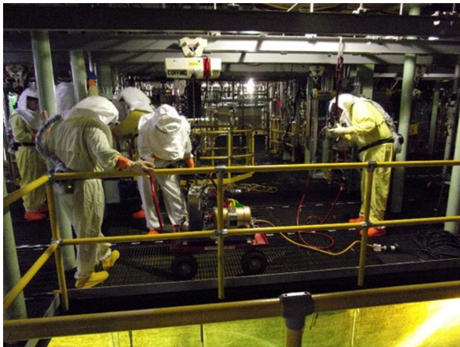
Operating Champion Shear to Cut Floor Pole Tools
