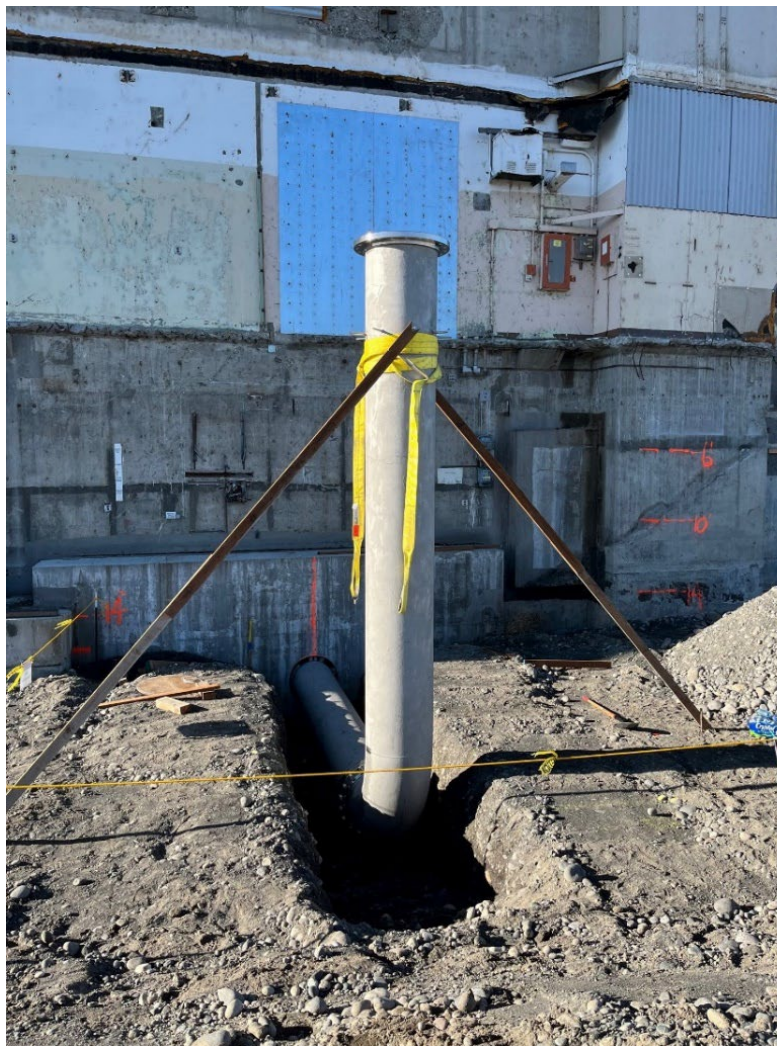
Installed Ventilation Pipe
