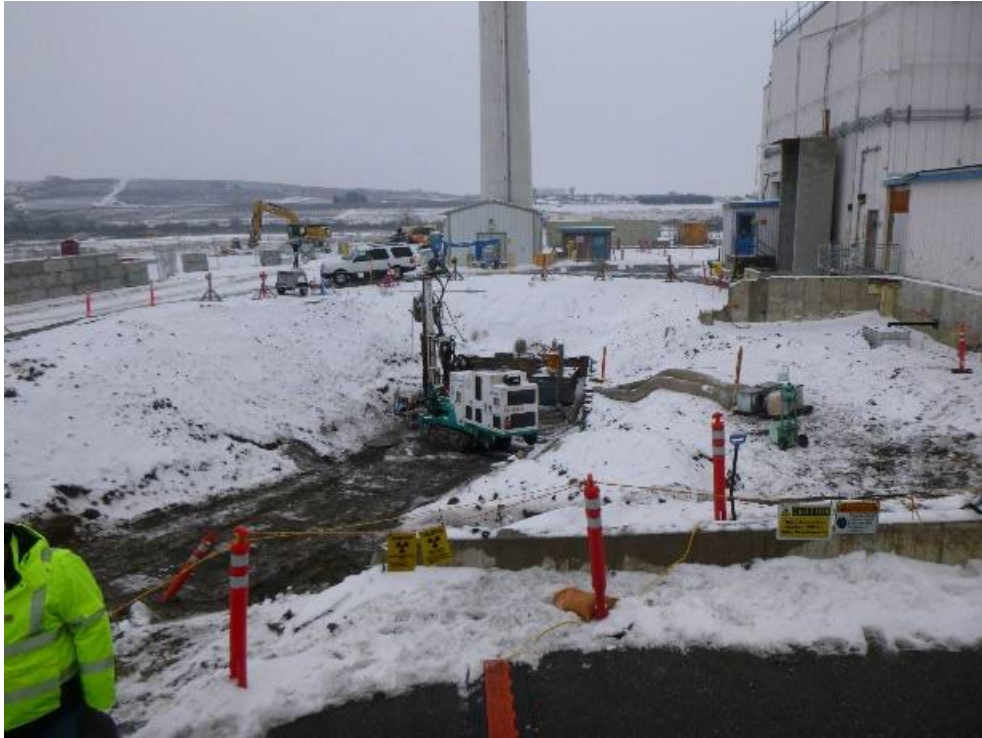
Temp Shoring Drill Rig
