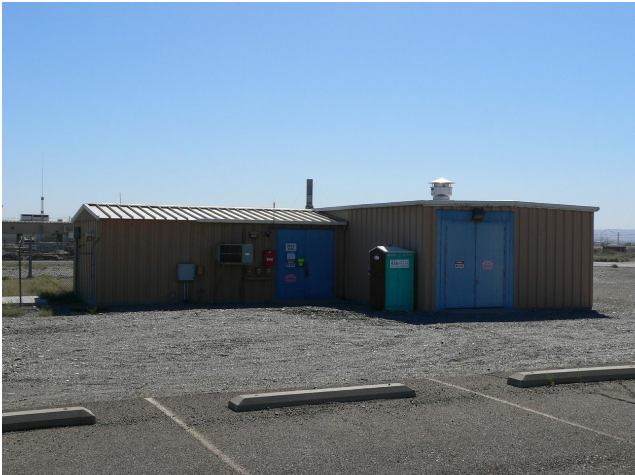
Figure 8. 352-F Switch Station (September 8, 2005).
