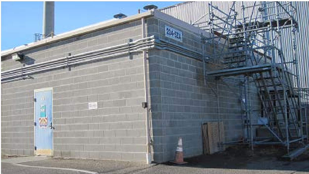
Figure 2. Northeast Corner of 234-5ZA Building Exterior (Cinderblock Construction)
