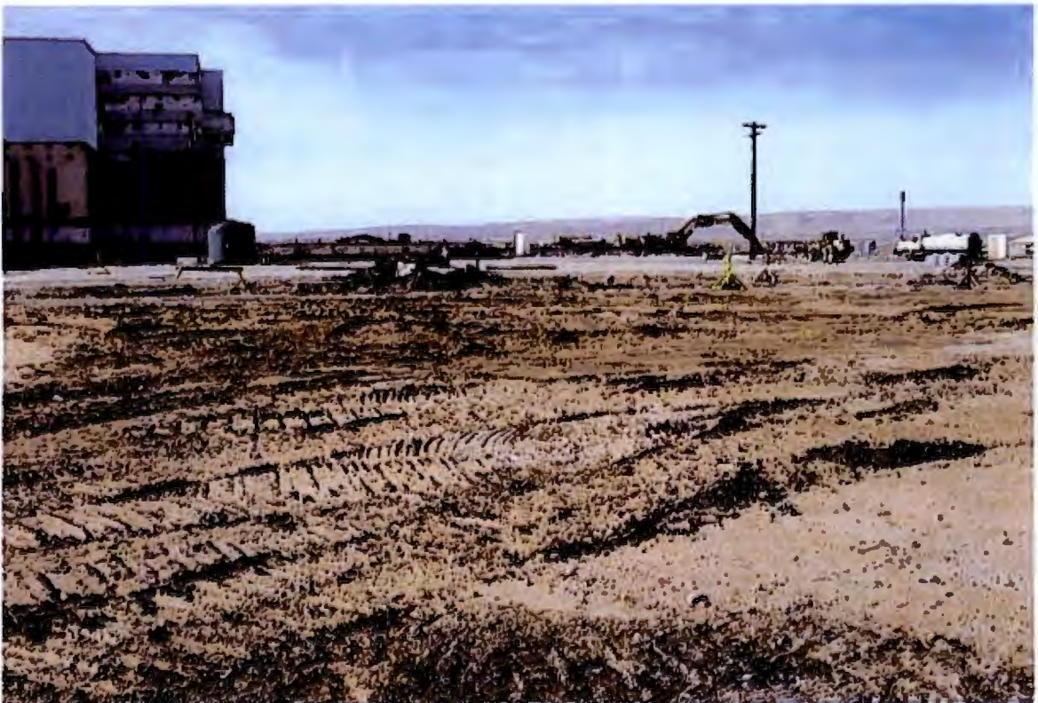
1119-N FACILITY COMPLETION
