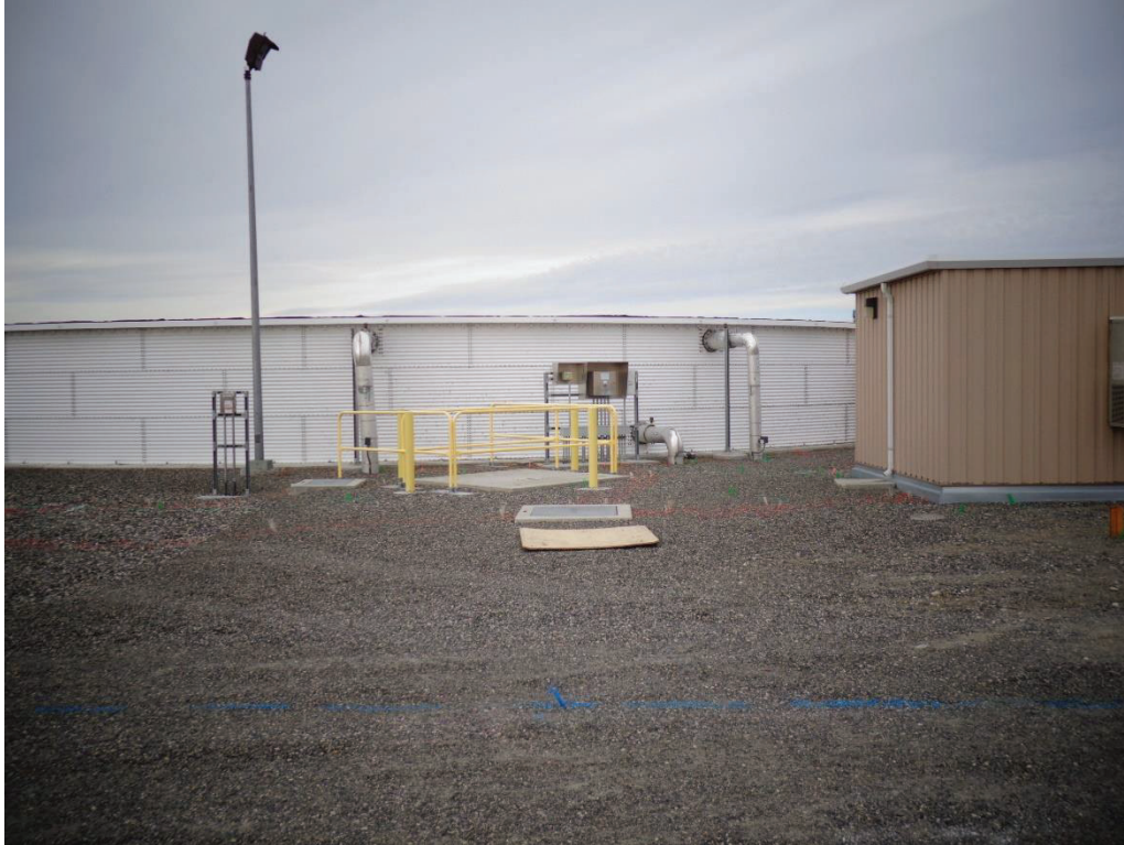
Pic#3 – Facing West, Leachate Tank & Transfer Building Cell 1
