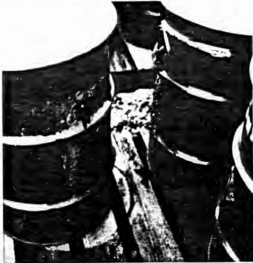
FIGURE 5. Photographs of Corroded Drums
