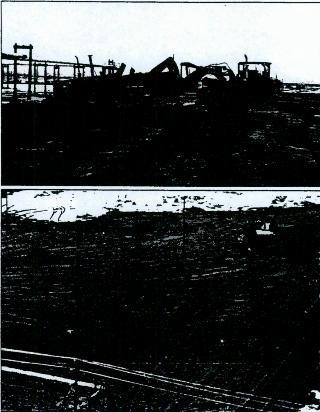
FIGURE 45. Backfilling the 203-S, 204-S, 205-S Site with a Scraper (top) and Performing Final Contouring with a Bulldozer and Grader (bottom). After final grading, the area was mulched and seeded with wheatgrass to stabilize the soil.
