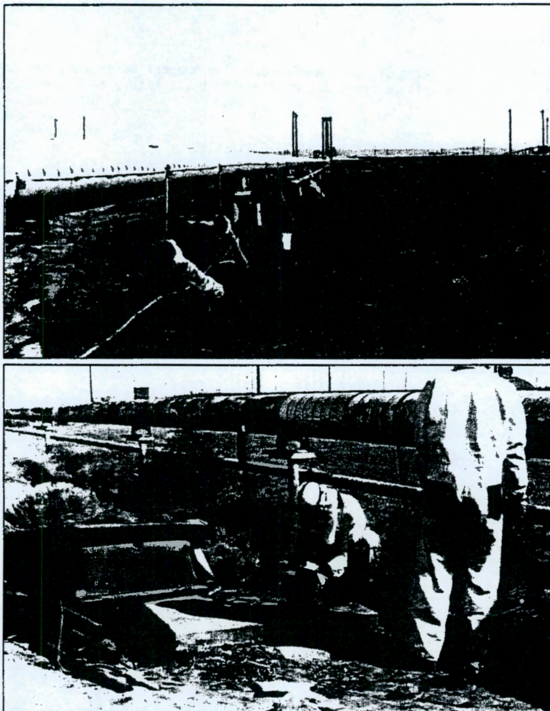
FIGURE 11. Dismantling the Cross-Country Section of the Uranium Nitrate Hexahydrate Line. Note cut-and-wrapped pipe sections (top), and dismantling a pipeline heat trace station (bottom).
