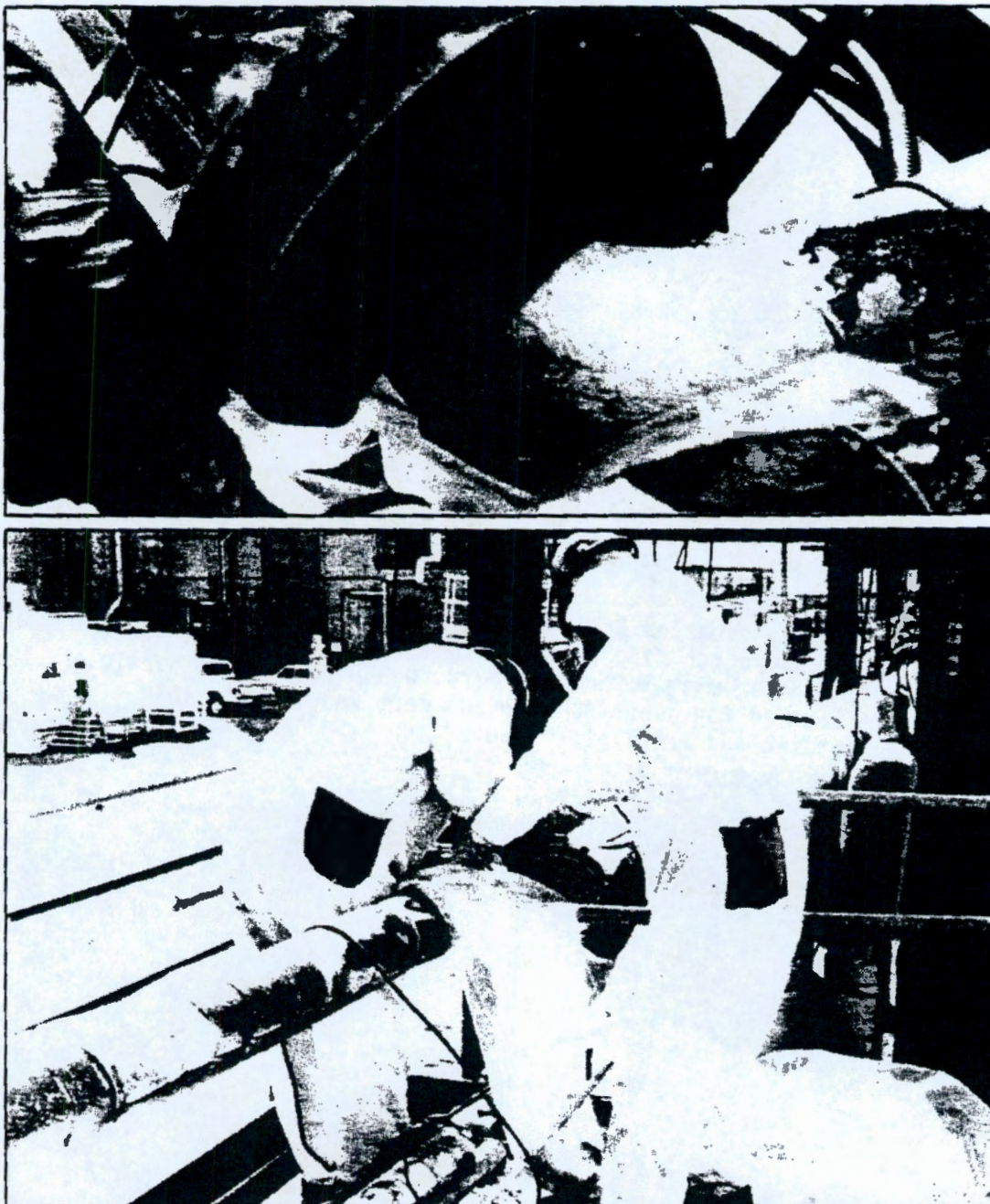
FIGURE 9. Pipe Cutting Operation. A hydraulic crimper (top) was the preferred cutting tool for piping 2 in. or smaller in diameter because the crimper sealed the pipe ends except for two small pinholes. A portable bandsaw (bottom) was used for large-diameter piping where the crimper could not be utilized.
