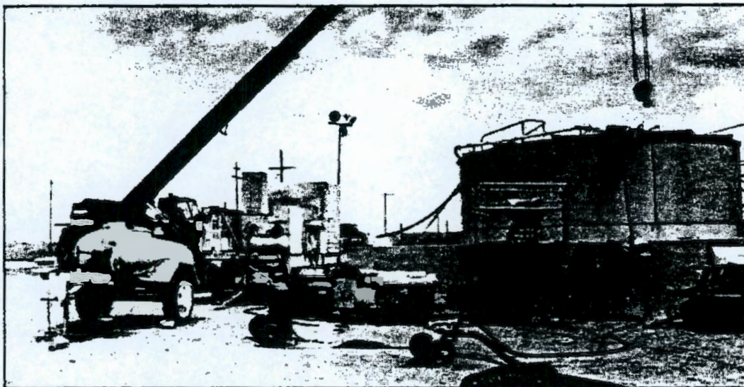
FIGURE 31. Sluicing Support Equipment Outside the Tank. A large array of equipment was required for hot water sluicing, including the high-pressure pump, portable motor starter, diesel generator, and fuel trailer in the foreground. The 7,000-ft 3 /min Portable Exhauster (left center) was used to draw vapors from the tank and to maintain a vacuum in the vessel.
