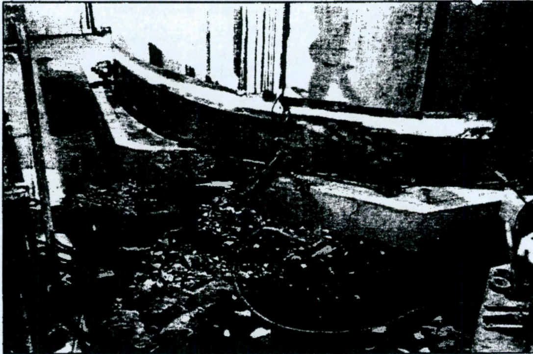
FIGURE 34. Using a Jackhammer to Remove the Tank Drain Line from the Concrete Tank Pedestal. Note the lead sheeting taped to the tank wall to reduce radiation exposure to the jackhammer operator.
