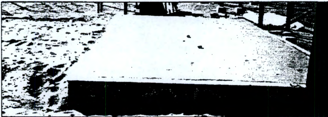
FIGURE 17. The 203-S Basin After Filling with Compacted Soil.
