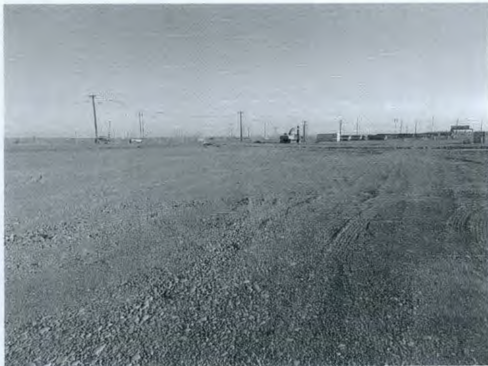
Figure 4. Looking north at 3705 and 3705BA following backfill in July of 2012.
