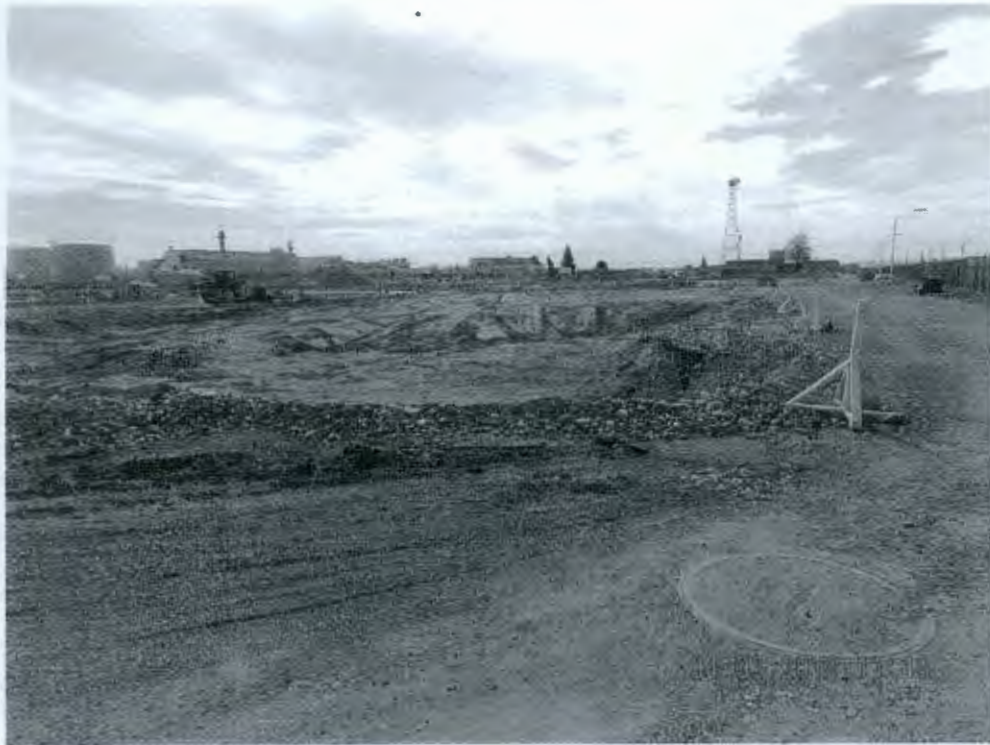
Figure 3. Looking south at 3705 and 3705BA following slab removal in April of 2012.
