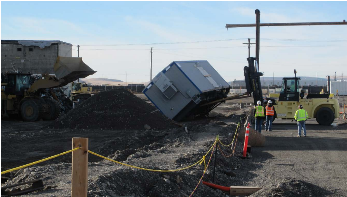
Figure 2. MO2501 During Demolition
