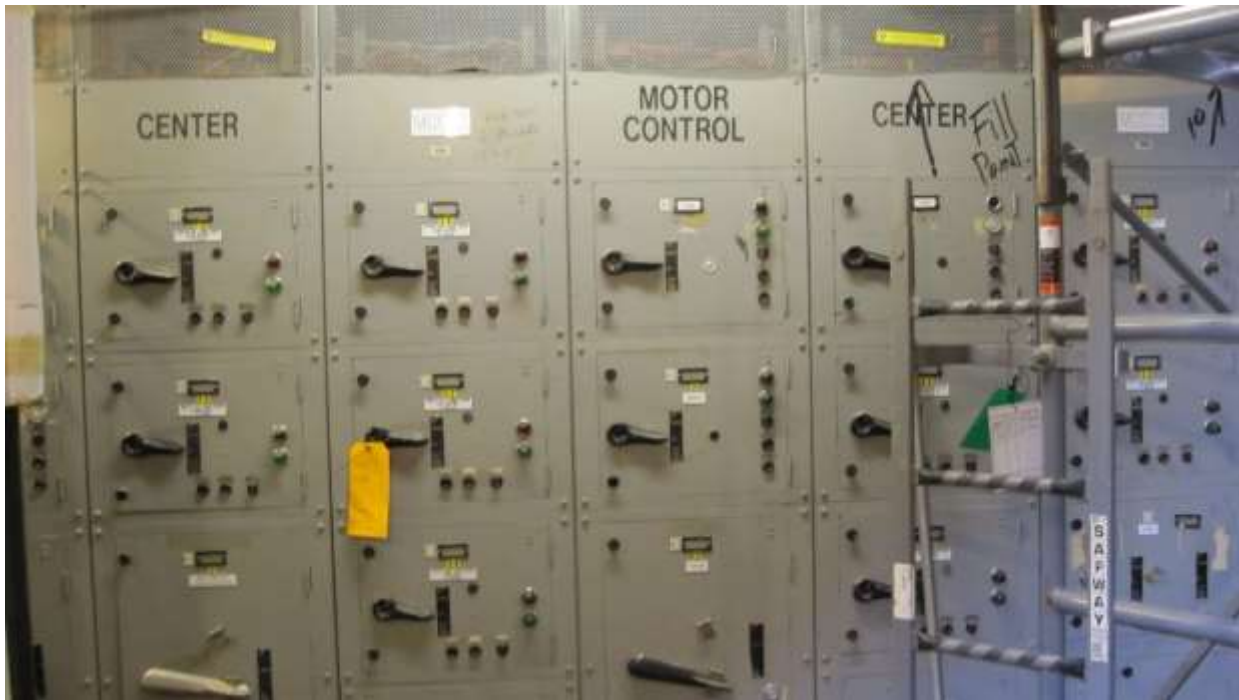
Figure 6. Room 501, Electrical Switchgear (21 Buckets)
