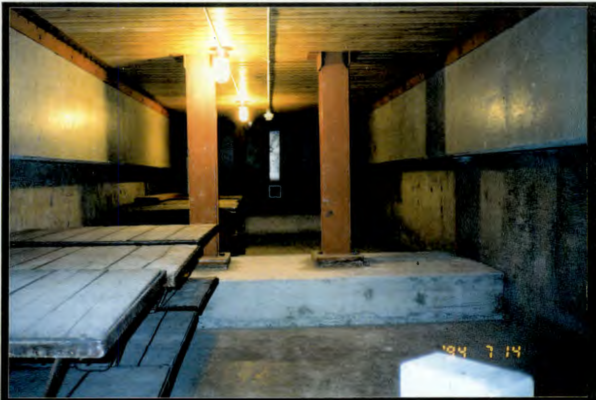
PHOTO #21 – H-52-L North Bunker (Former Missile Storage Area). Wood ceiling, columns and concrete foundation recently installed.
