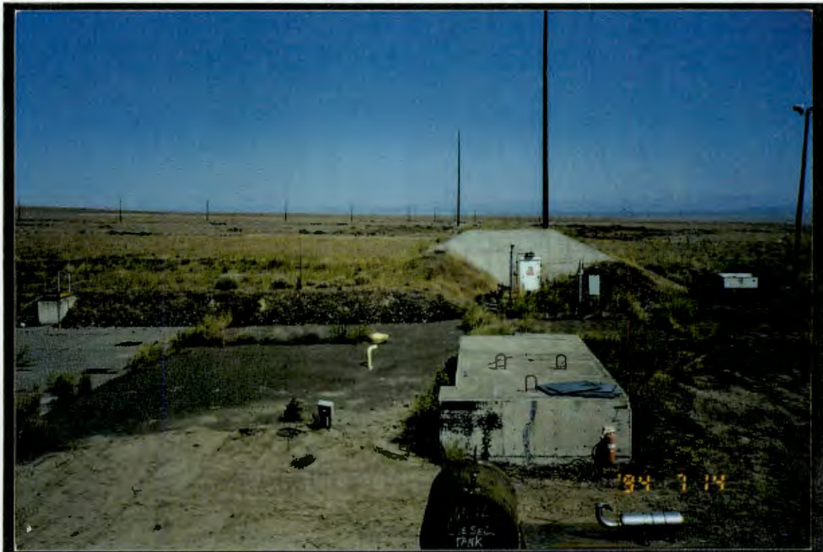
PHOTO #20 – H-52-L North Bunker entrance on ALE Reserve. Soil mound covers where missile elevator doors were once located.
