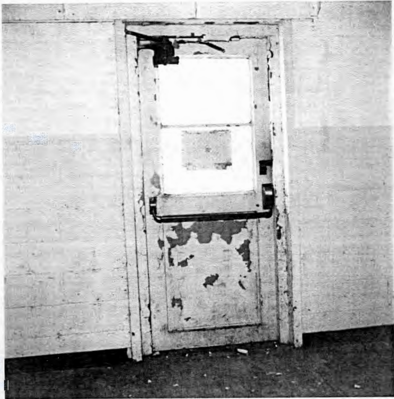
Photograph 6. Peeling Paint in the Lunch Room.
