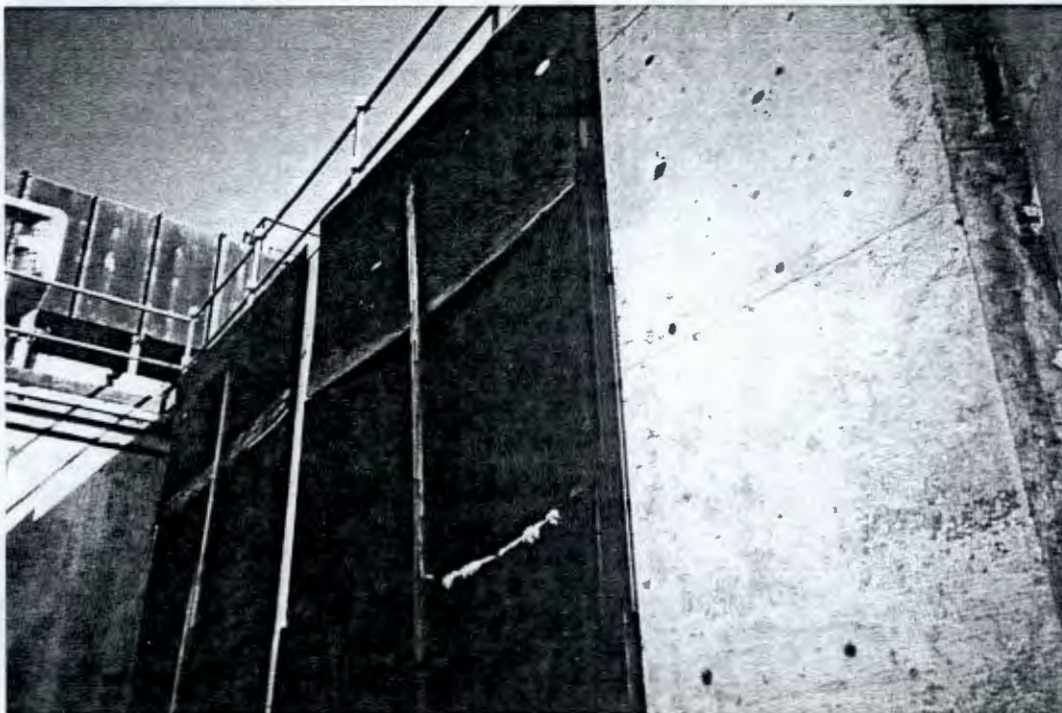
Photograph 3. Wood Covers Over the Stack Plenum Openings.
