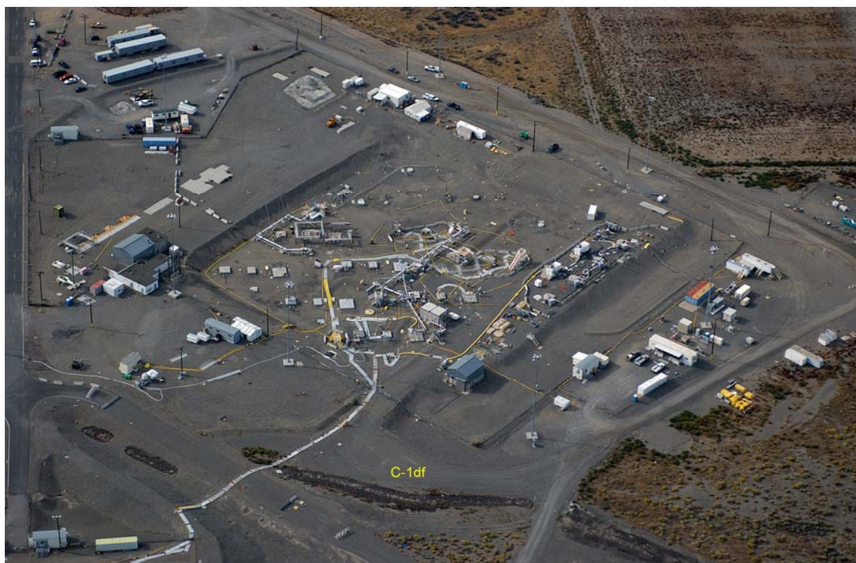
Figure 8-1. Aerial Photograph of WMA C during Active Tank Waste Retrievals (2008)
