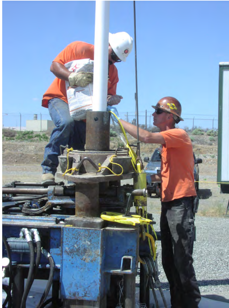
Figure 3.13. Silica sand was added to the well annulus between the 4-in. PVC well casing and 6-7/8-in. (ID) temporary steel casing during well construction. Hydraulic casing jacks, located in center, were used to back pull the temporary casing during well construction.
