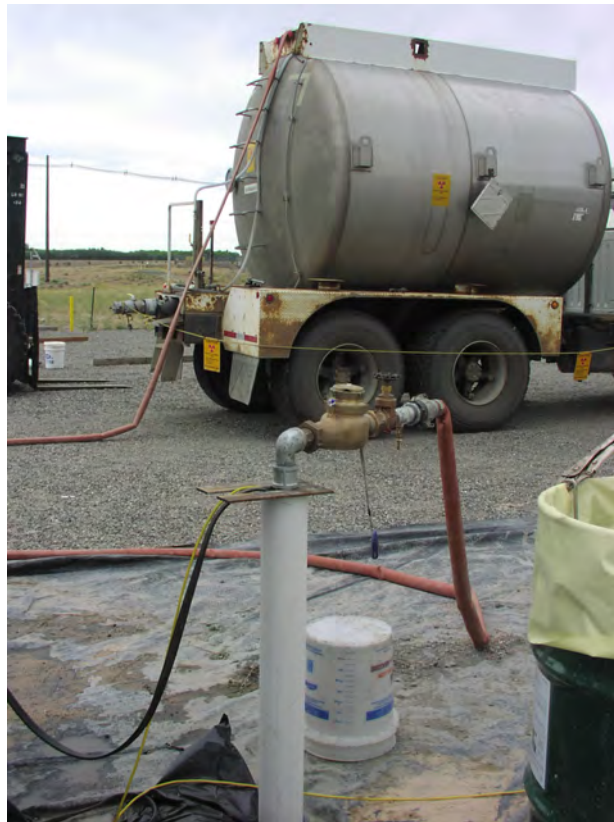
Figure 3.16. Water was pumped out of 4-in. PVC wells into a storage tank during well development.
