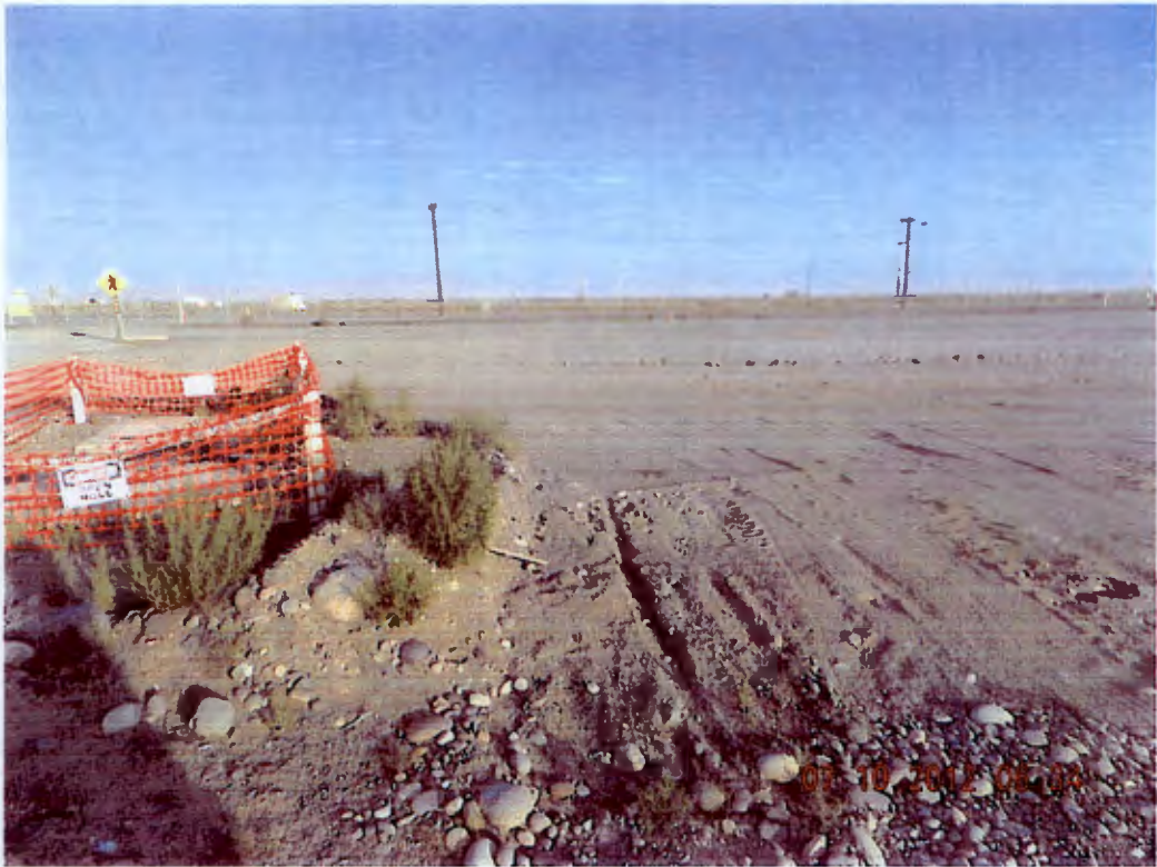
Figure 4. Looking west at 3719 following backfill in July of 2012.
