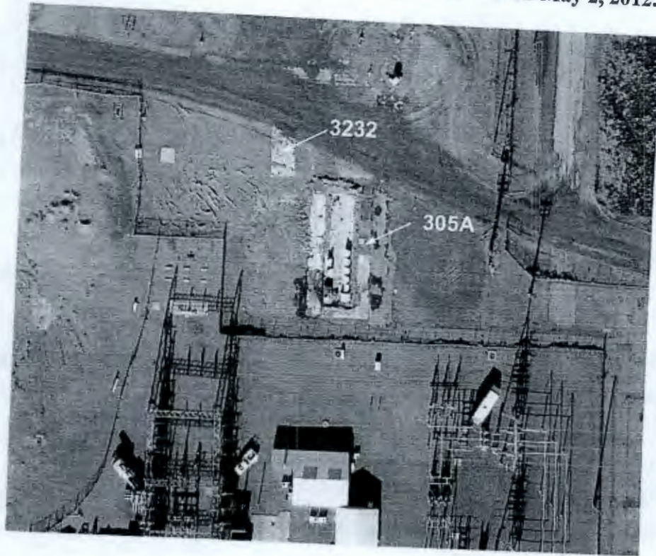
Figure 3. 305A and 3232 Slabs prior to demolition on May 2, 2012.
