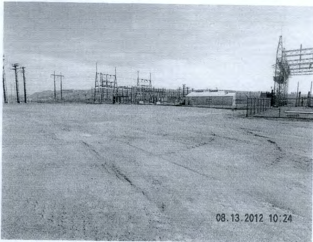
Figure 5. Looking northeast at 305A and 3232 following backfill on August 13, 2012.
