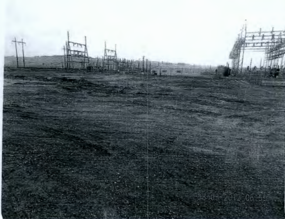
Figure 4. Looking east at 305A and 3232 following slab removal on August 8, 2012.
