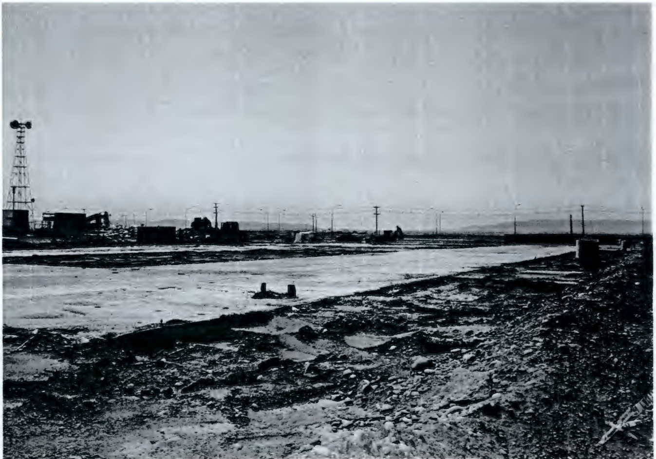
View of 3706 Concrete Slab from the Northeast (May 2006)
