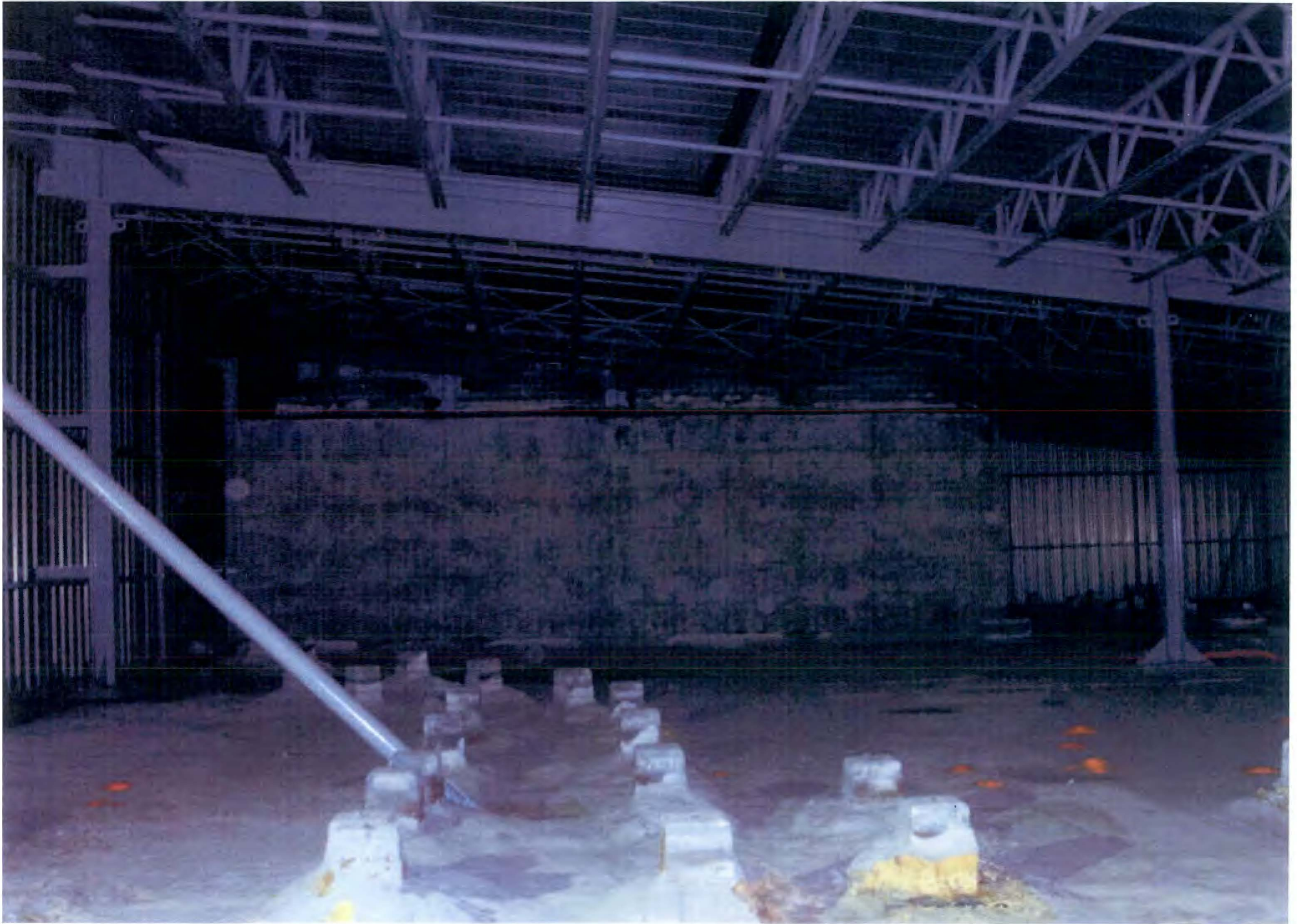
PHOTO # 104/109N/Area Under SSE Roof-East Vent Valve Struct. Looking East/EI.40'/02-07-2012
