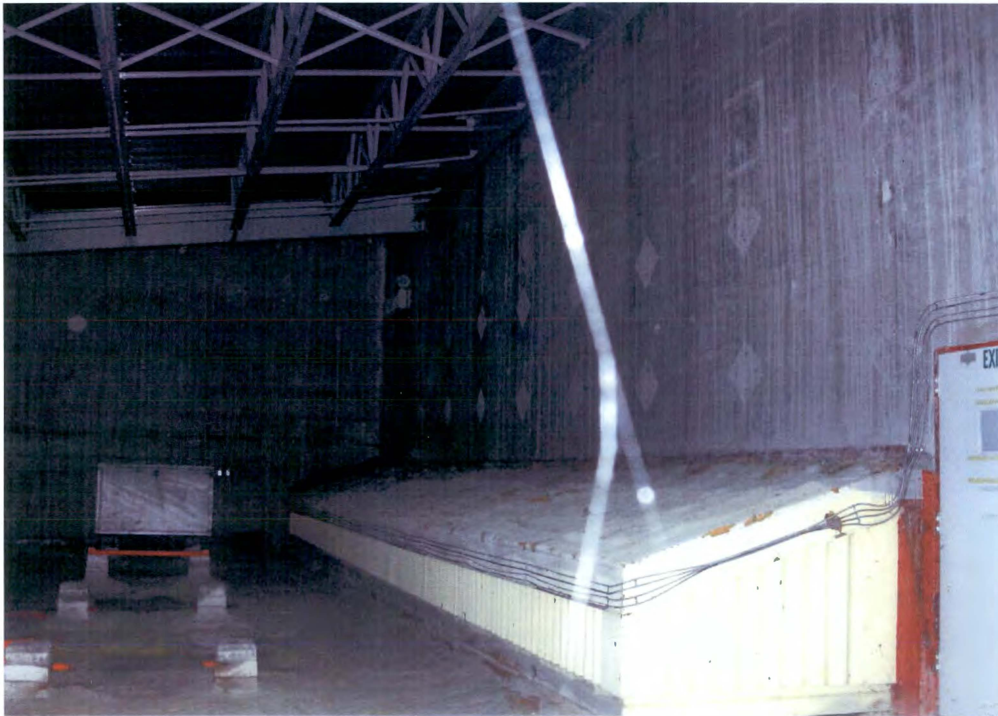
PHOTO # 108/109N/Area Under SSE Roof-North Wall E. of Press./El.40'/02-07-2012
