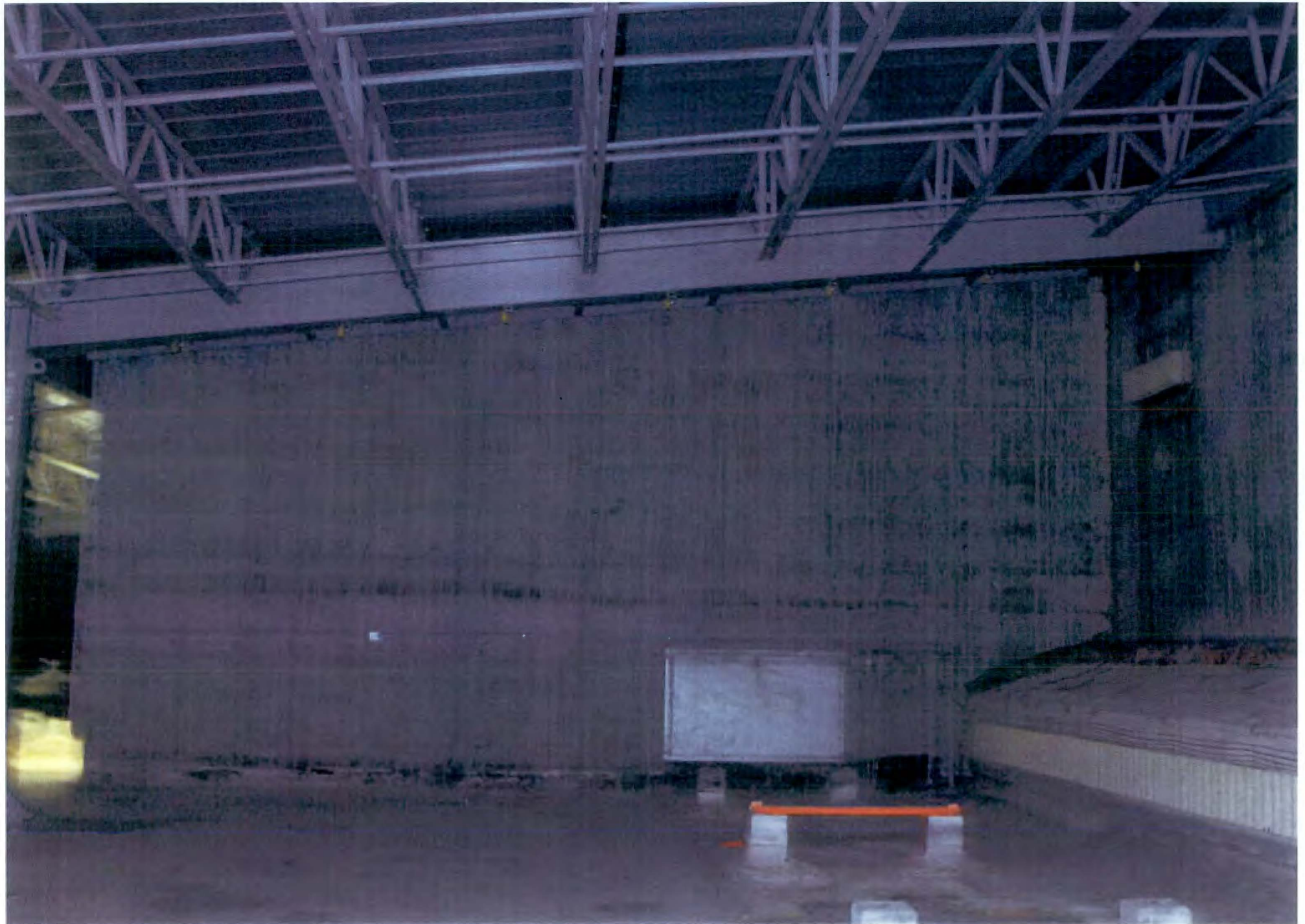
PHOTO # 109/109N/Area Under SSE Roof-E.Wall of Press./El.40'/02-07-2012
