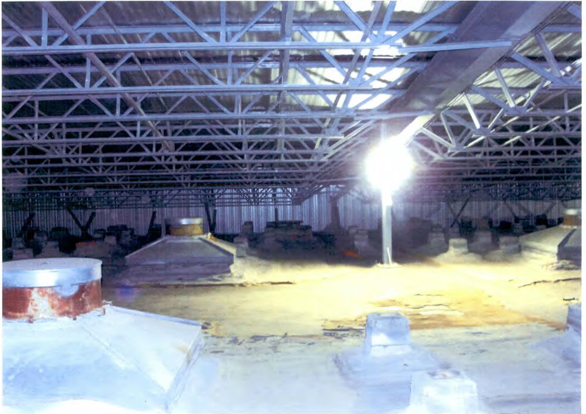
PHOTO # 107/109N/Area Under SSE Roof-South Wall E.End/EI.40'/02-07-2012
