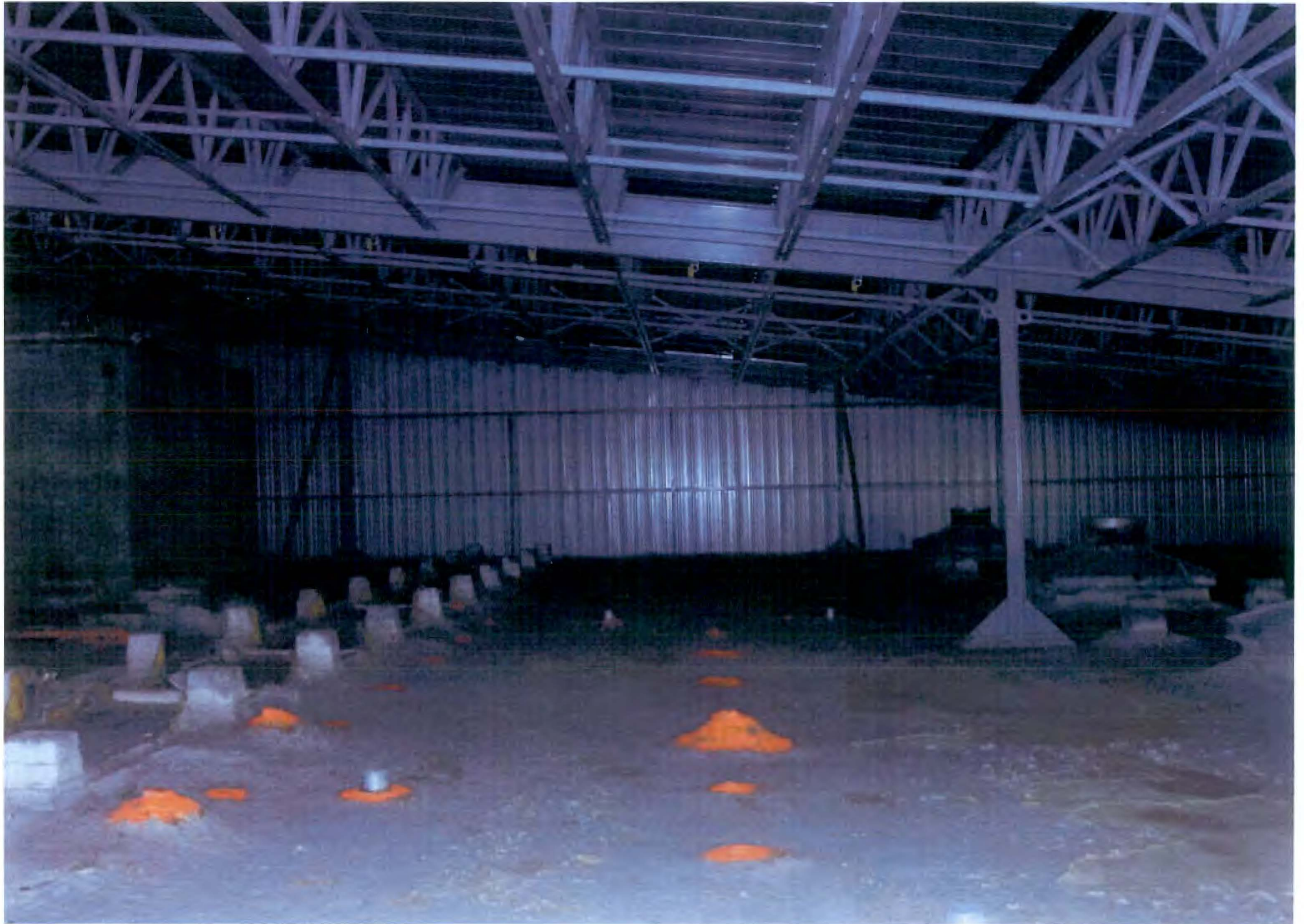
PHOTO # 105/109N/Area Under SSE Roof-East Wall Ctr./El.40'/El.40'/02-07-2012
