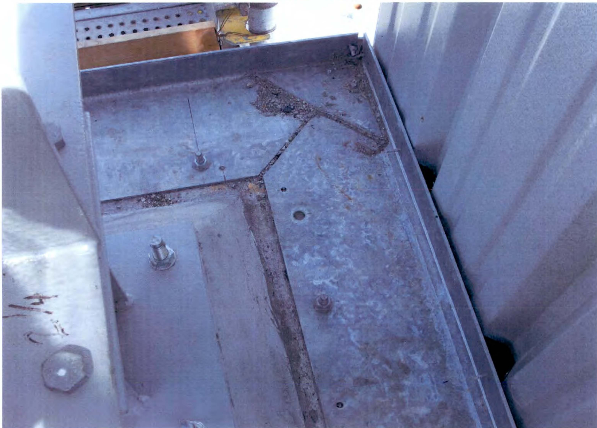
PHOTO # 124/109N Pressurizer/SSE Roof-Bent Pl.Closure/04-06-2011
