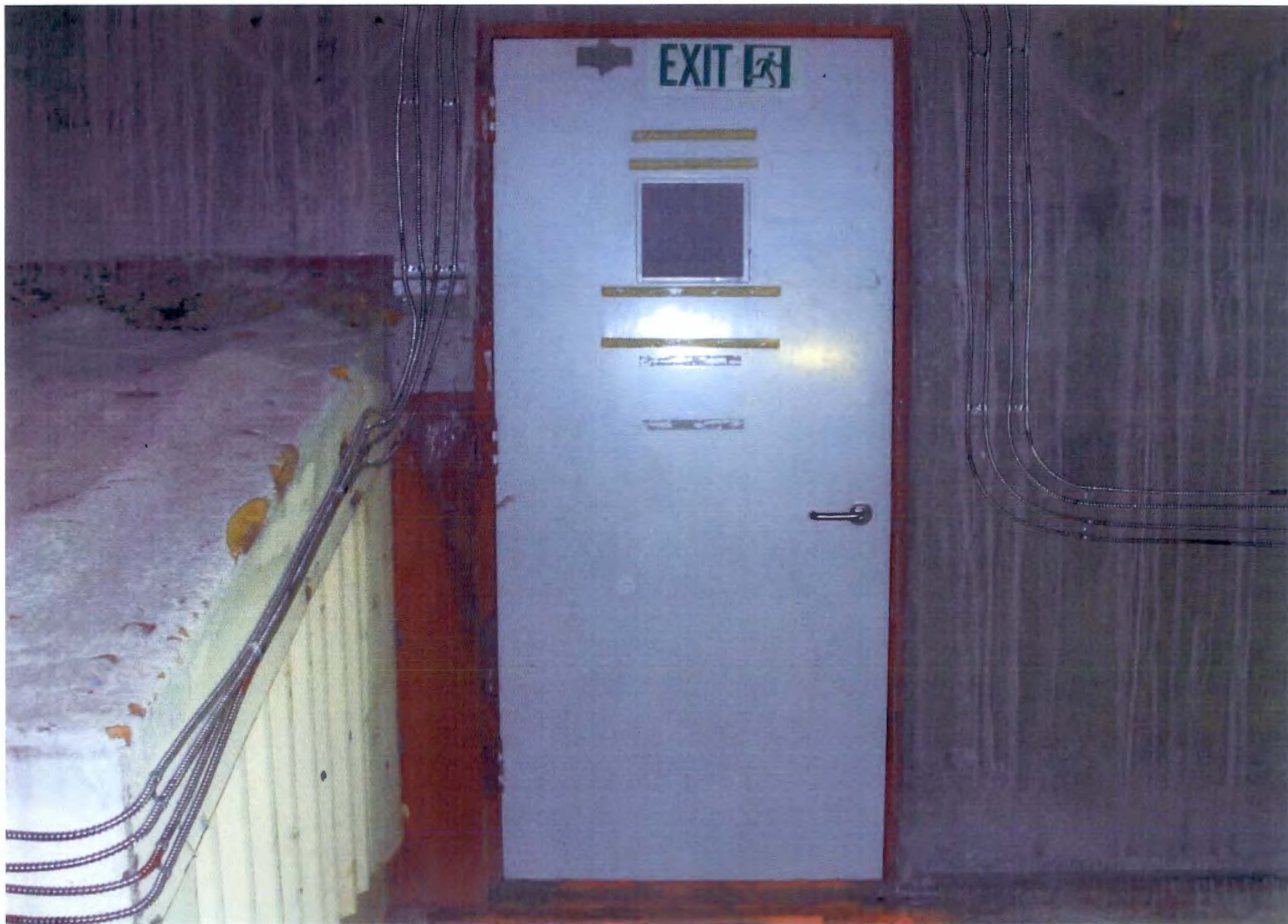
PHOTO # 102/109N/Area Under SSE Roof-Access Door/EI.40'/02-15-2012
