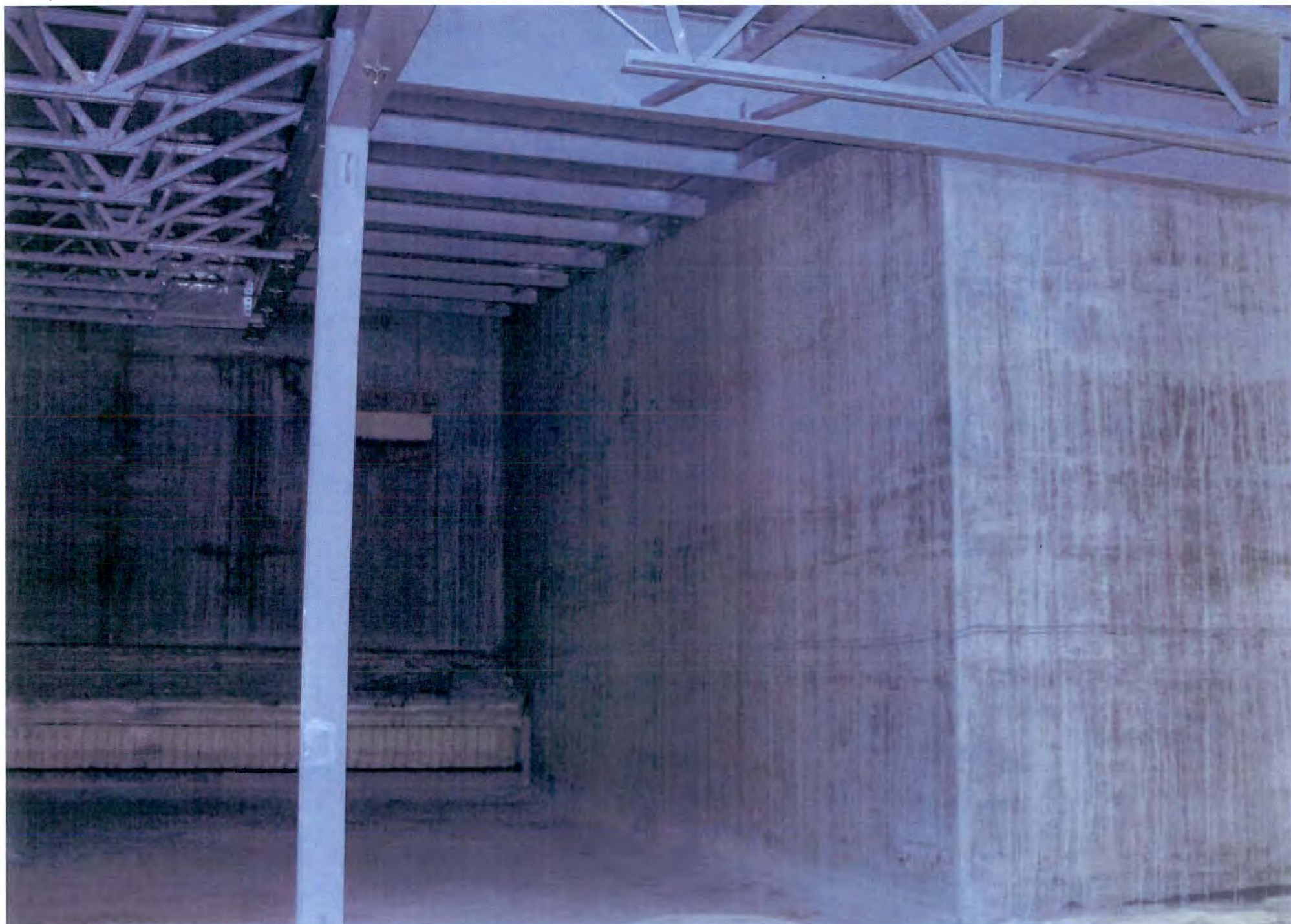
PHOTO # 111/109N/Area Under SSE Roof-W.Side of Press./El.40'/02-07-2012
