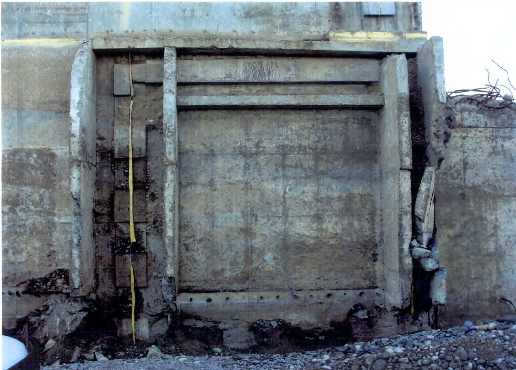
PHOTO # 147/109N W.Wall Below Grade S.End/EI.Varies/07-10-2012
