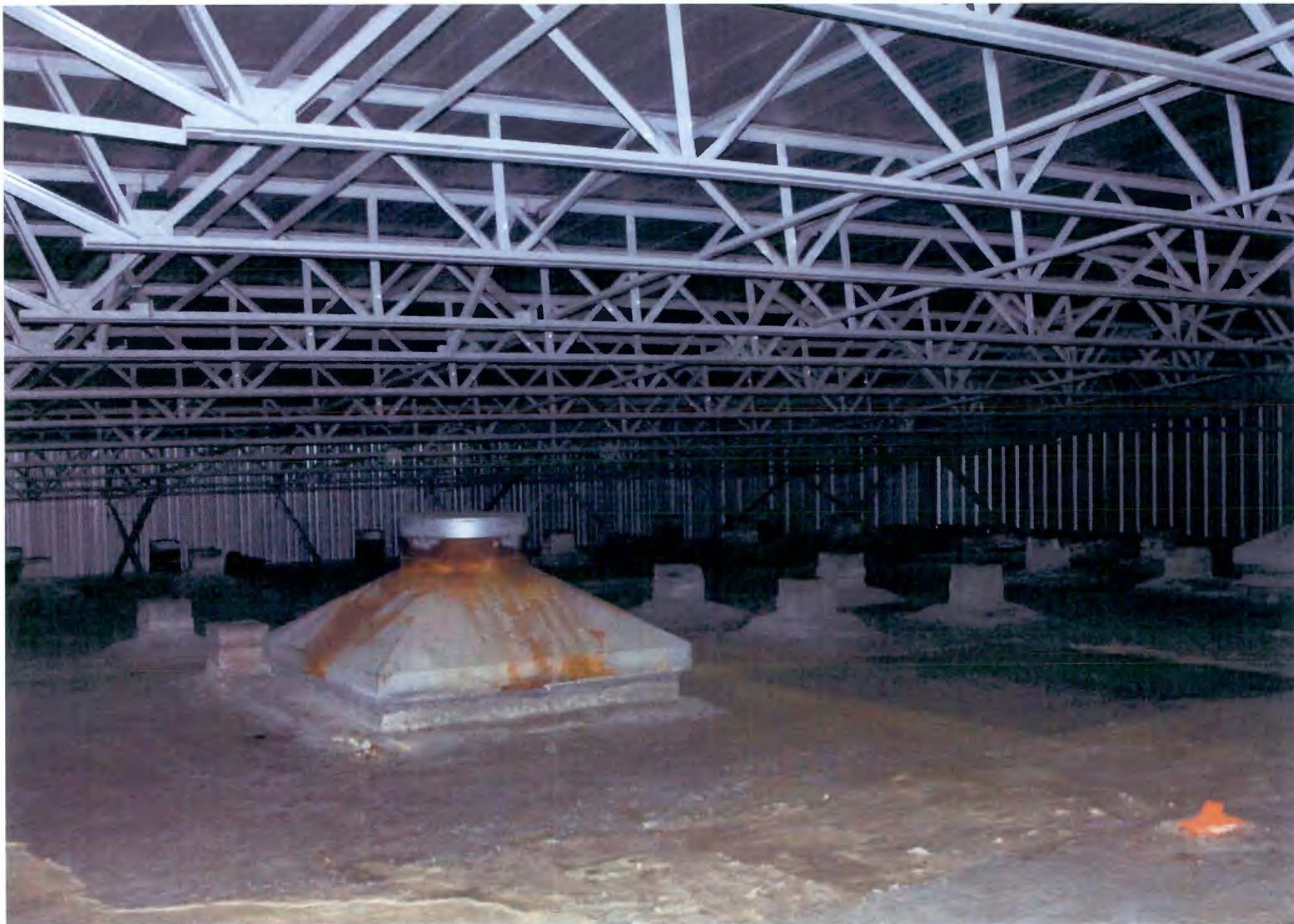
PHOTO # 116/109N/Area Under SSE Roof-S.Wall W.End/EI.40'/02-07-2012
