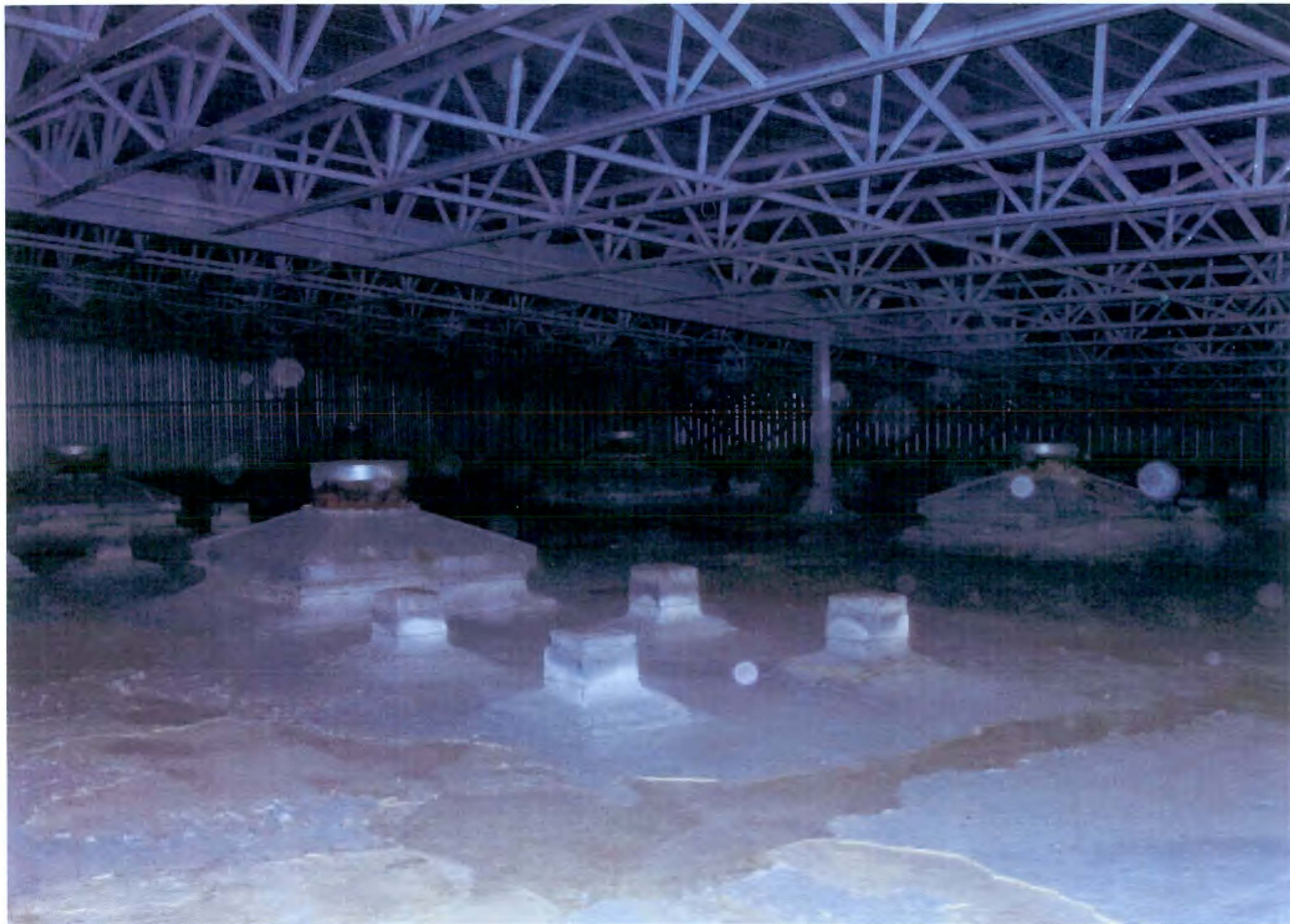
PHOTO # 106/109N/Area Under SSE Roof-SW Corner/EI.40'/02-07-2012
