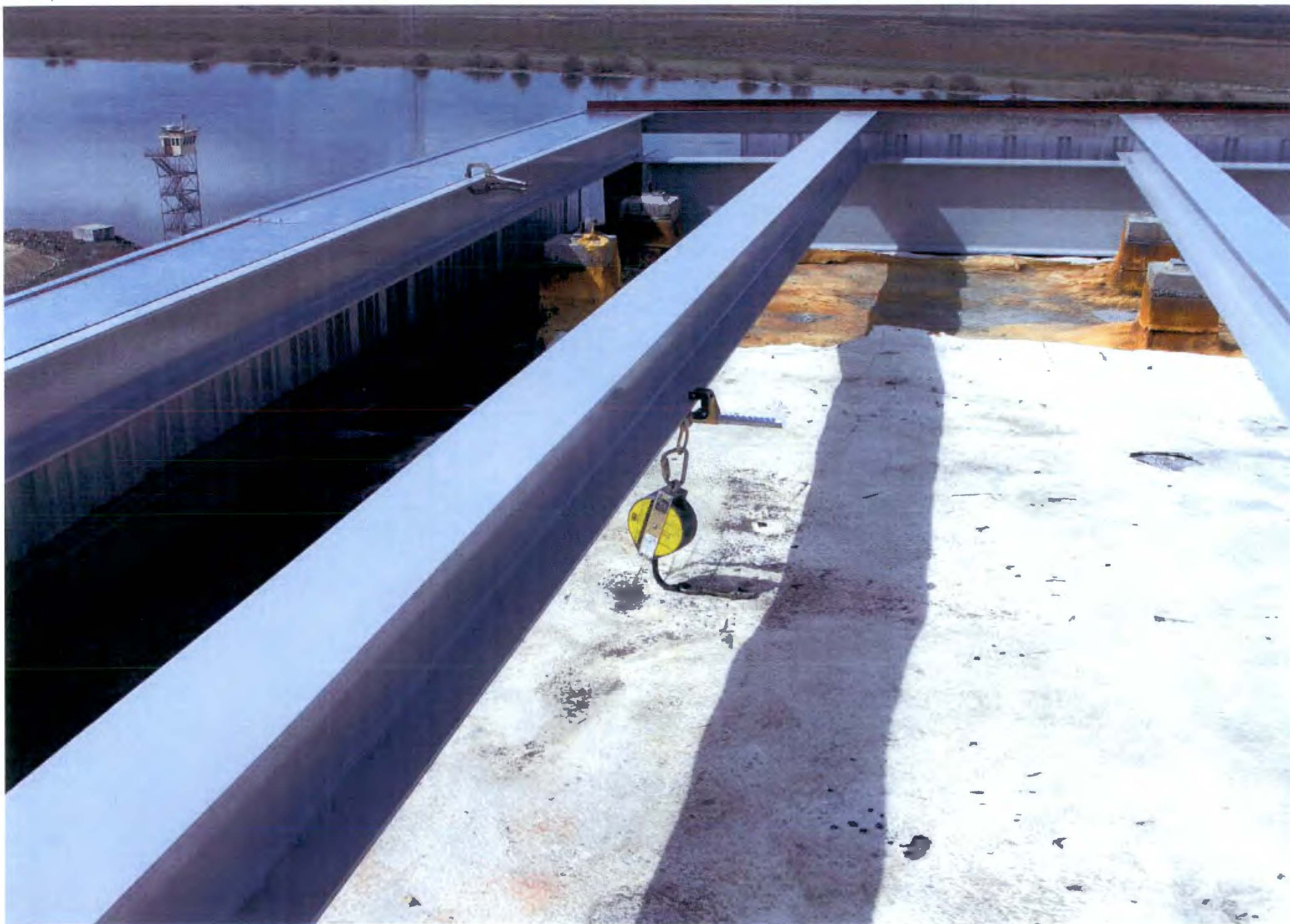
PHOTO # 132/109N Pressurizer/SSE Roof-South Side/04-06-2011
