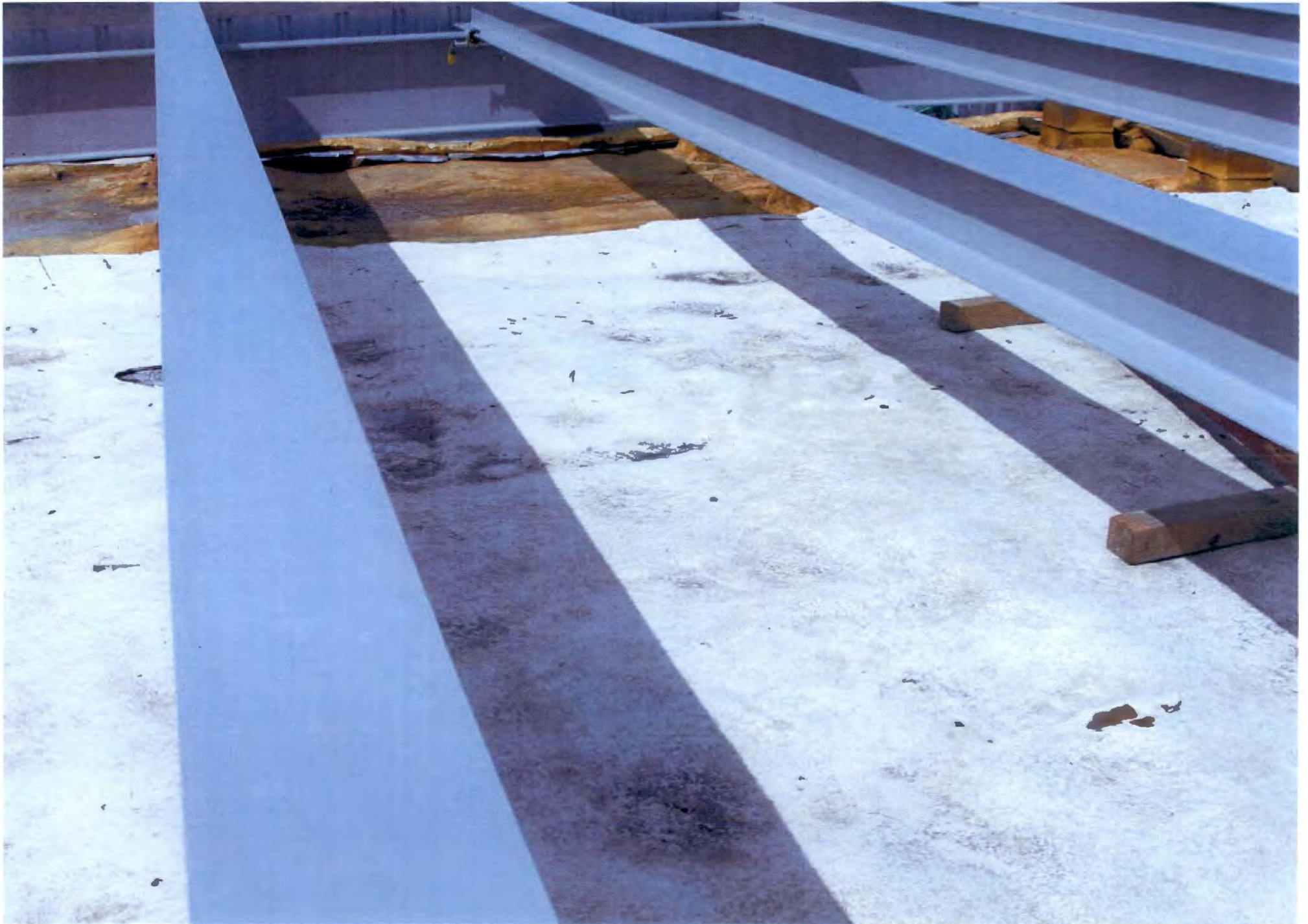
PHOTO # 136/109N Pressurizer/Top of Roof/04-06-2011
