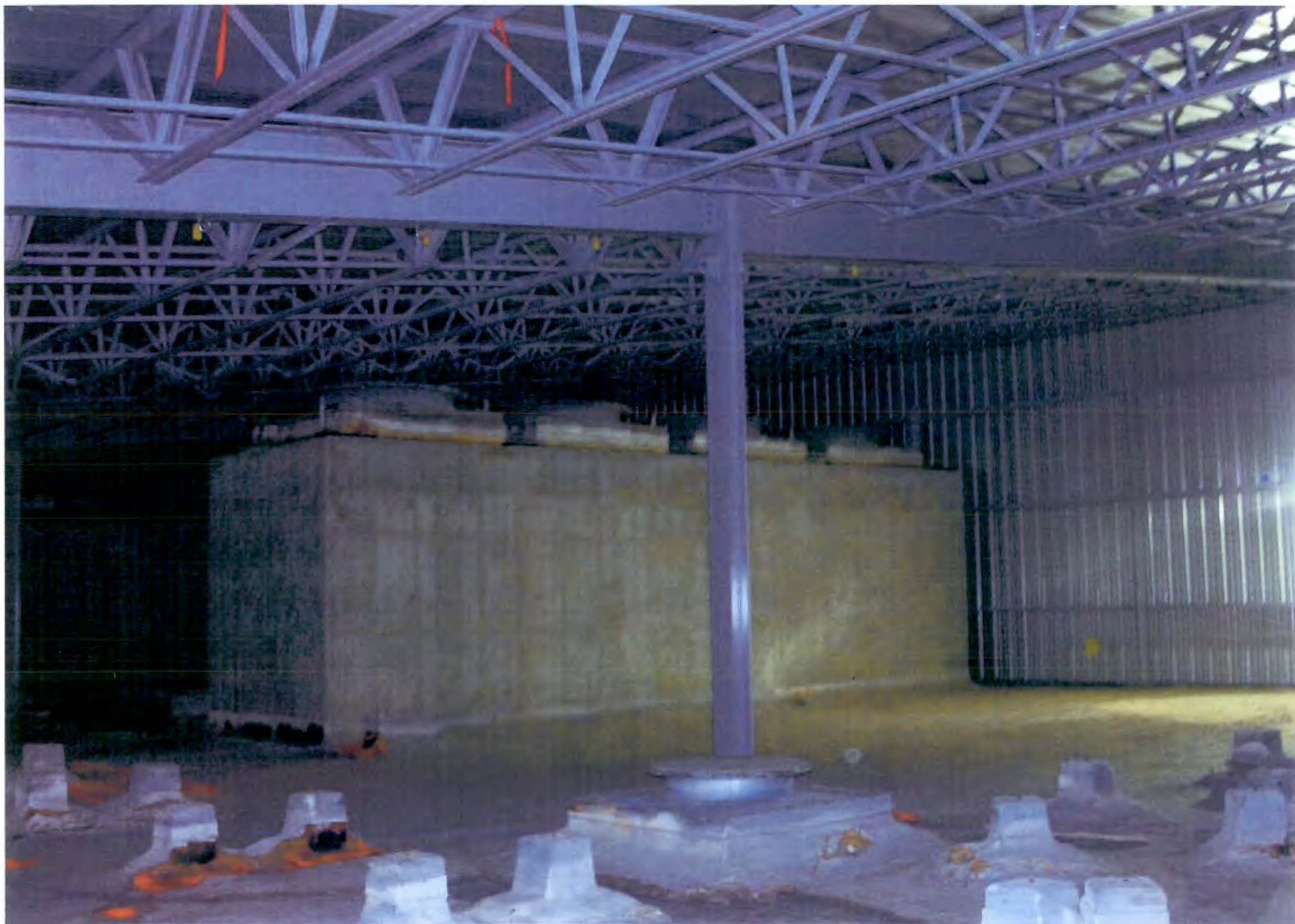
PHOTO # 113/109N/Area Under SSE Roof-Ctr.Vent Valve Struct./El.40'/02-07-2012
