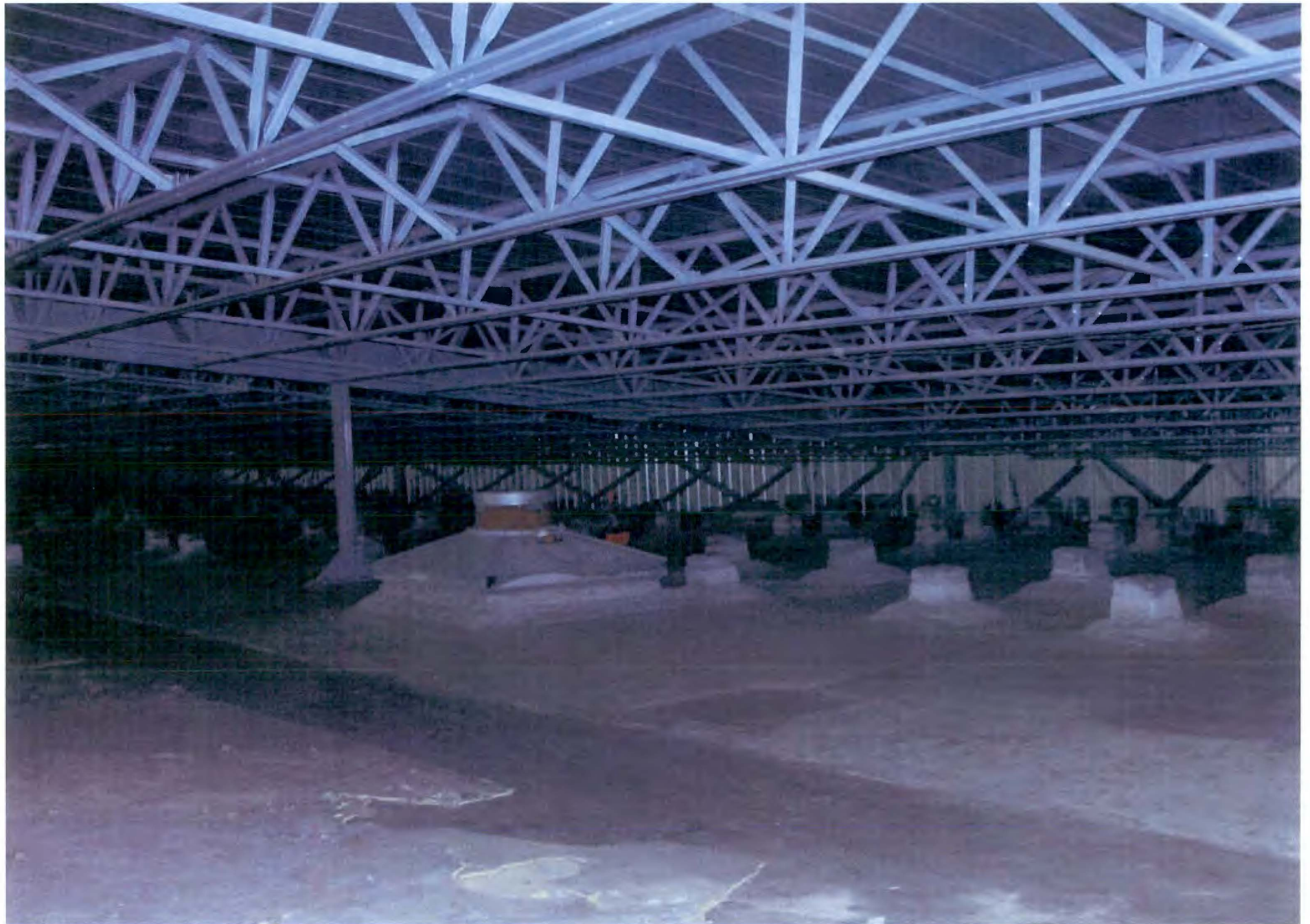
PHOTO # 117/109N/Area Under SSE Roof-South Wall Ctr./El.40'/02-07-2012
