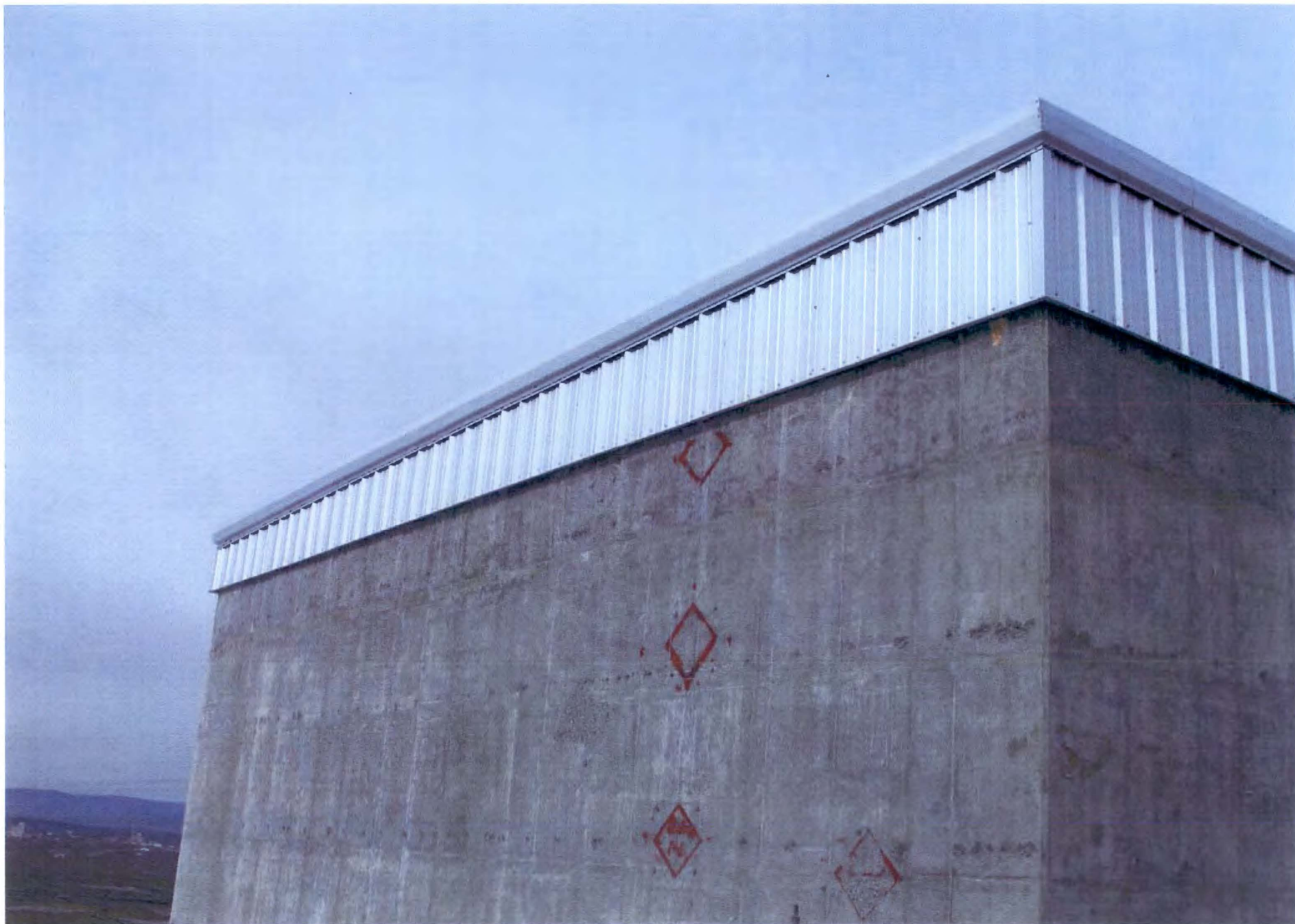
PHOTO # 137/109N Pressurizer/SSE-Roof East Side/04-20-2011
