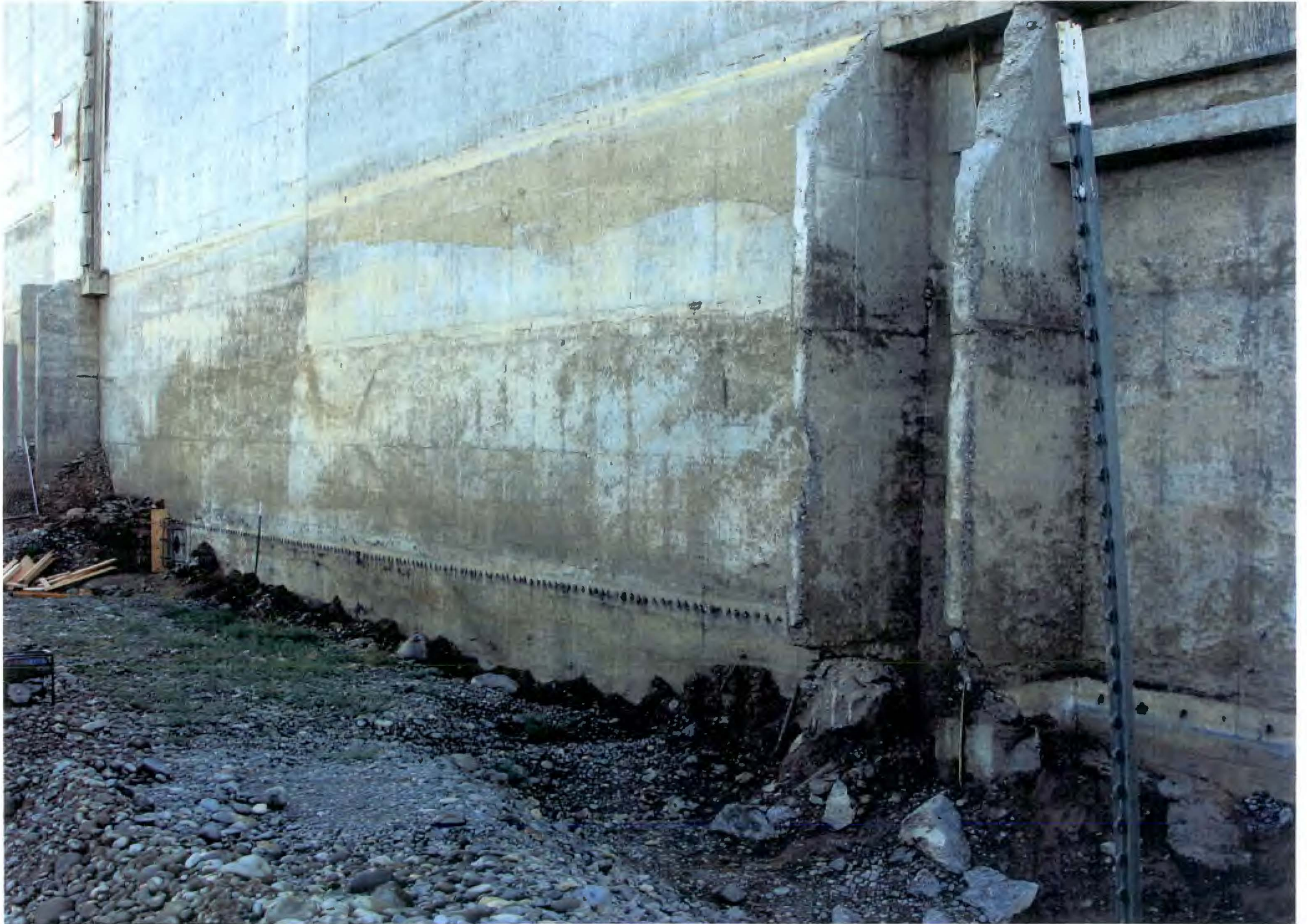
PHOTO # 144/109N W.Wall Below Grade Looking North/EI.Varies/07-10-2012
