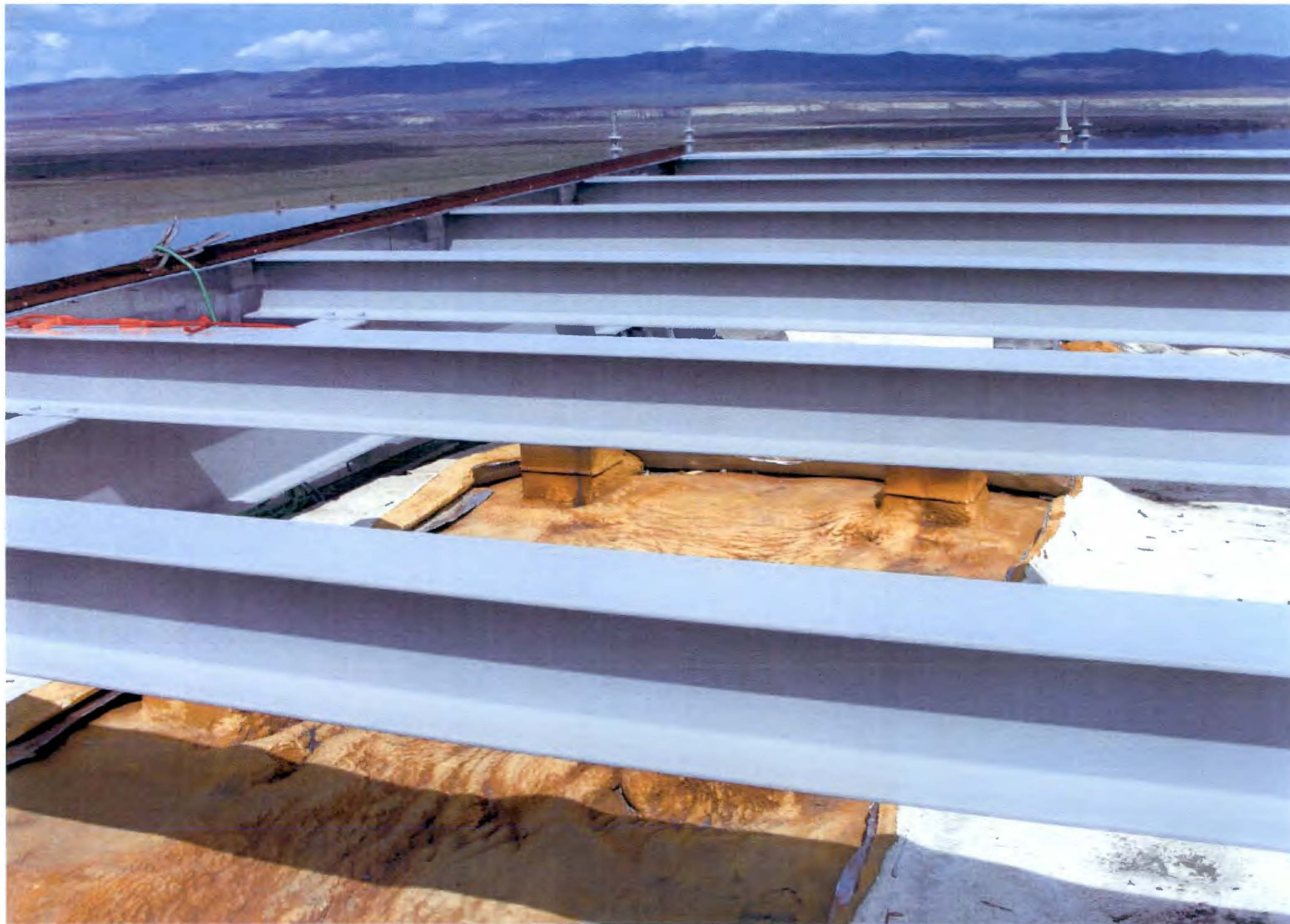
PHOTO # 134/109N Pressurizer/SSE Roof Looking NW/04-06-2011
