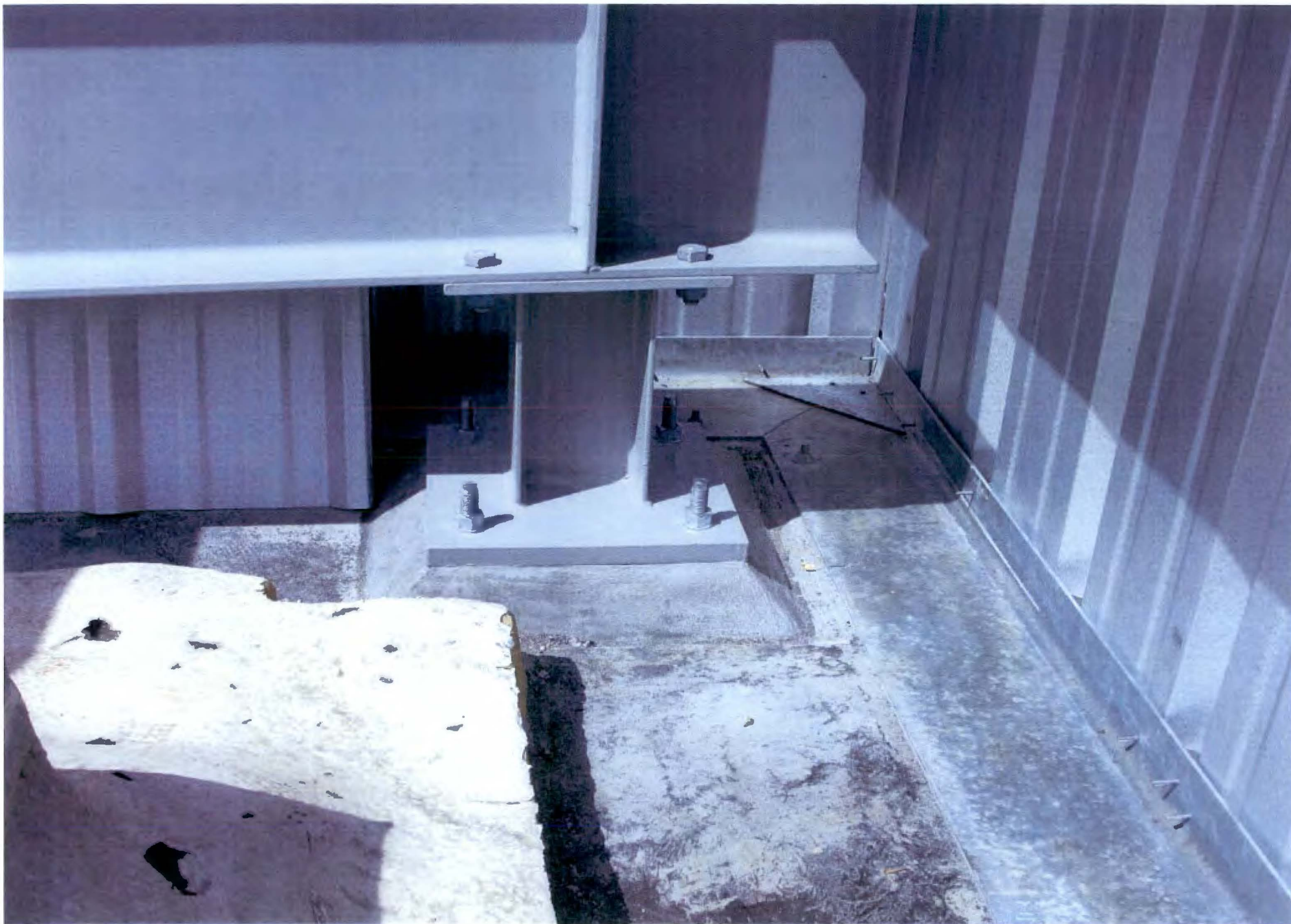
PHOTO # 128/109N Pressurizer/SSE Roof-NW Corner/04-06-2011
