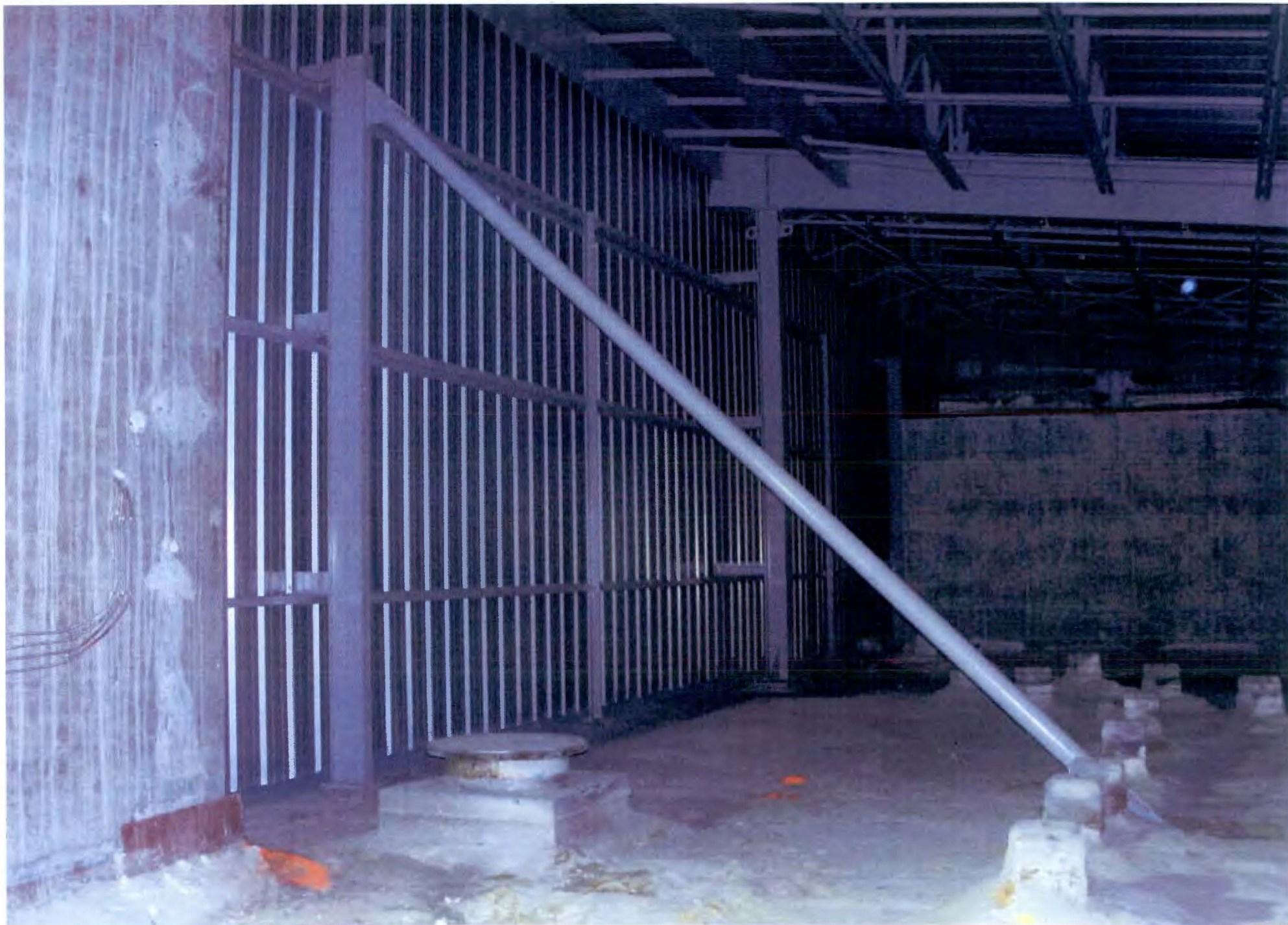
PHOTO # 103/109N/Area Under SSE Roof-North Wall East End/EI.40'/02-07-2012
