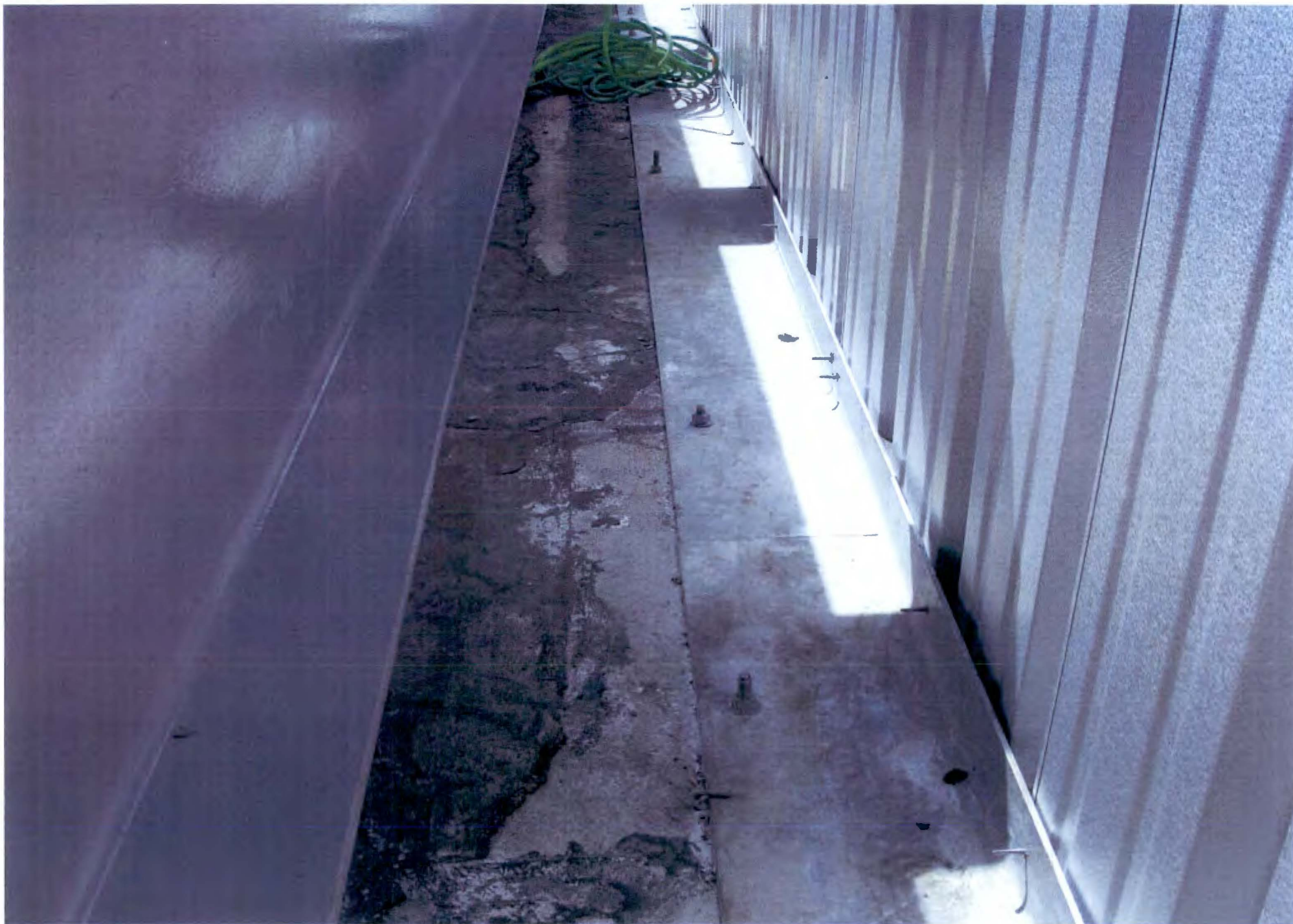
PHOTO # 129/109N Pressurizer/SSE Roof-West Side/04-06-2011
