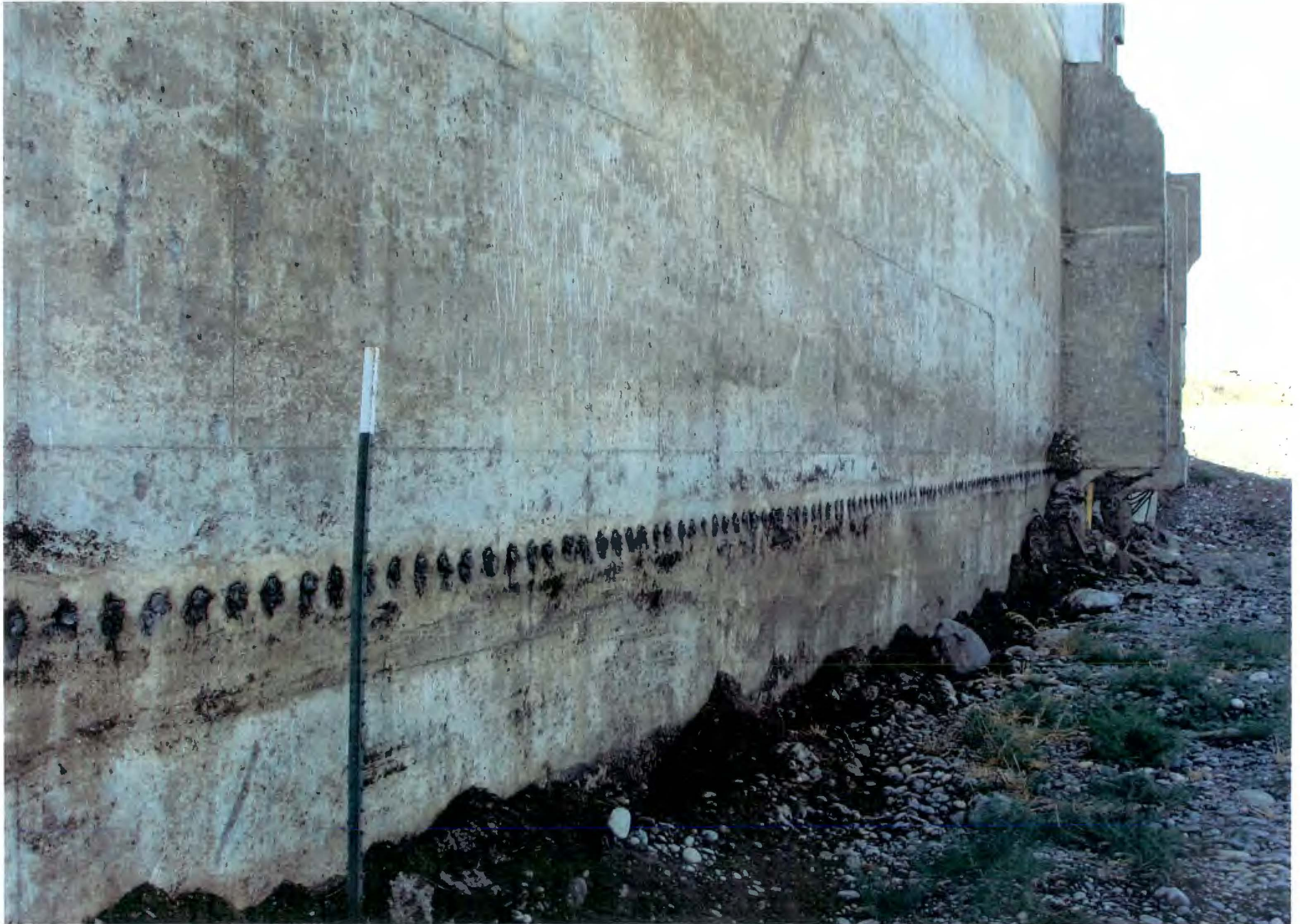
PHOTO # 146/109N W.Wall Below Grade Looking South/EI.Varies/07-10-2012
