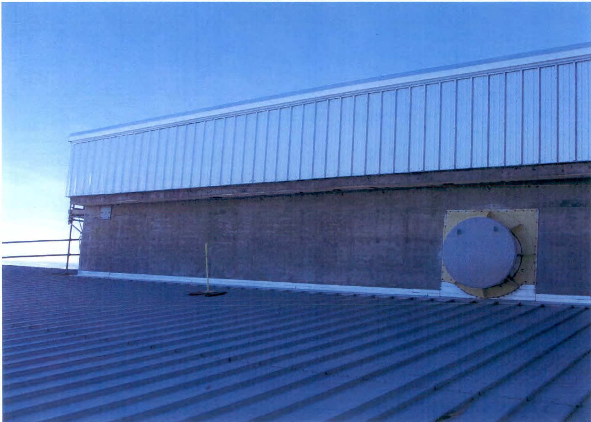
PHOTO # 118/109N/SSE Roof-Tie-In to S.Side 105N/09-21-2011
