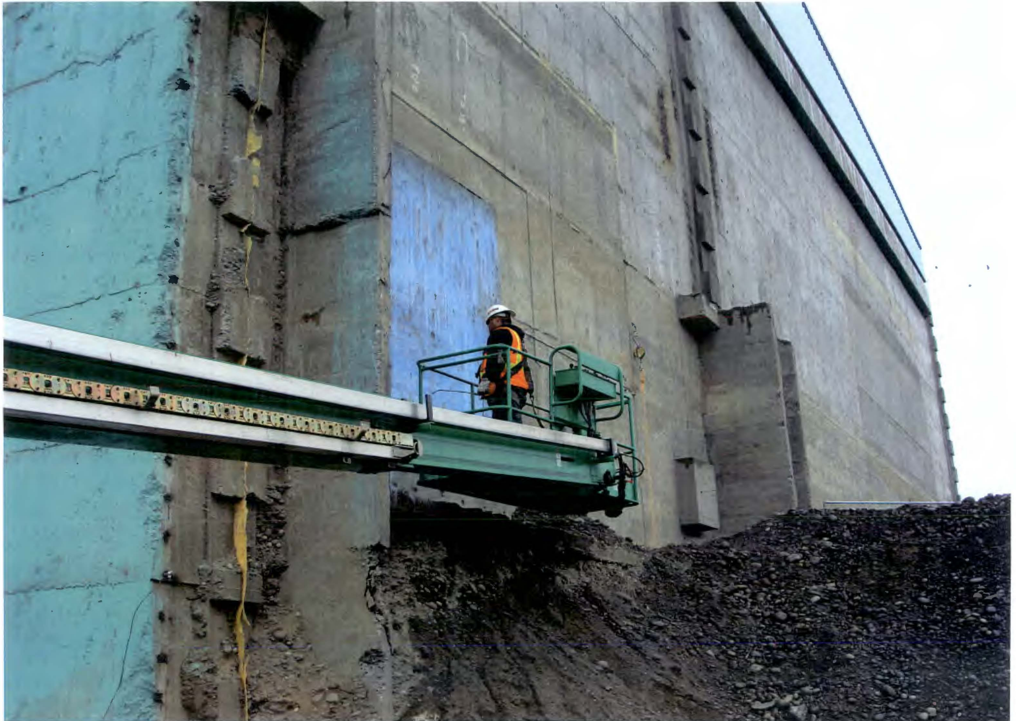
PHOTO # 143/109N W.Wall N.End Pourbacks/El.Varies/06-26-2012
