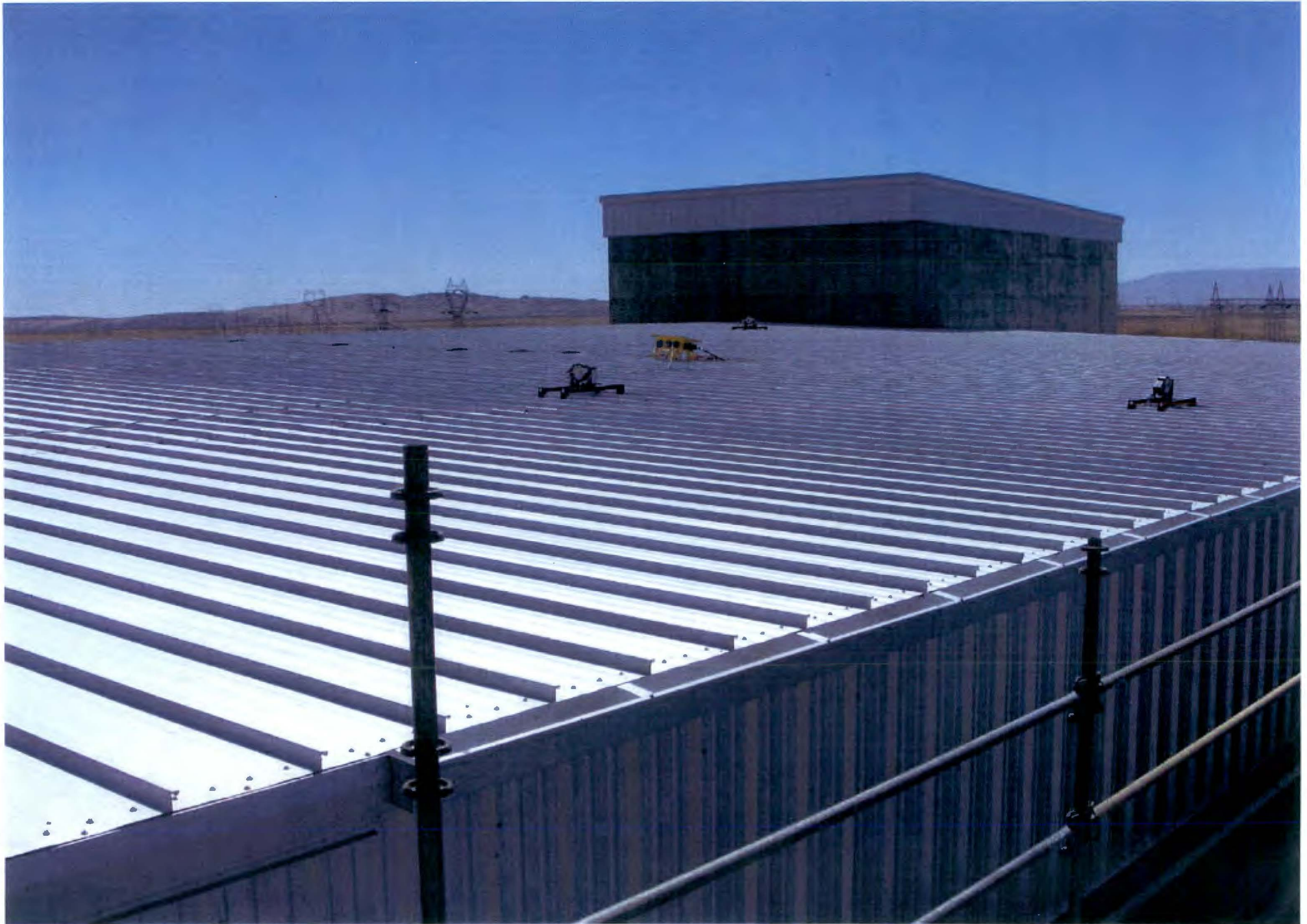
PHOTO # 142/109N Pressurizer/SSE Roof-NW Side/08-18-2011
