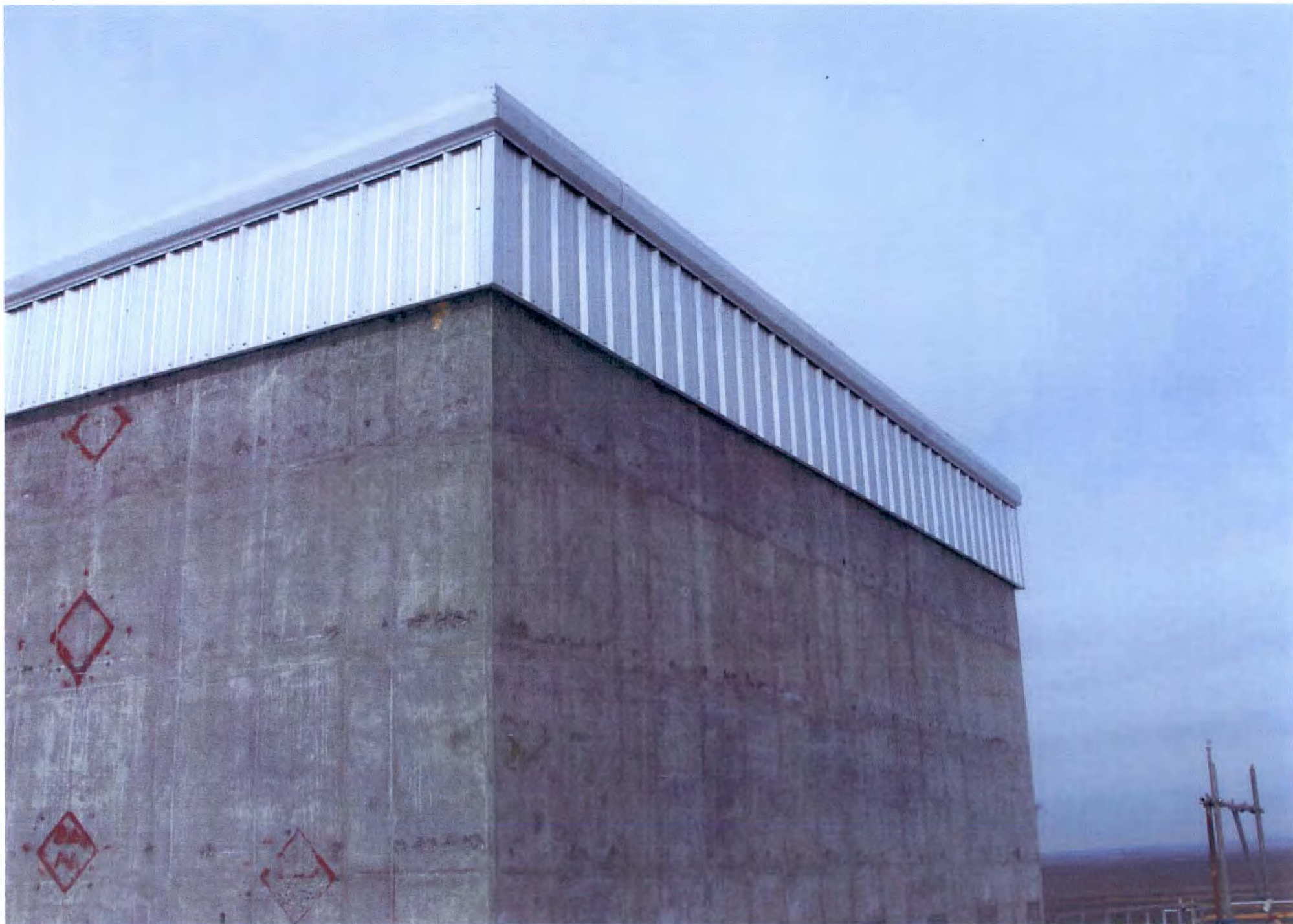
PHOTO # 138/109N Pressurizer/SSE Roof-North Side/04-20-2011
