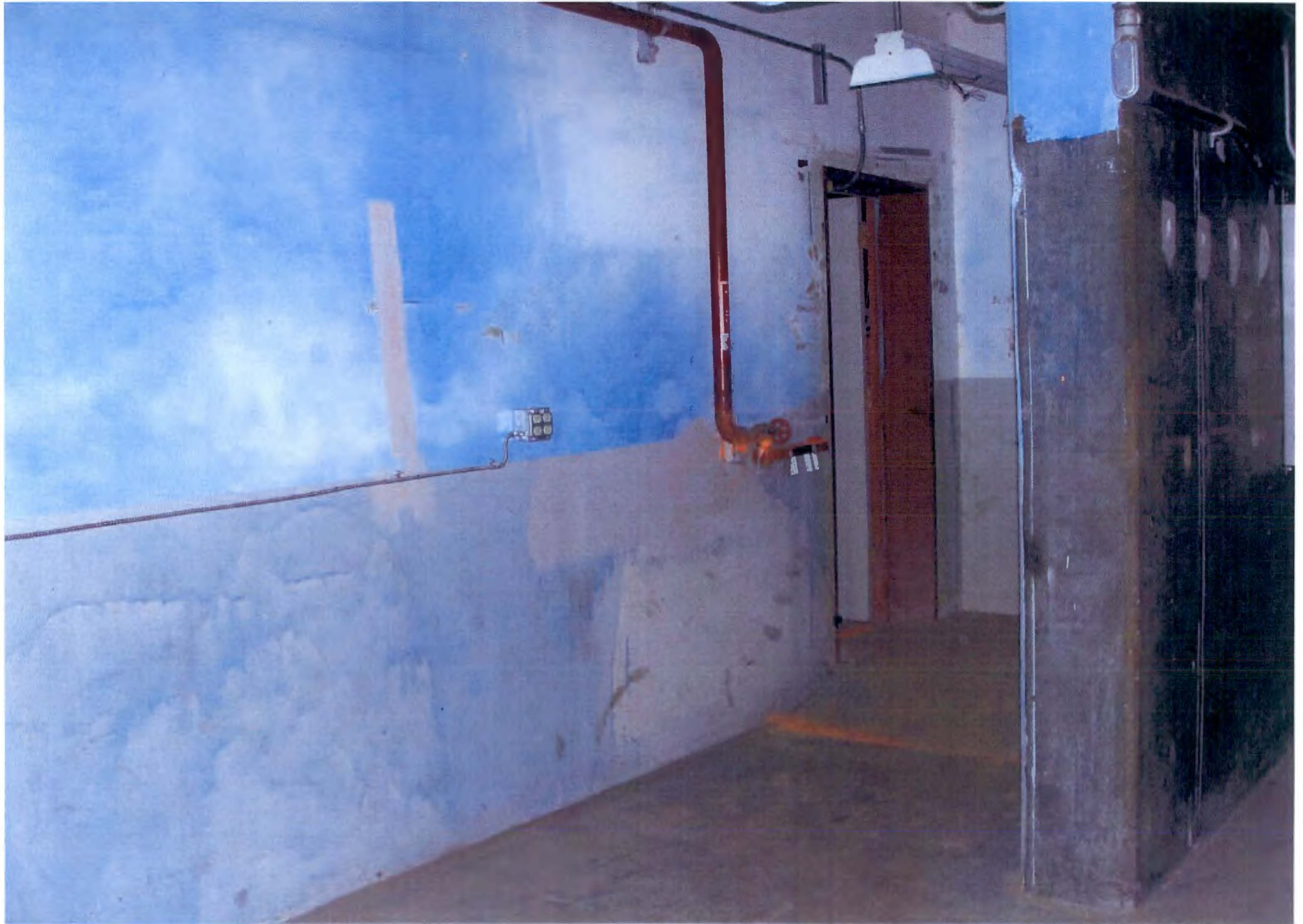
PHOTO # 101/109N/Area Below SSE Roof-Access Door/EI.40'/02-07-2012
