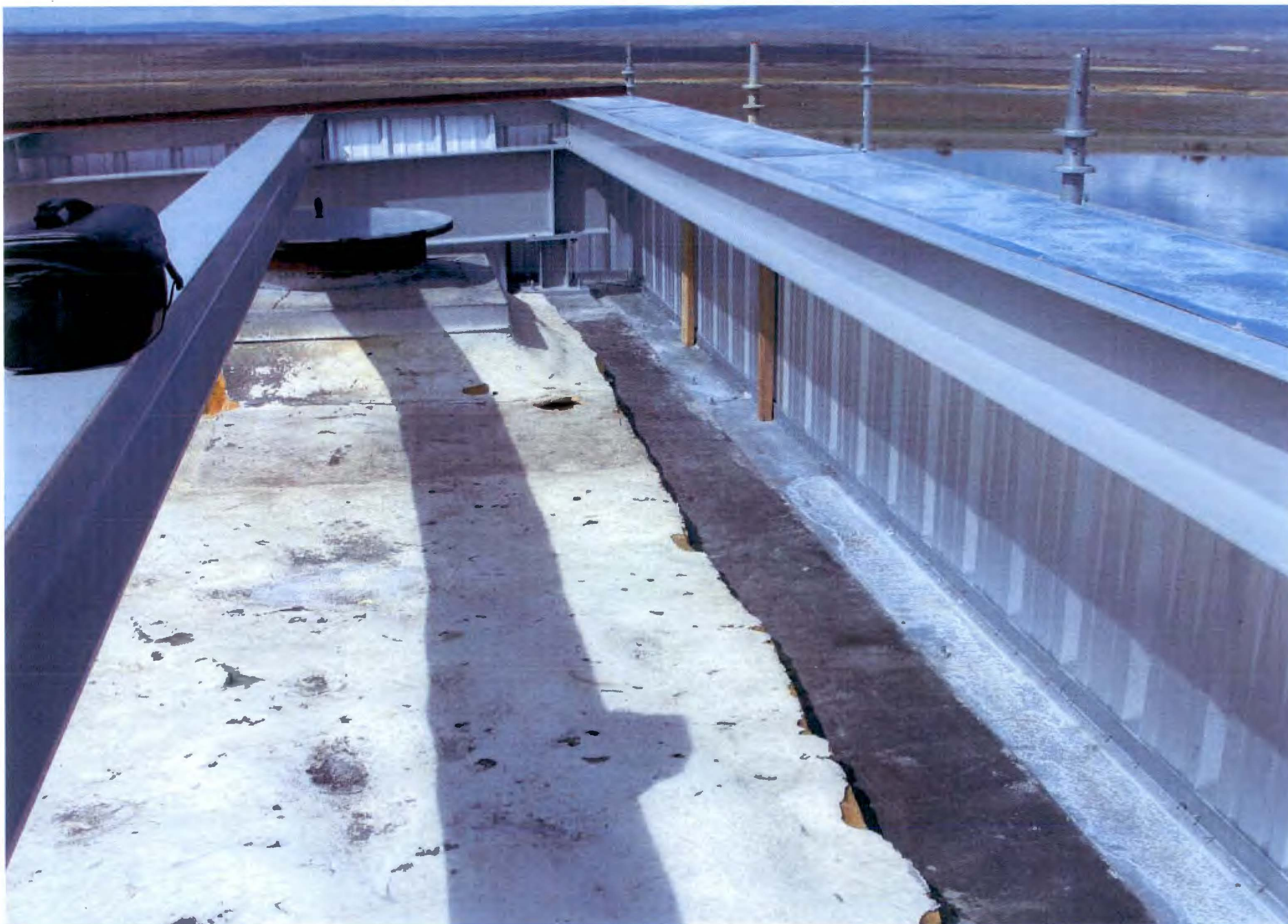
PHOTO # 121/109N Pressurizer/SSE Roof NW Corner/04-06-2011
