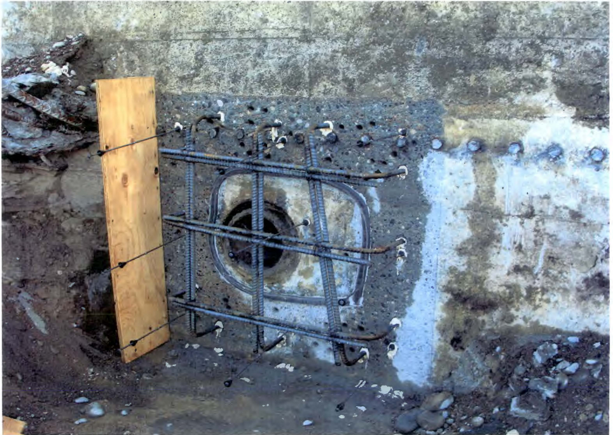
PHOTO # 145/109N W.Wall Below Grade Pourback (10" BD Line)/El.Varies/07-10-2012
