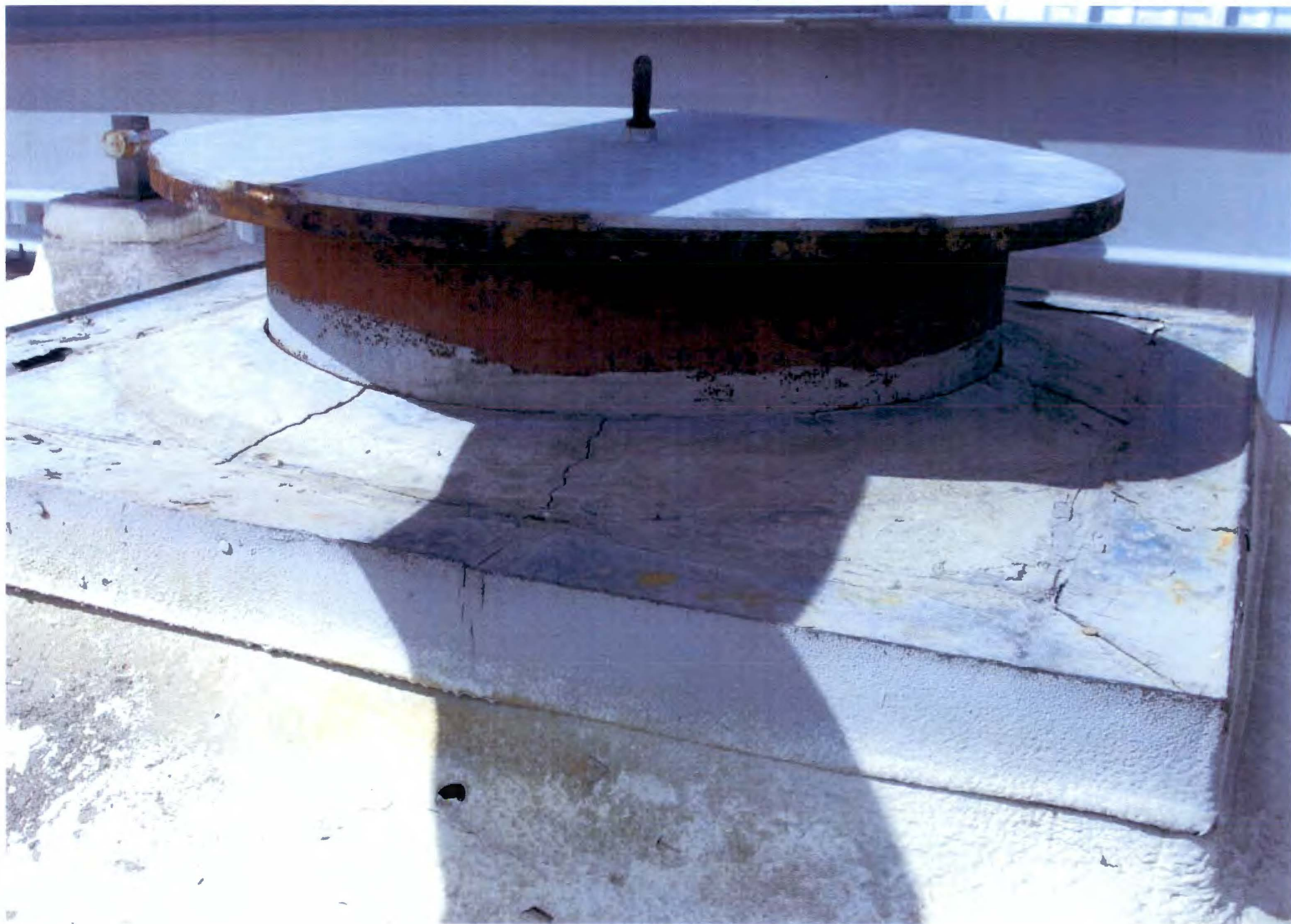
PHOTO # 126/109N Pressurizer/SSE Roof-Cover Plate/04-06-2011
