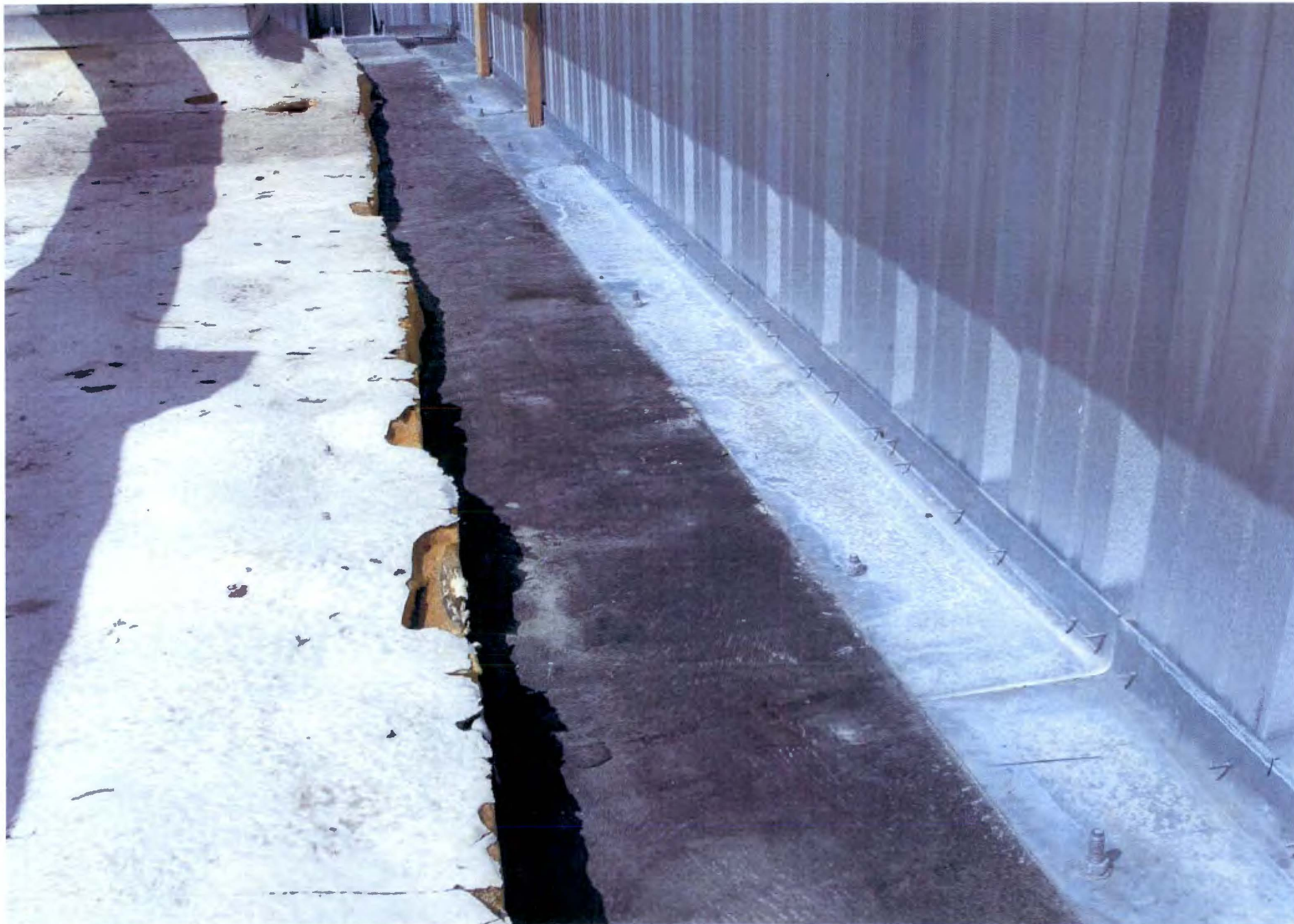
PHOTO # 127/109N Pressurizer/SSE Roof North Side/04-06-2011
