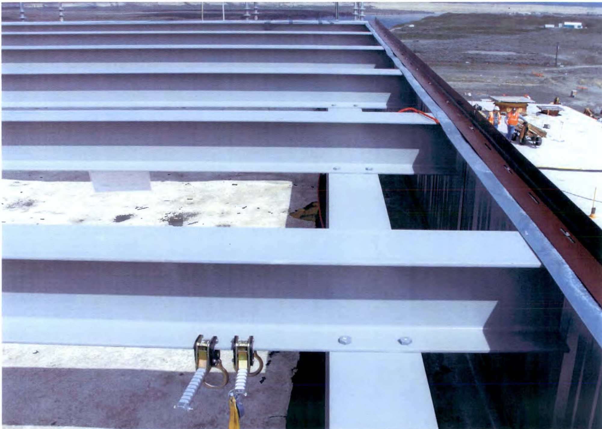
PHOTO # 135/109N Pressurizer/SSE Roof Looking North/04-06-2011
