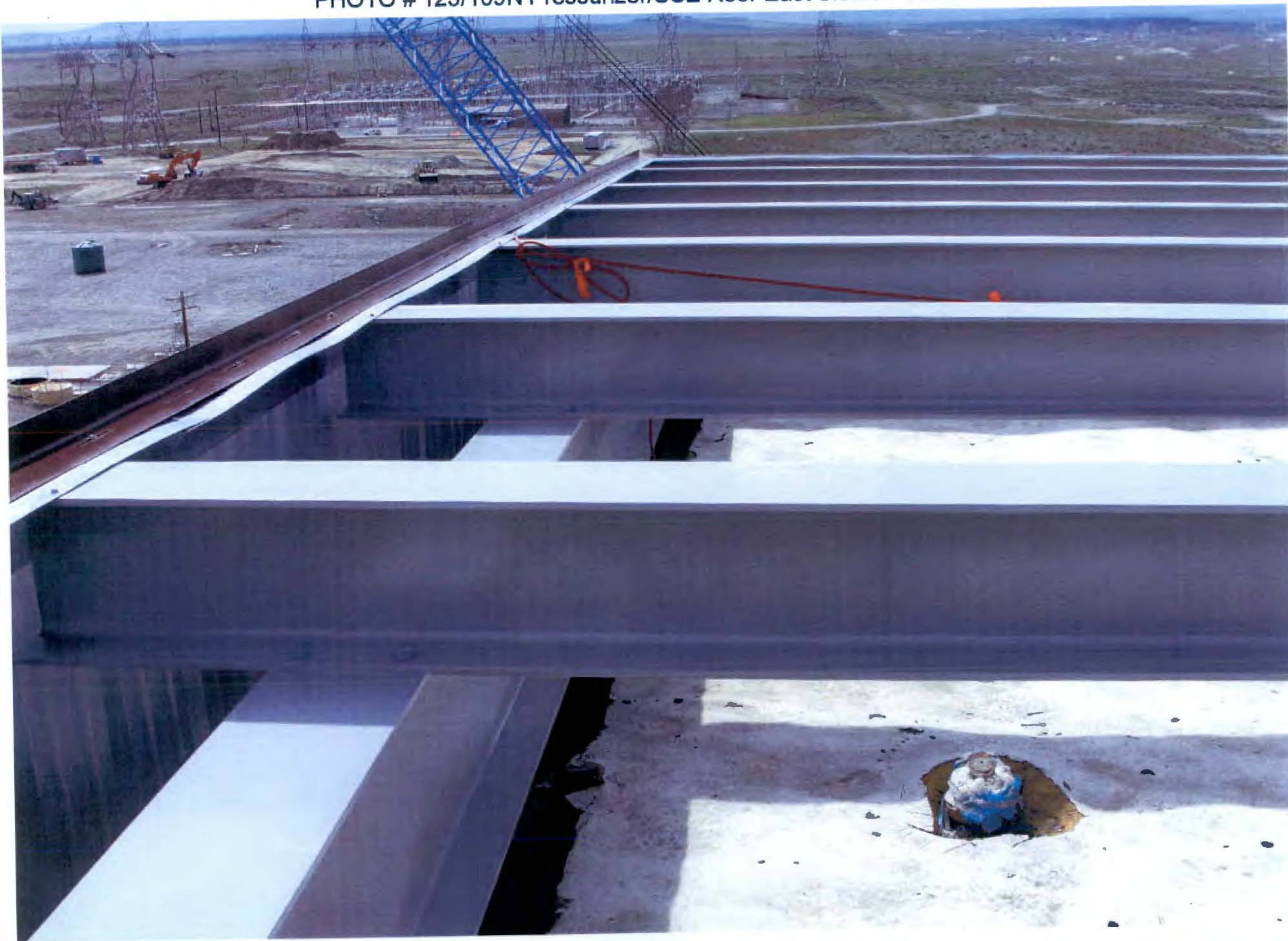
PHOTO # 123/109N Pressurizer/SSE Roof-East Side/04-06-2011
