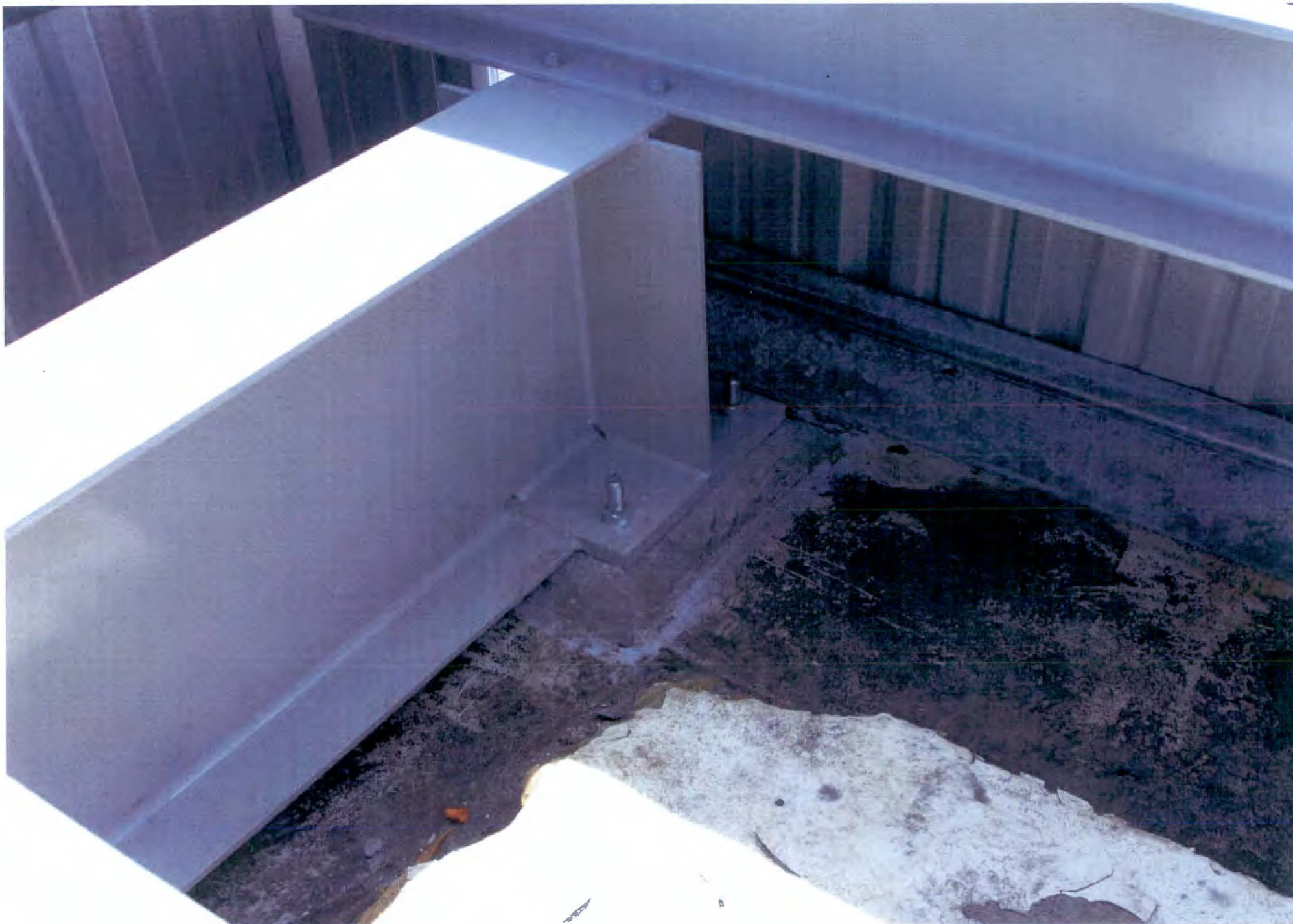
PHOTO # 130/109N Pressurizer/SSE Roof-SE Corner/04-06-2011
