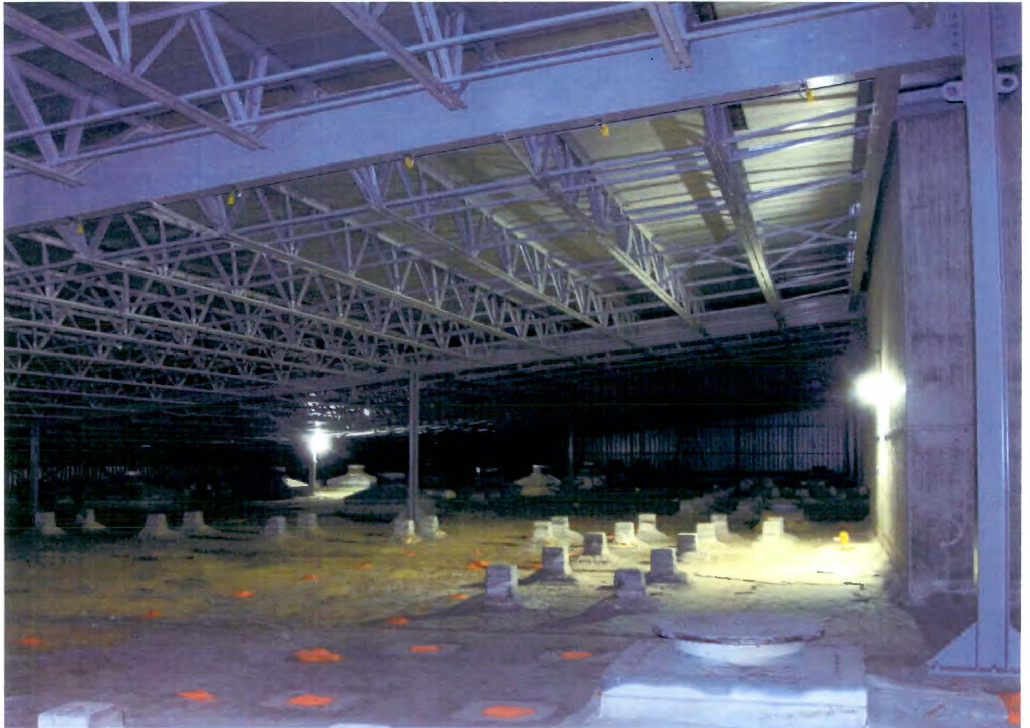
PHOTO # 110/109N/Area Under SSE Roof-West ½ Roof/EI.40'/02-07-2012
