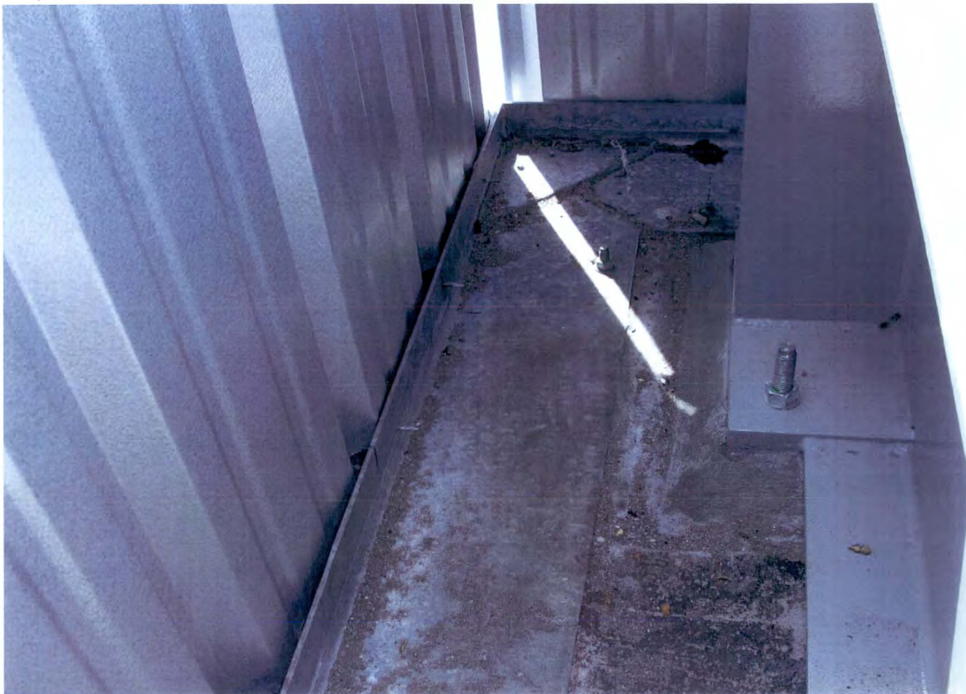
PHOTO # 131/109N Pressurizer/SSE Roof-SE Corner/04-06-2011
