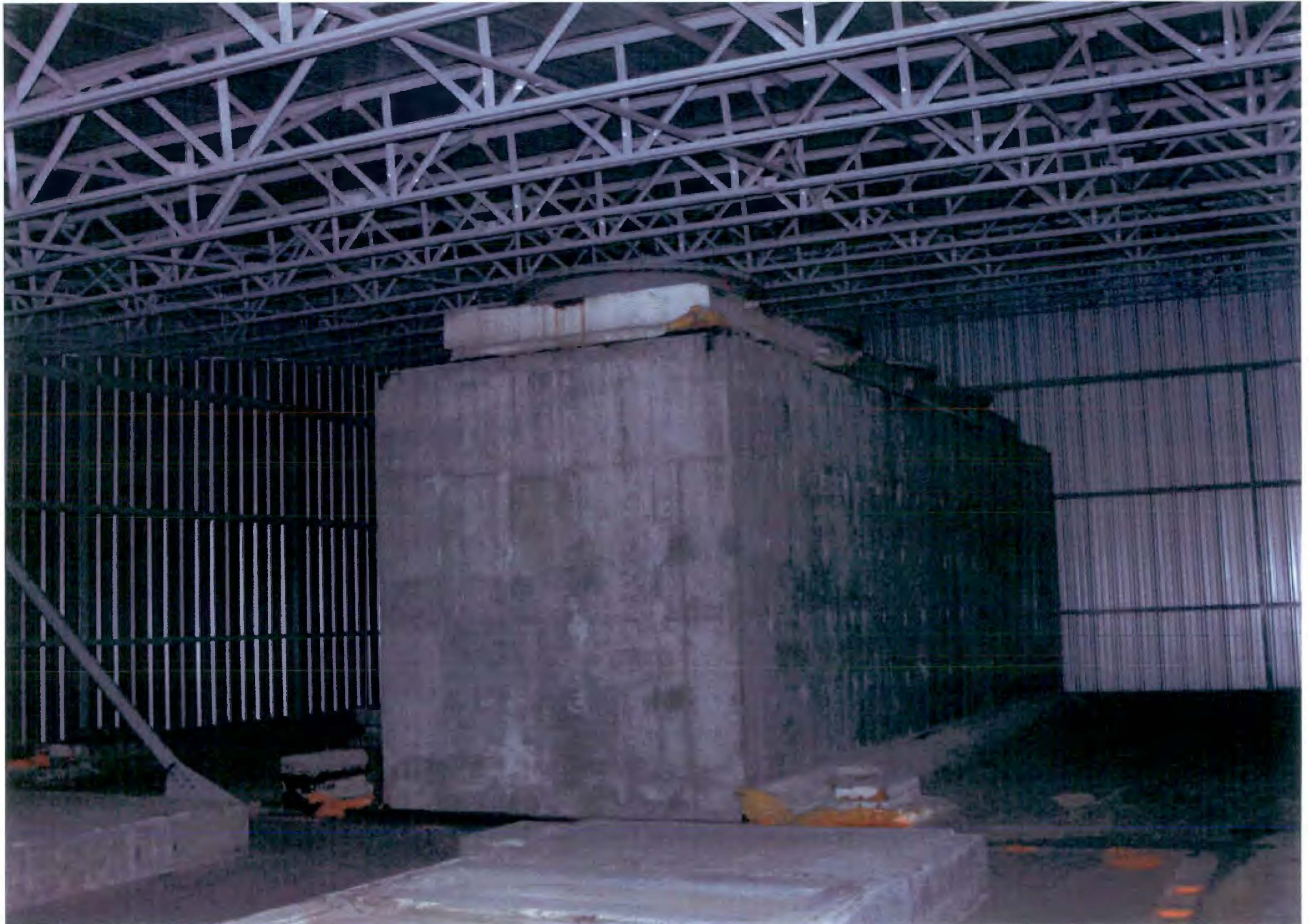
PHOTO # 114/109N/Area Under SSE Roof-W.Vent Valve Struct./El.40'/02-07-2012
