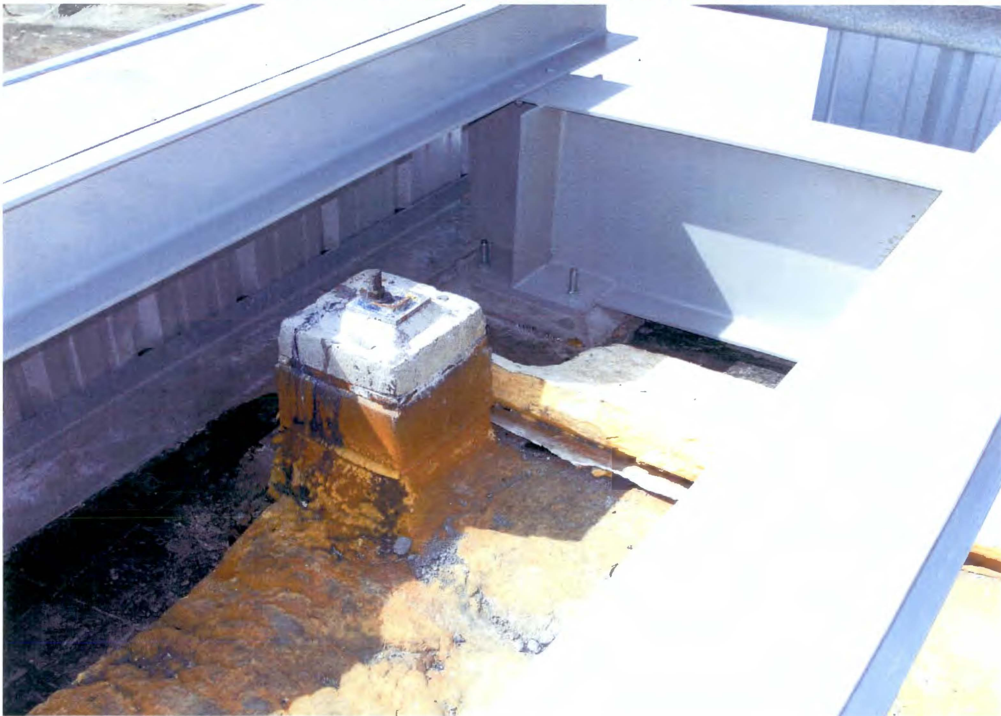
PHOTO # 133/109N Pressurizer/SSE Roof-SW Corner/04-06-2011
