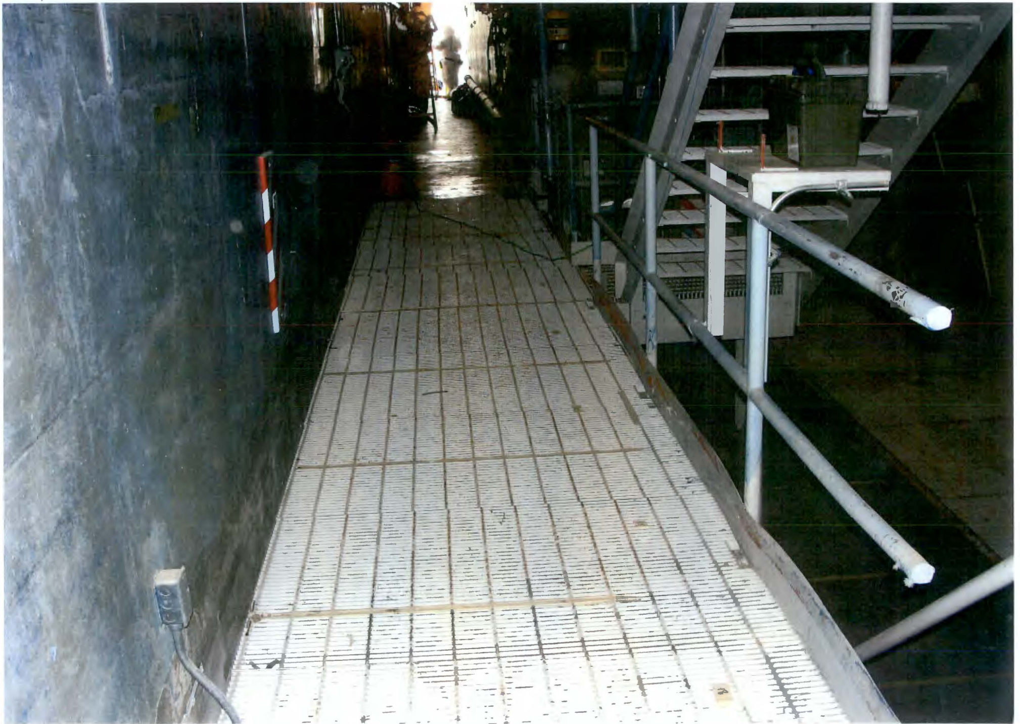
PHOTO # 525/105N/Corridor#7 Center Looking West/EI.+5'-0"/06-05-2012
