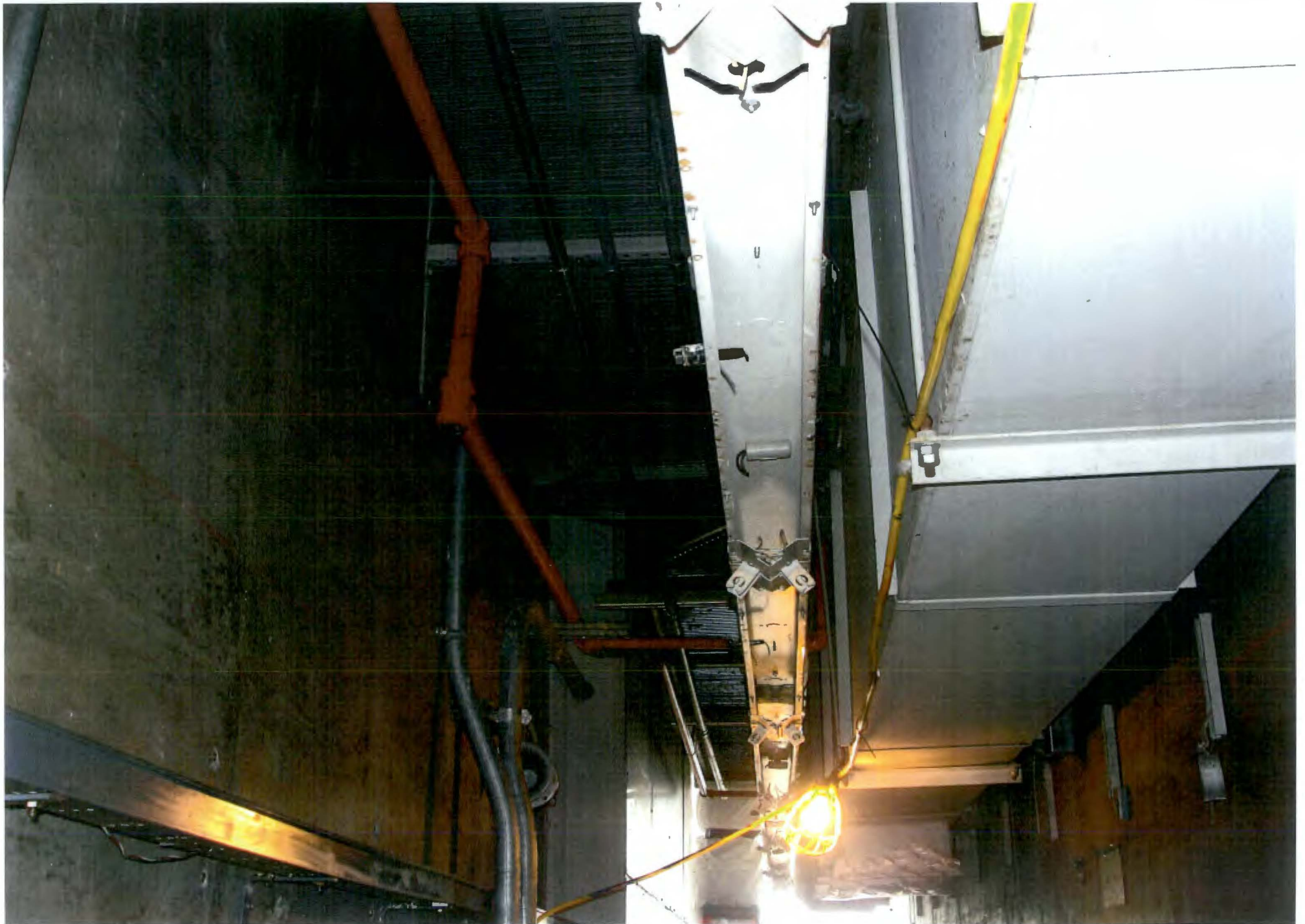
PHOTO # 528/105N/Corridor#7 Ceiling West End/El.+5'-0"/06-05-2012
