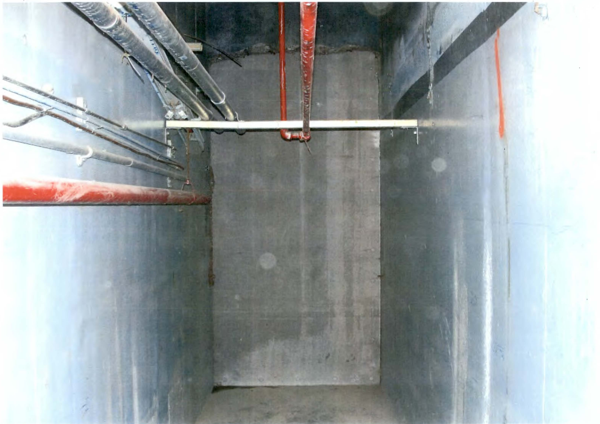
PHOTO # 522/105N/Corridor#7 East End Cover Plate/EI.+5'-0"/06-05-2012
