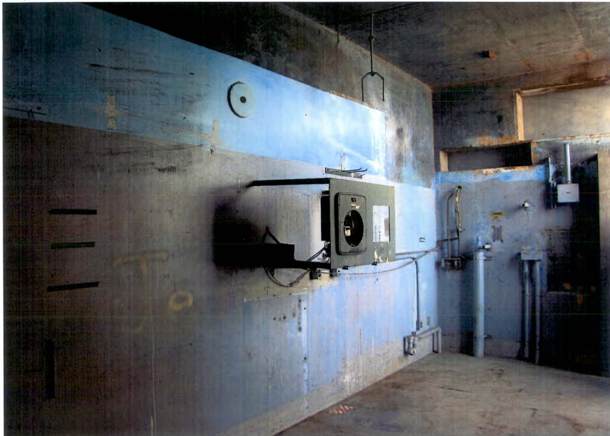
PHOTO # 537/105N/Corridor #22 Looking SE/EI.0'-0"/07-17-2012
