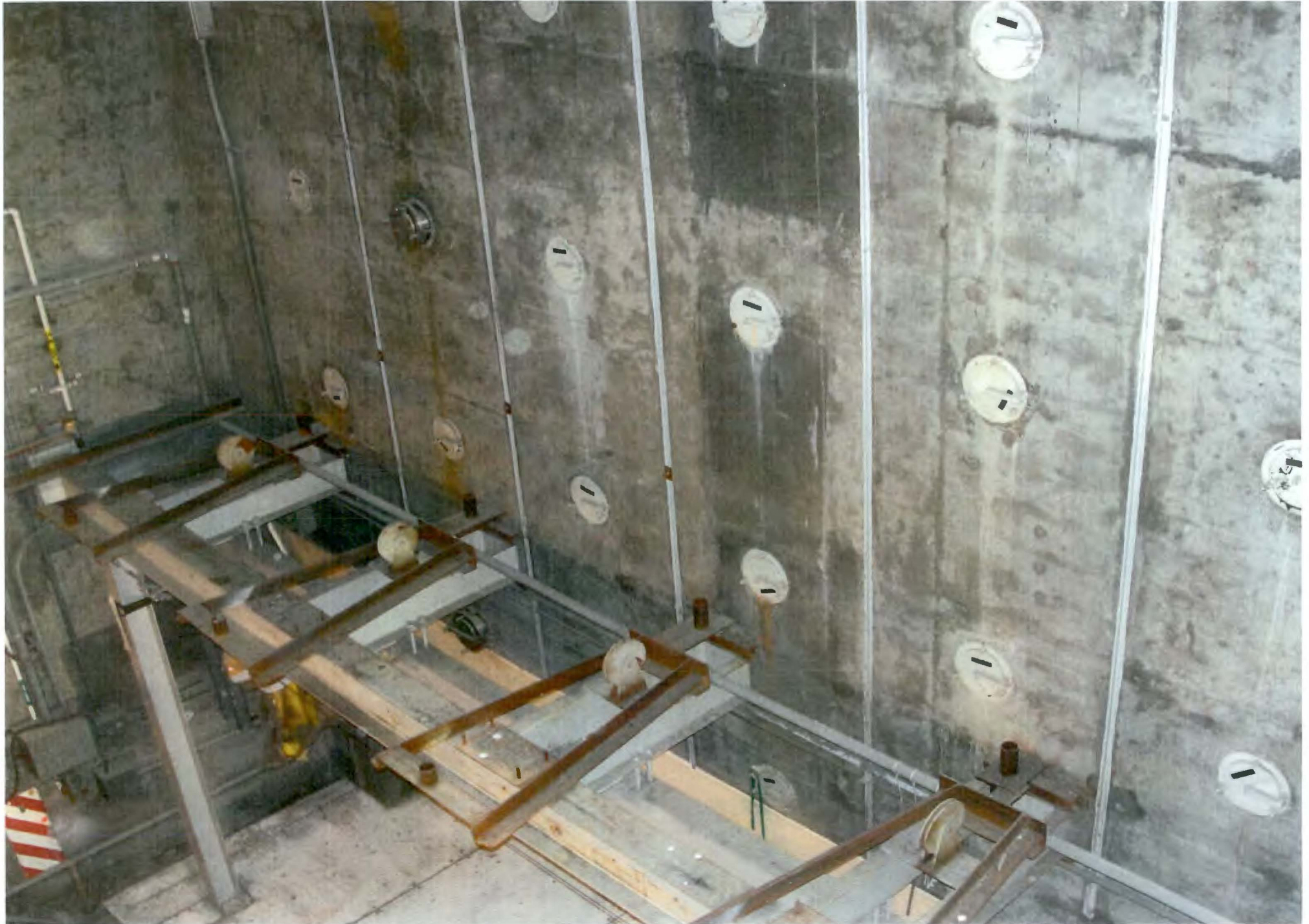
PHOTO # 517/105N/Rm.#175 North Wall/EI.Varies/06-05-2012
