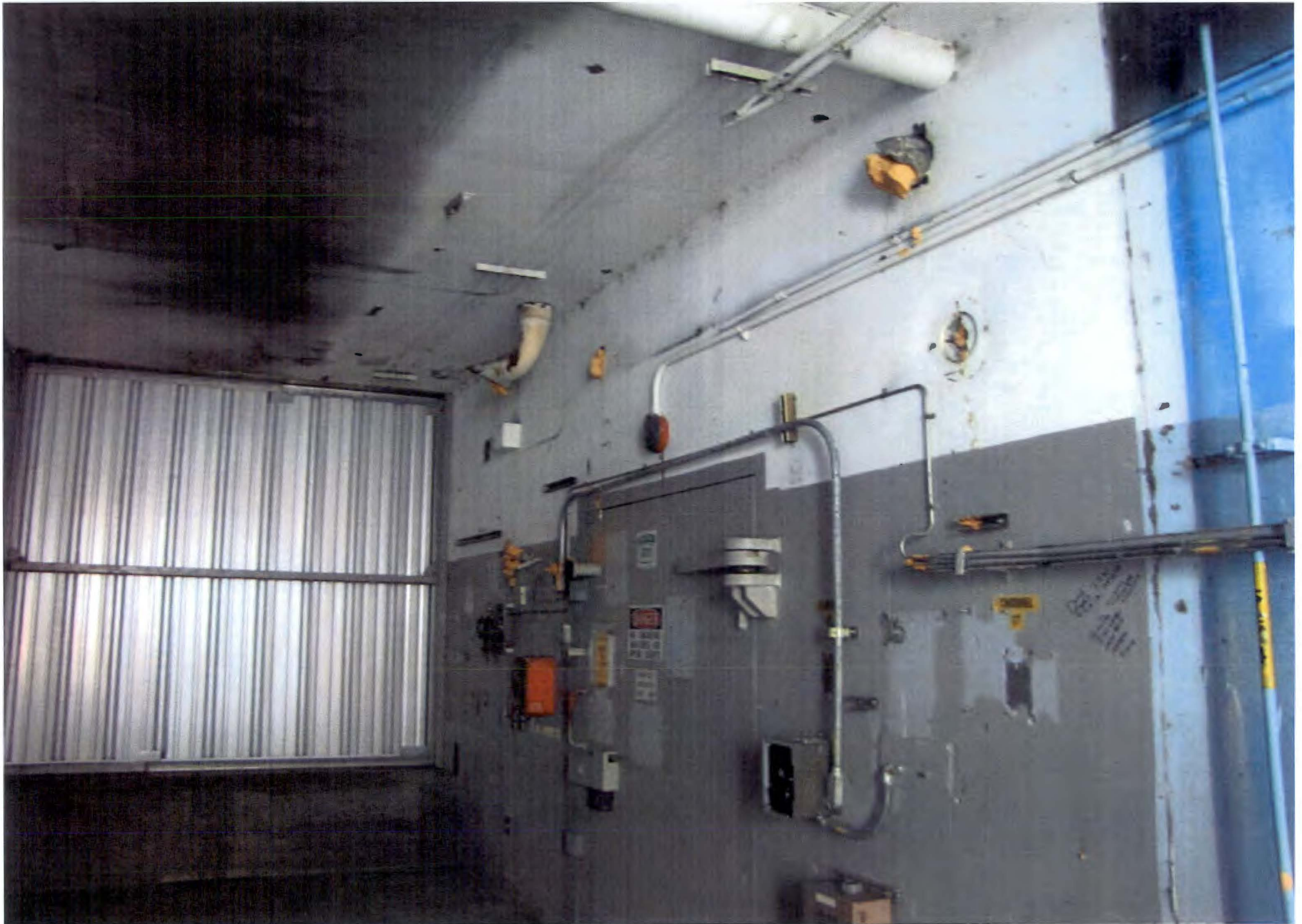
PHOTO # 535/105N/Corridor #22 Looking NE/EI.0'-0"/07-17-2012
