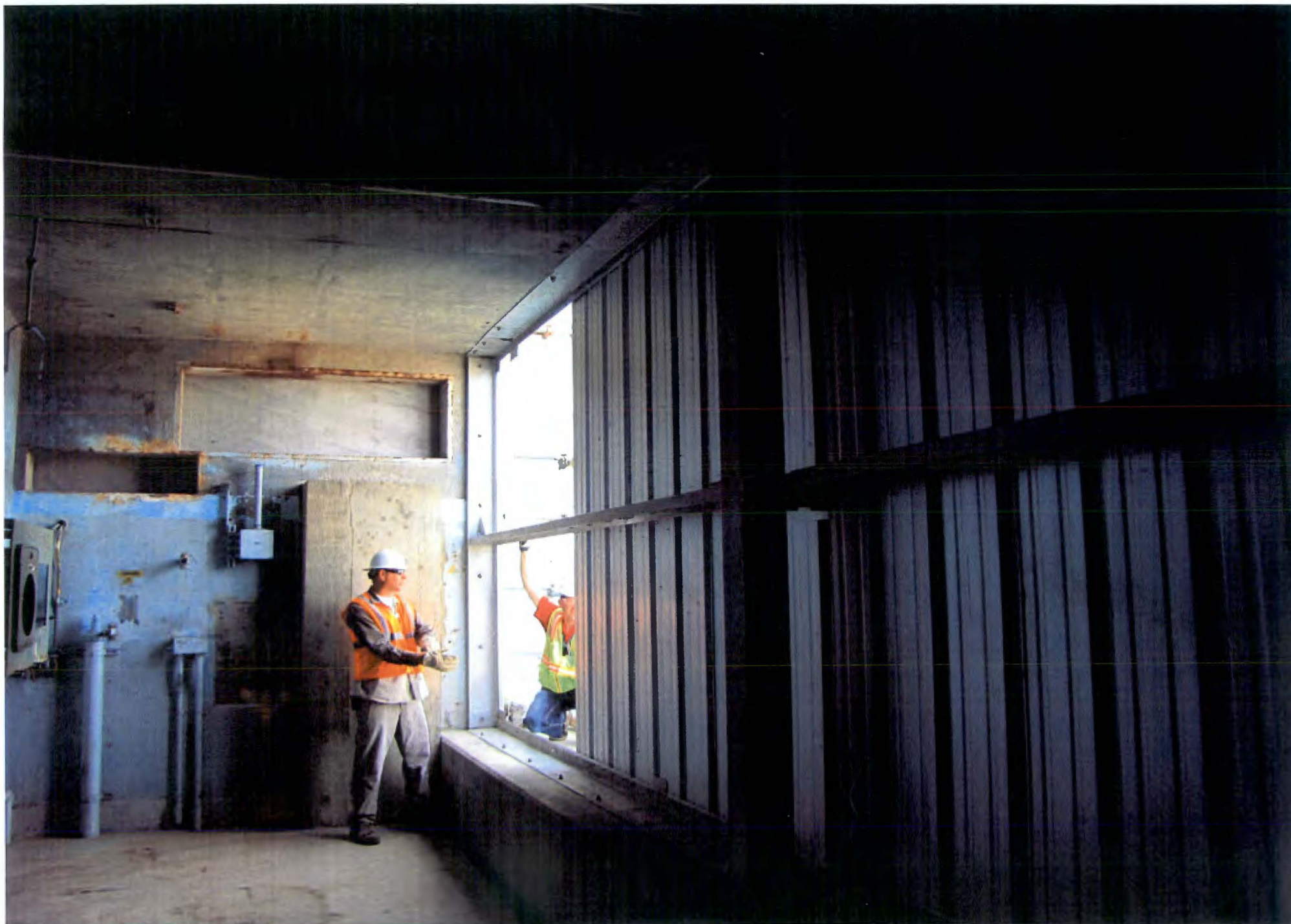
PHOTO # 538/105N/Corridor #22 Looking SW/EI.0'-0"/07-17-2012
