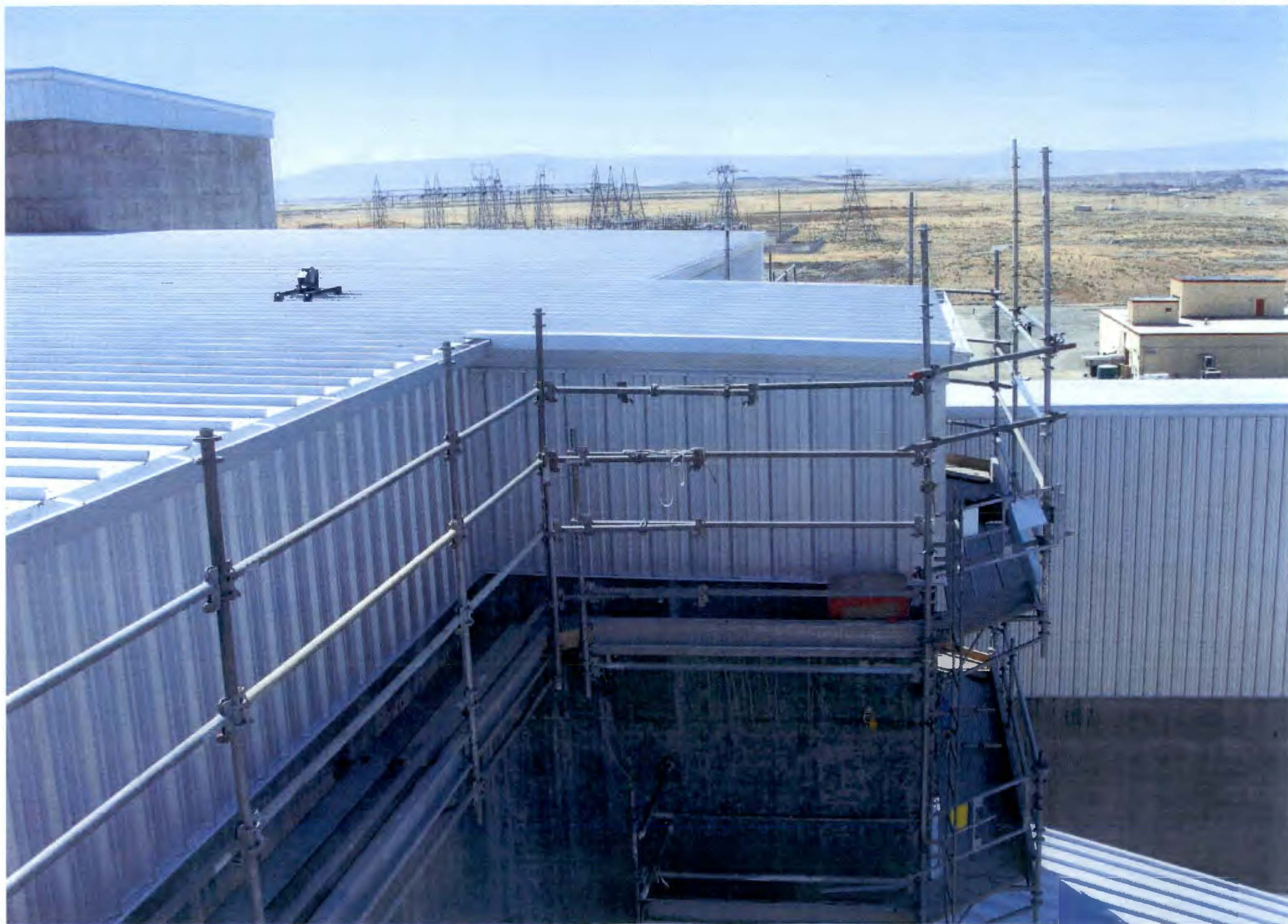
PHOTO # 507/105N/Rod Rm. SSE Roof-Gutter at Main Roof W. Side/EI.Varies/08-18-2011
