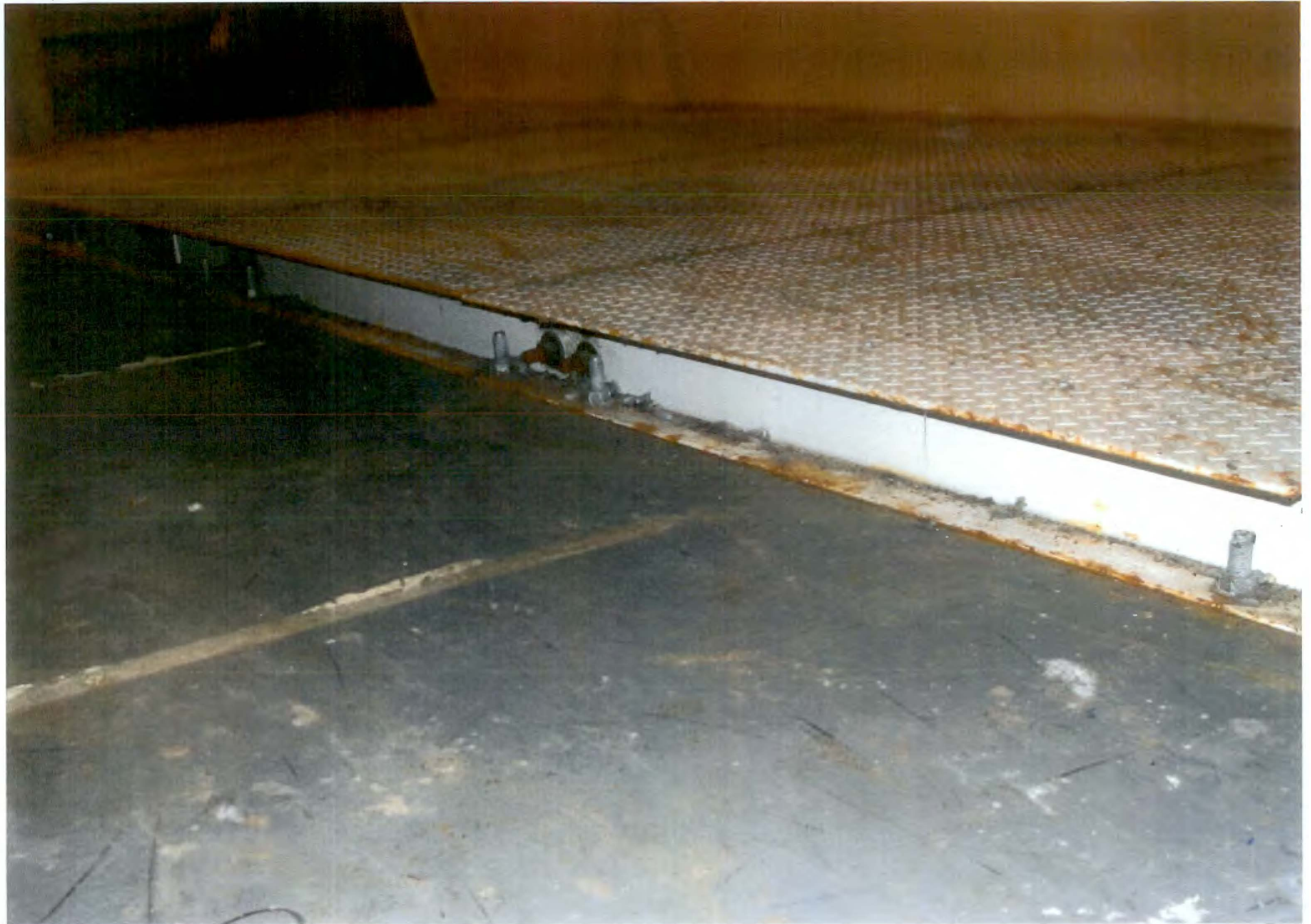
PHOTO # 521/105N/Rm.#175-Discharge Tunnel Cover Plates/El.+1-0"/06-05-2012
