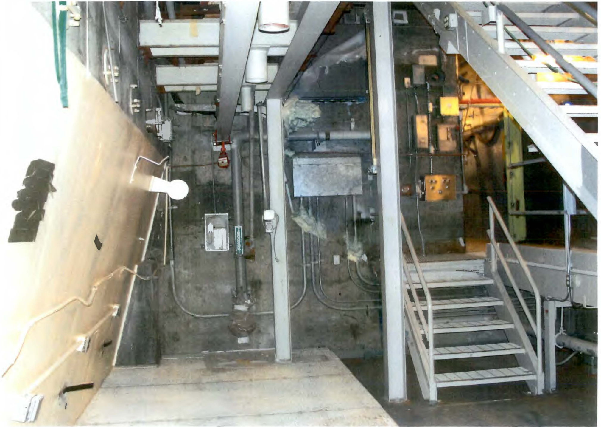
PHOTO # 519/105N/Rm.#175-Looking East/EI.+1'-0"/06-05-2012
