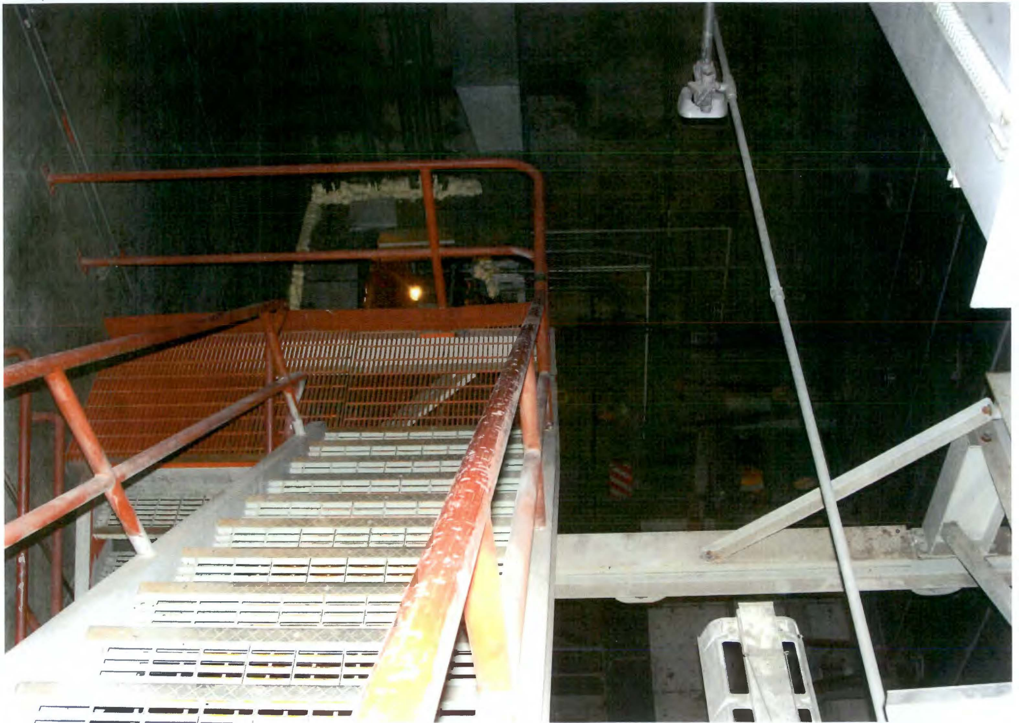
PHOTO # 515/105N/Stair#8 Looking Down from Platform/EI.+33-9"/06-05-2012
