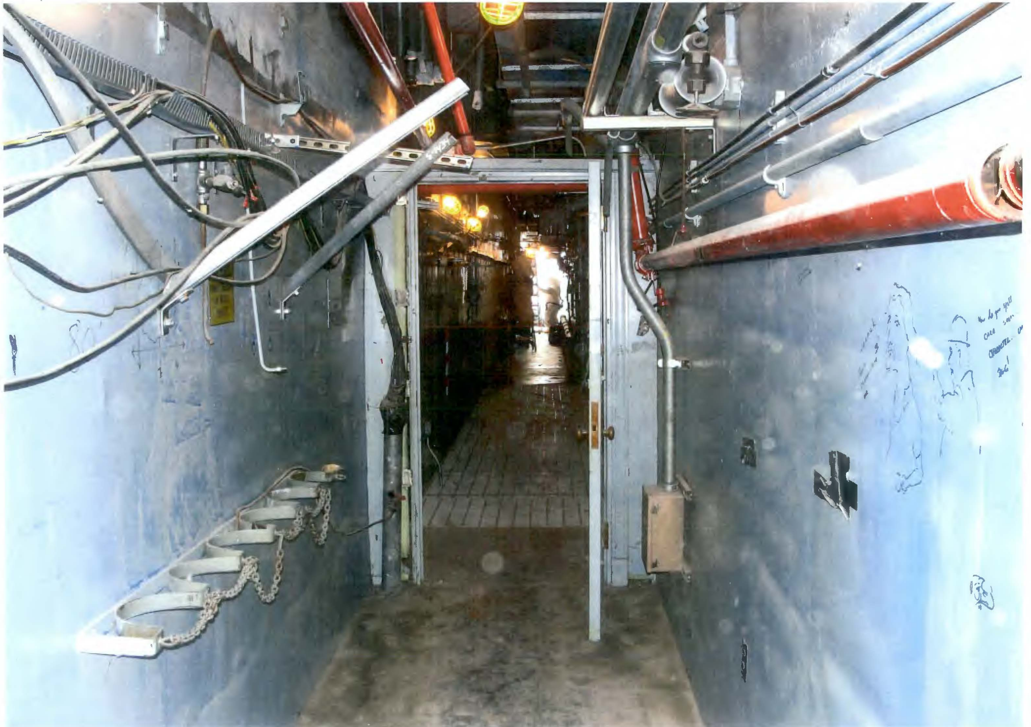
PHOTO # 524/105N/Corridor#7 Center Looking West/EL.+5'-0"/06-05-2012
