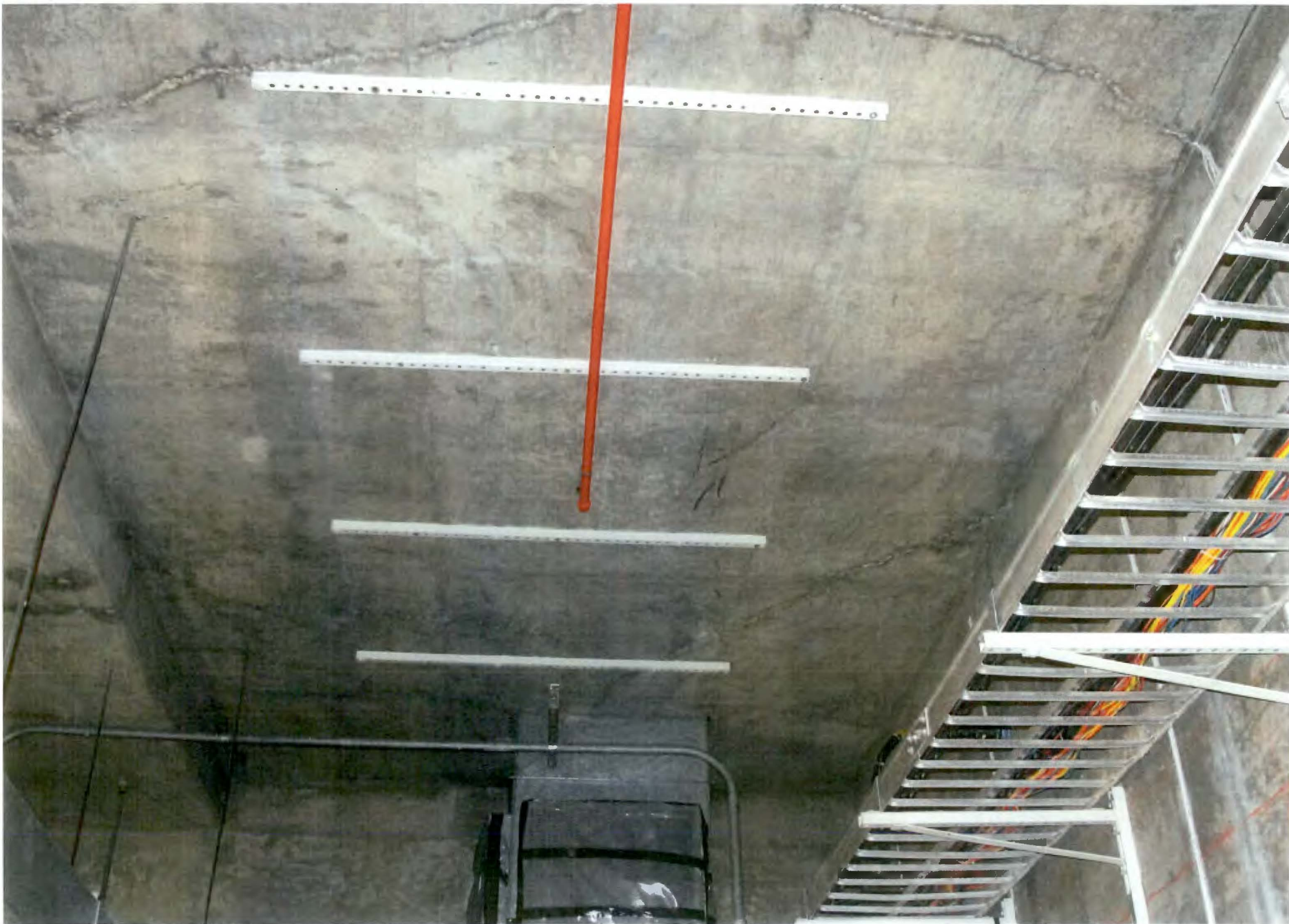
PHOTO # 512/105N/Rm.#507 Ceiling Looking West/EI.+43'-6"/06-05-2012
