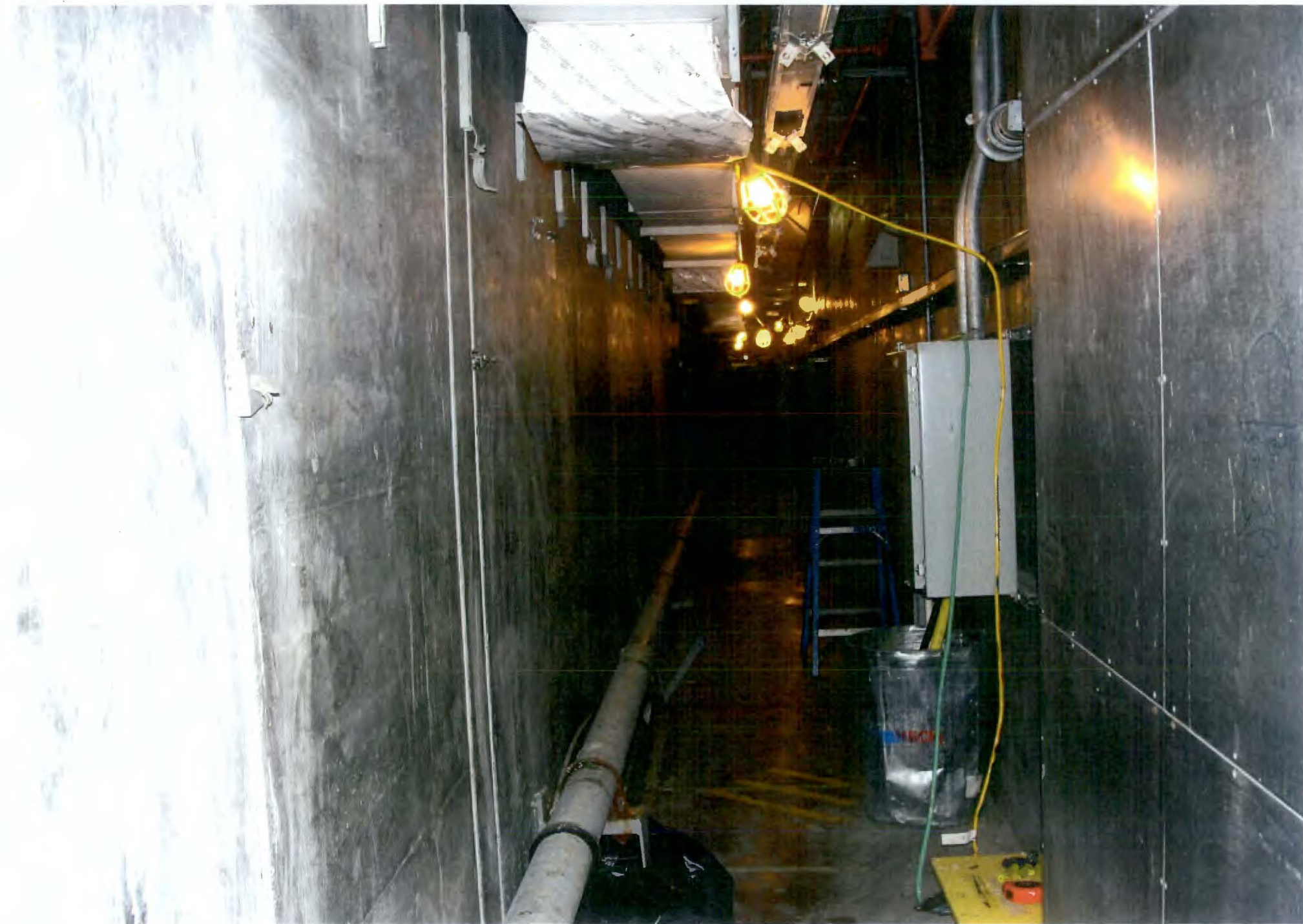
PHOTO # 531/105N/Corridor#7 West End Looking East/EI.+5'-0"/06-05-2012
