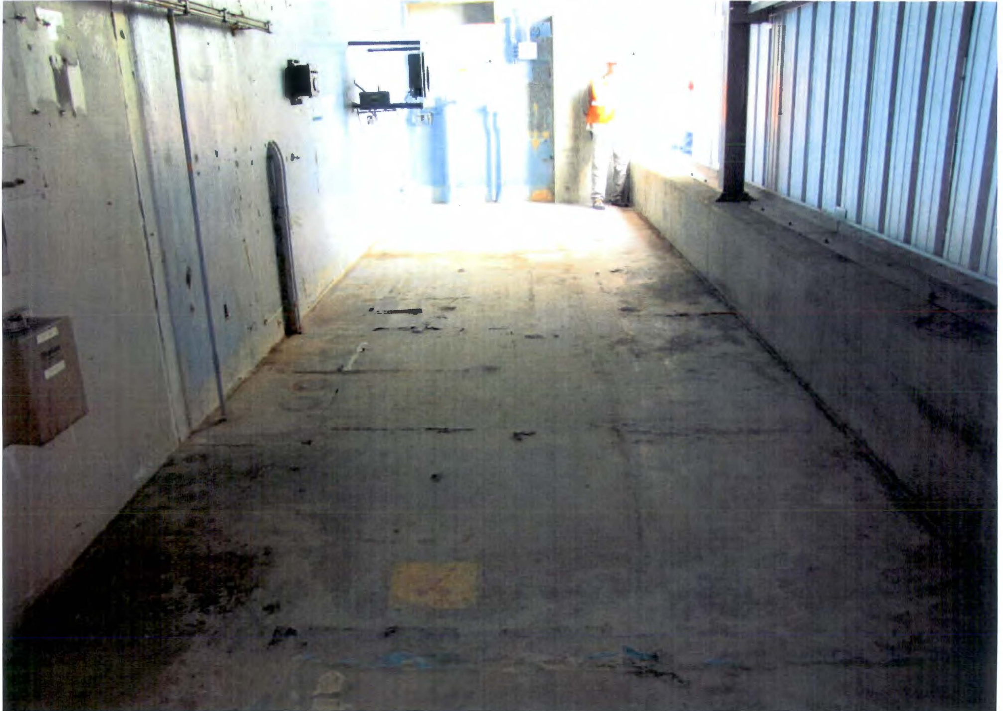
PHOTO # 539/105N/Corridor #22 Floor Looking South/EI.0'-0"/07-17-2012
