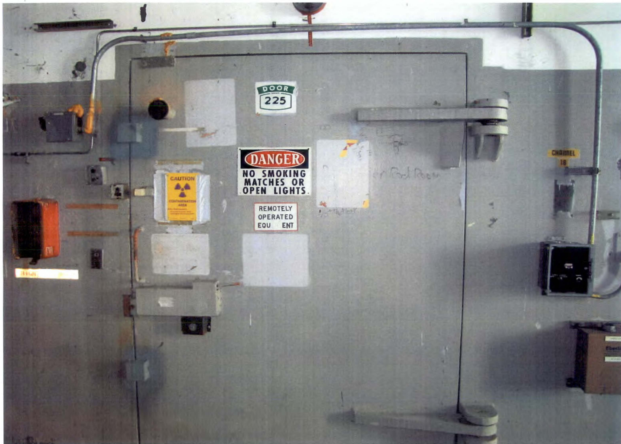
PHOTO # 532/105N/Corridor #22 Shld Door at East Wall/EI.0'-0"/07-17-2012
