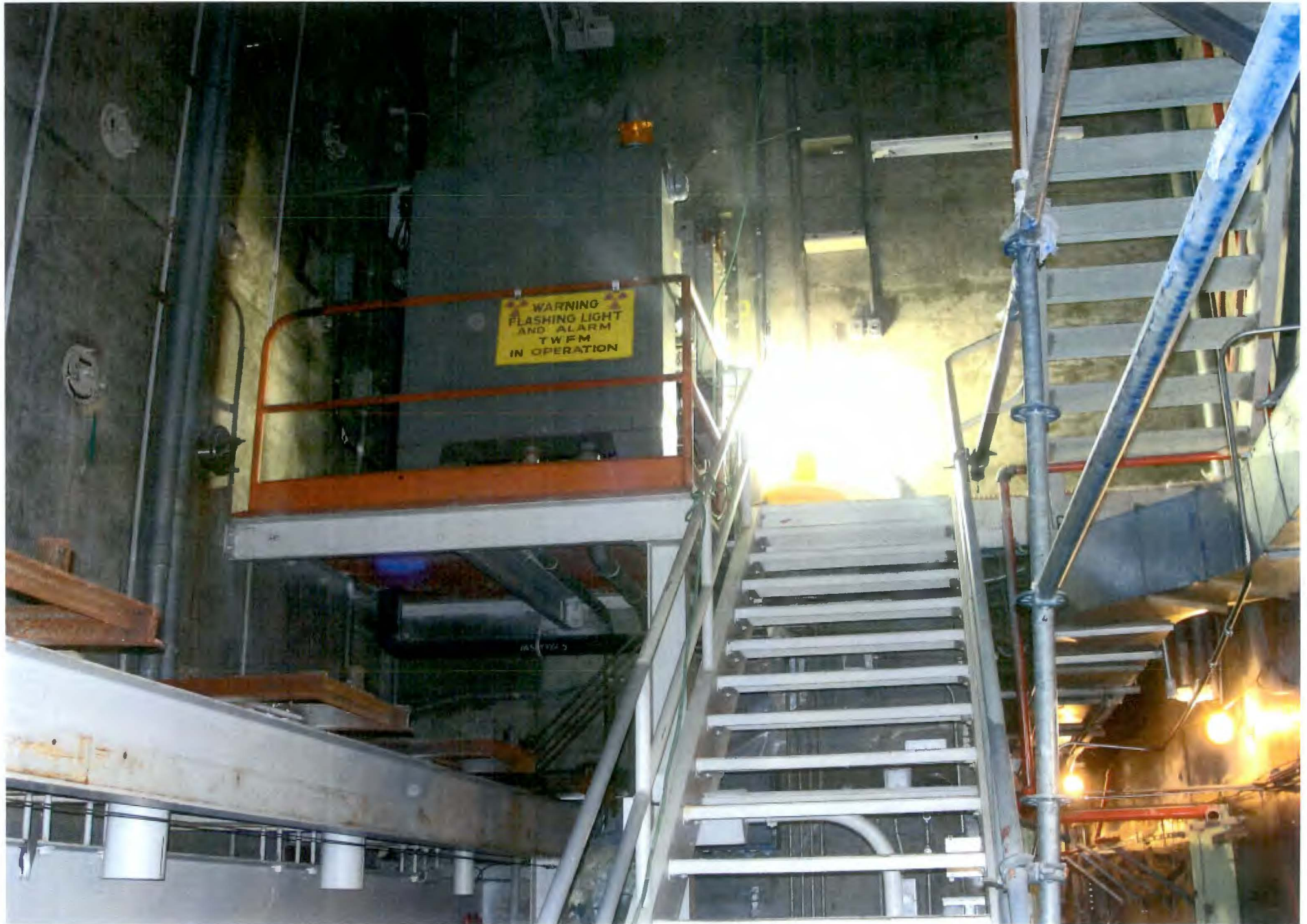
PHOTO # 518/105N/Stair#8-Looking East/EI.+1'-0"/06-05-2012
