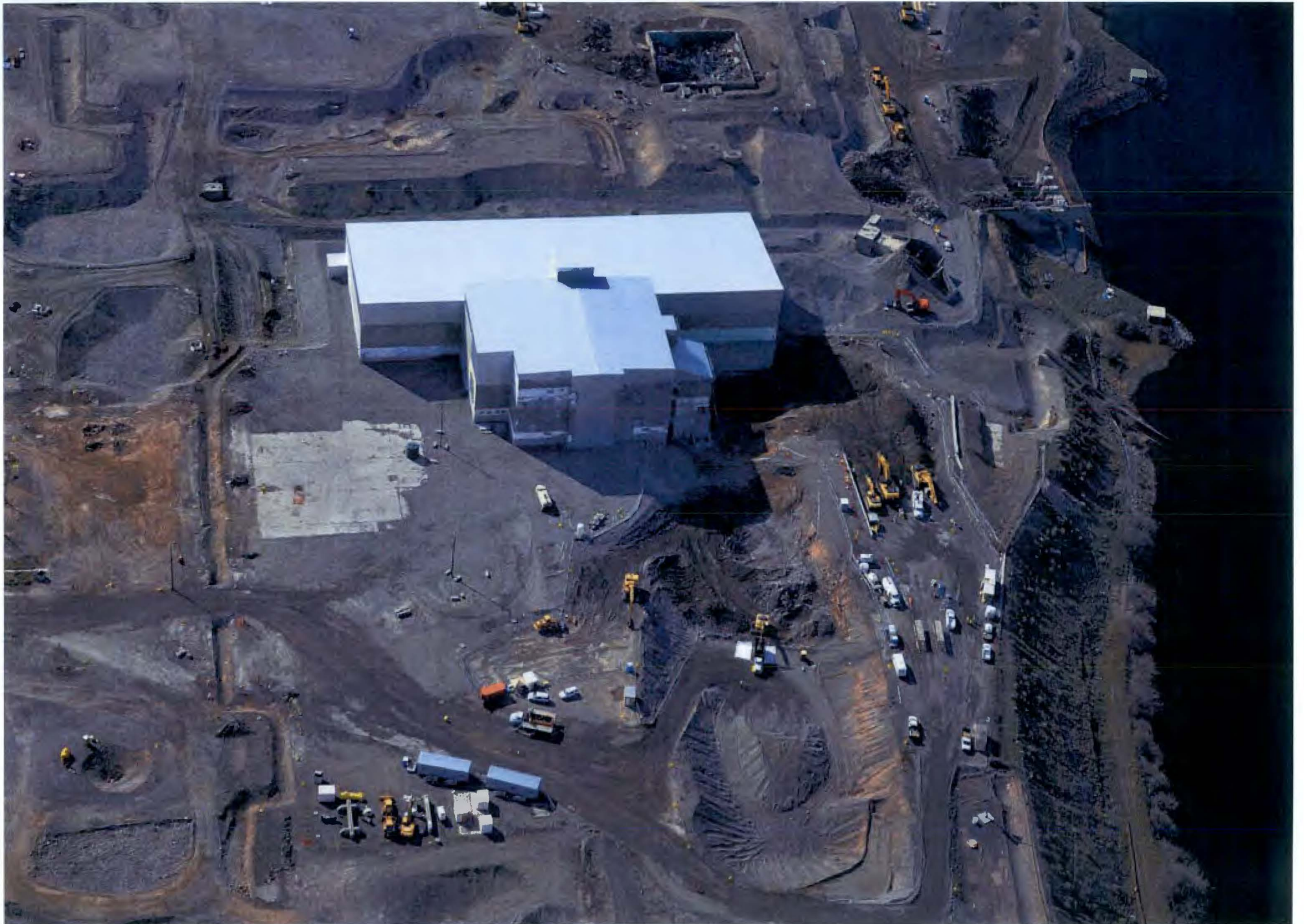
PHOTO # 508/105N/Main & Rod Rm. SSE Roof/EI.Varies/03-12-2012
