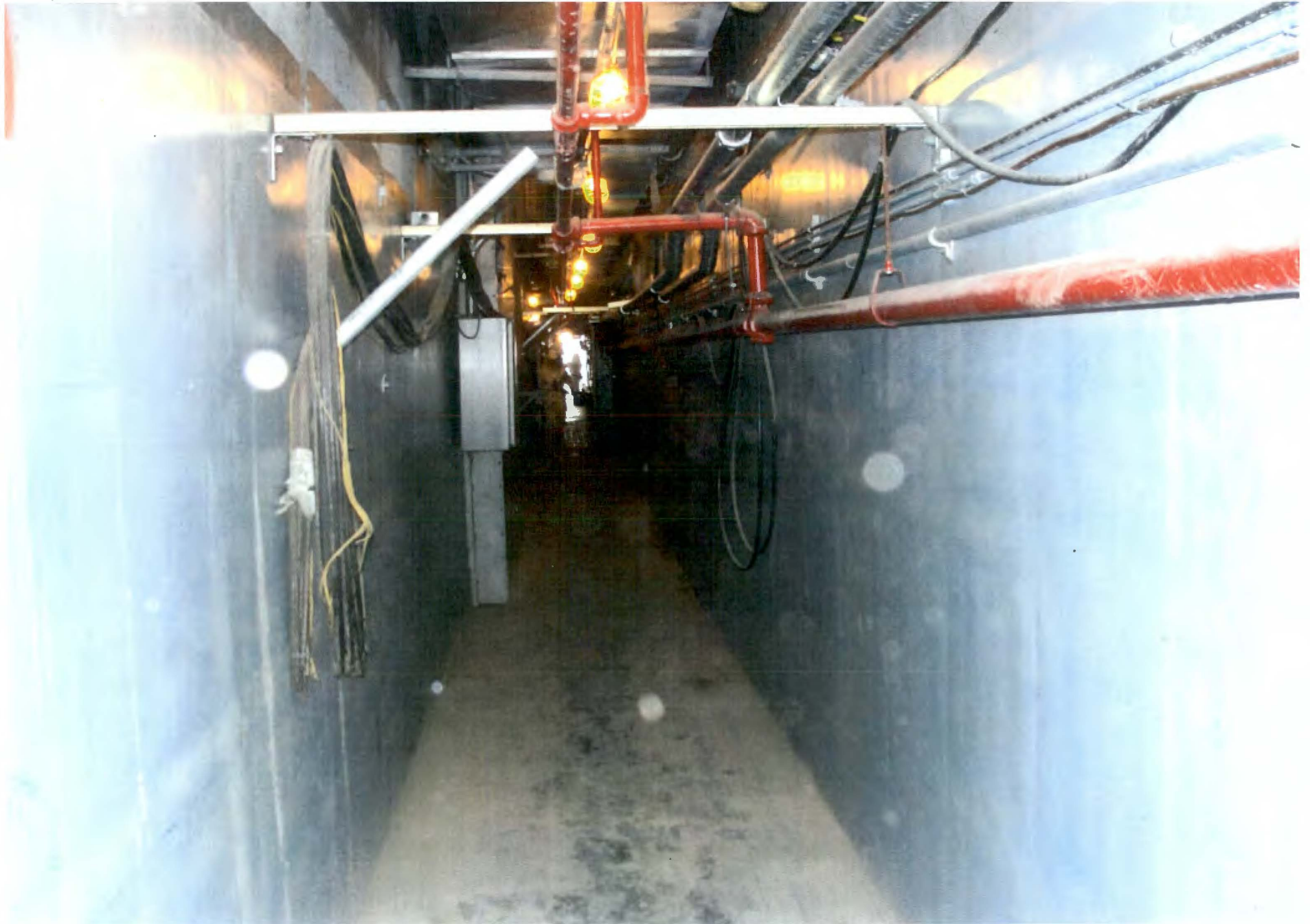
PHOTO # 523/105N/Corridor#7East End Looking West/EI.+5'-0"/06-05-2012
