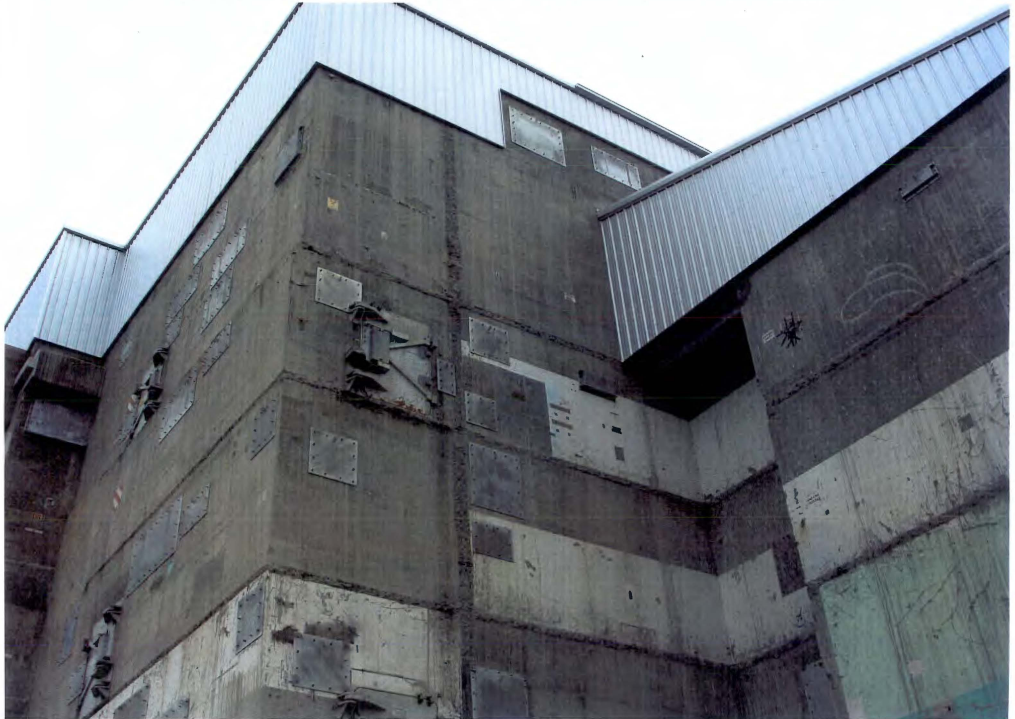
PHOTO # 543/105N/West Wall Above Grade-N. of Rod Rm./El.Varies/07-19-2012
