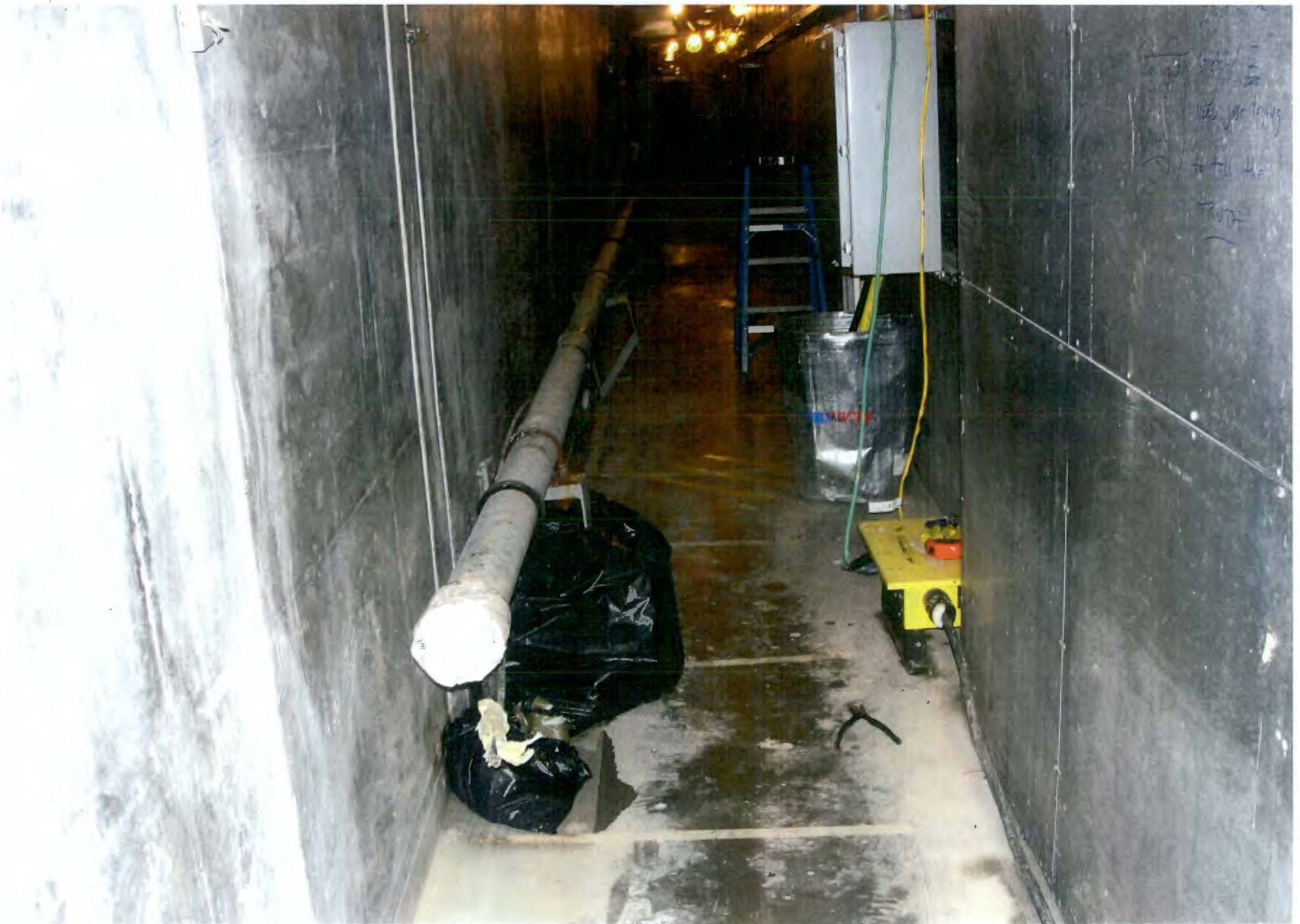
PHOTO # 529/105N/Corridor#7 West End Looking East/EI.+5'-0"/06-05-2012
