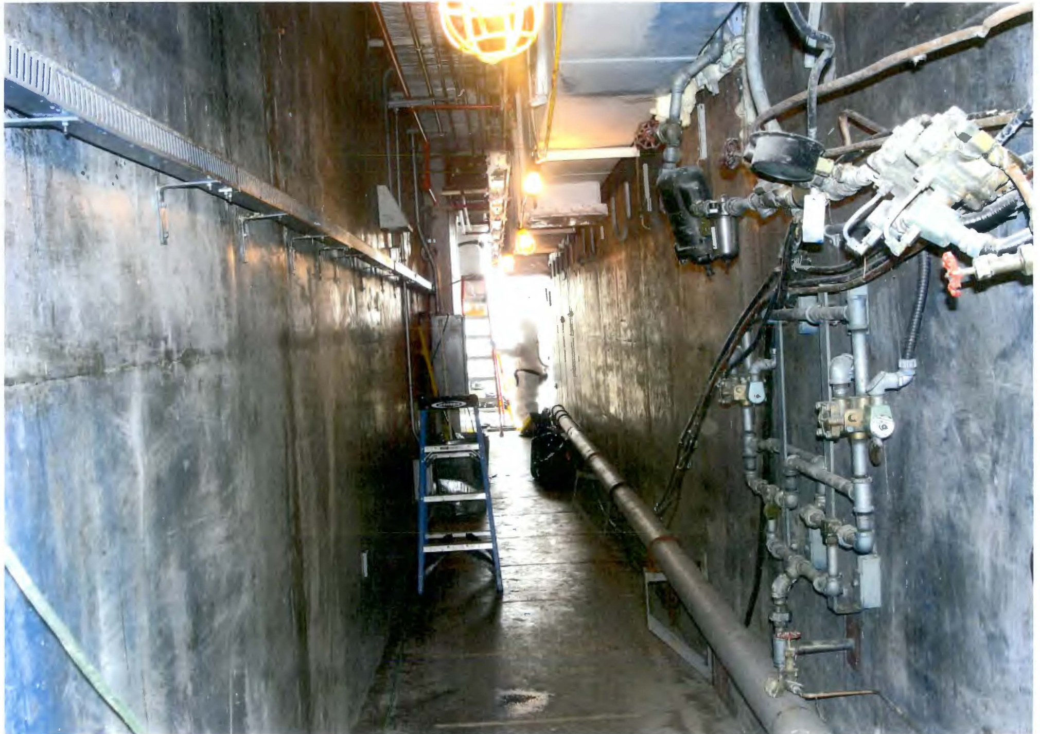
PHOTO # 527/105N/Corridor#7 West End Looking West/EI.+5'-0"/06-05-2012
