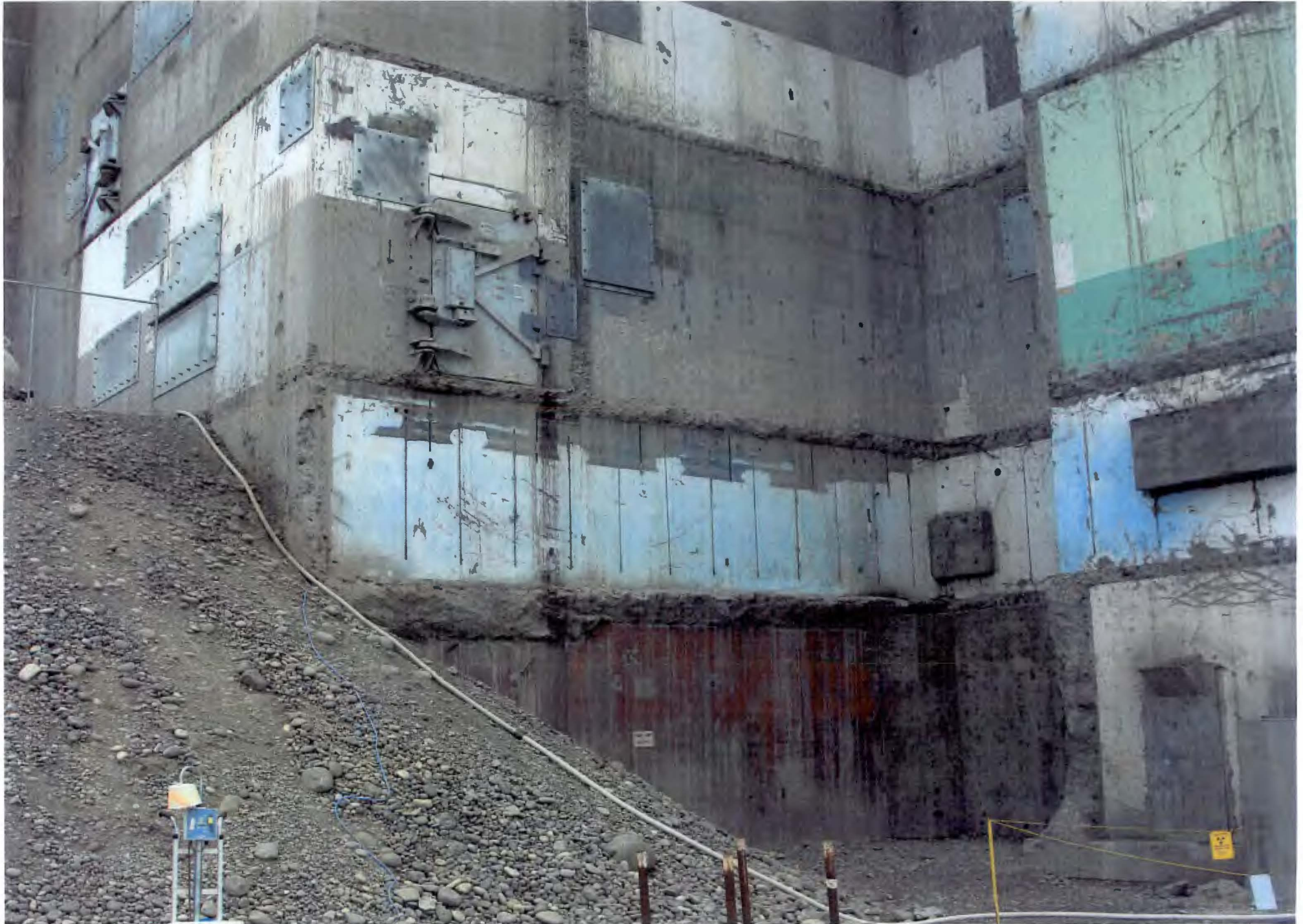
PHOTO # 542/105N/West Wall Below Grade-N. of Rod Rm./El.Varies/07-19-2012
