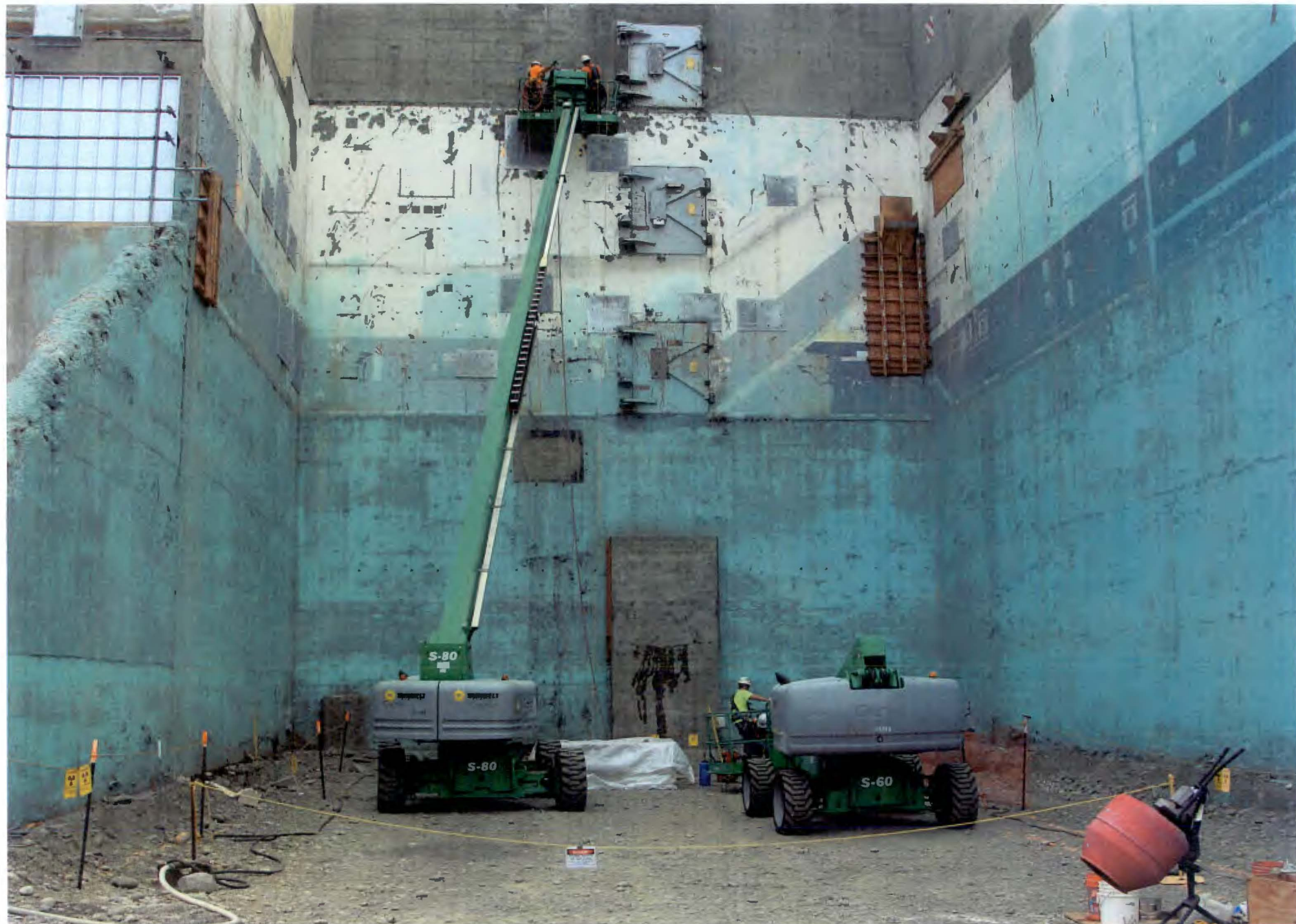
PHOTO # 544/105N/W. Wall Below Grade Between Rod Rm. & 109N/EI.Varies/07-19-2012
