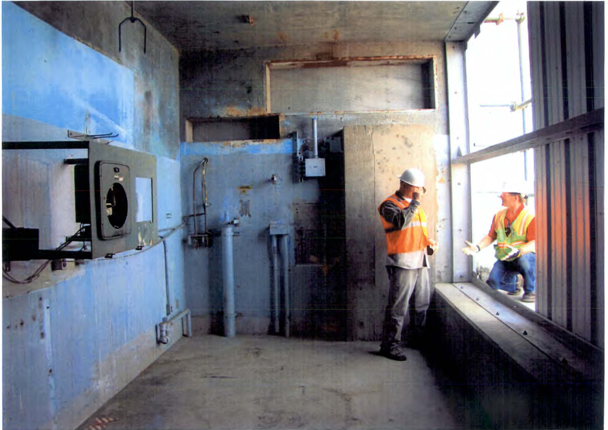
PHOTO # 536/105N/Corridor #22 Looking South/EI.0'-0"/07-17-2012
