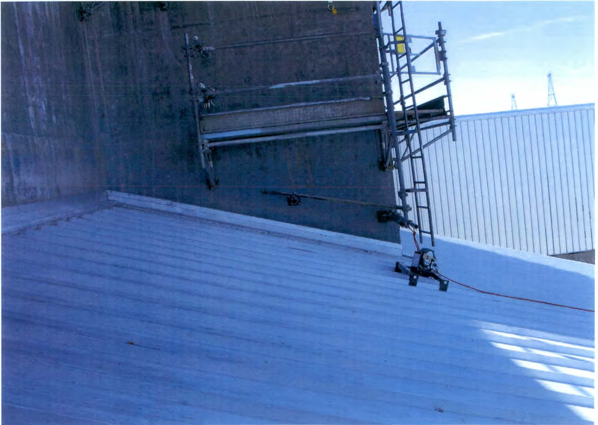
PHOTO # 504/105N/Rod Rm. SSE Roof-Looking South/El.Varies/08-18-2011
