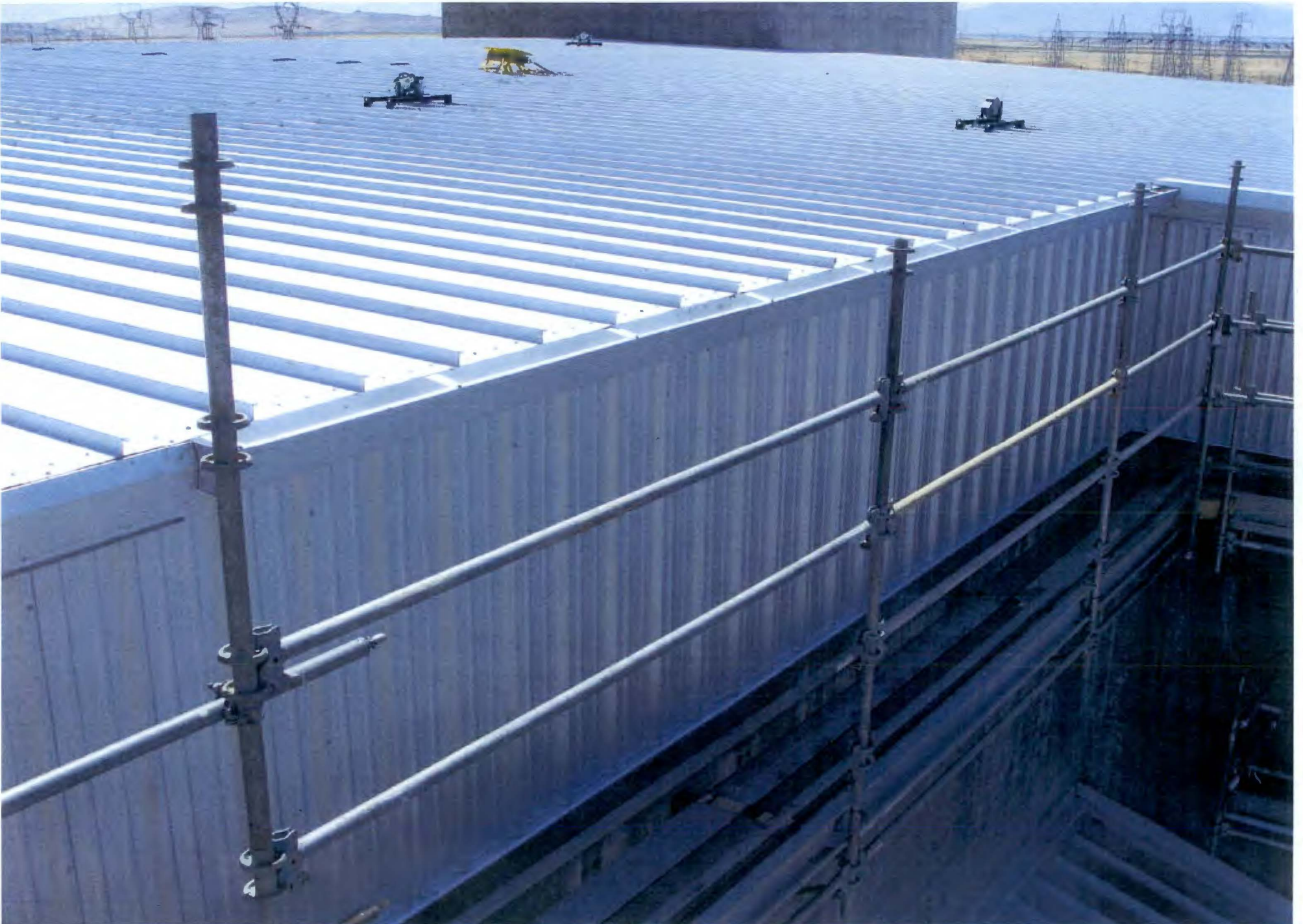
PHOTO # 506/105N/Rod Rm. SSE Roof-Gutter at Main Roof W. Side/EI.Varies/08-18-2011
