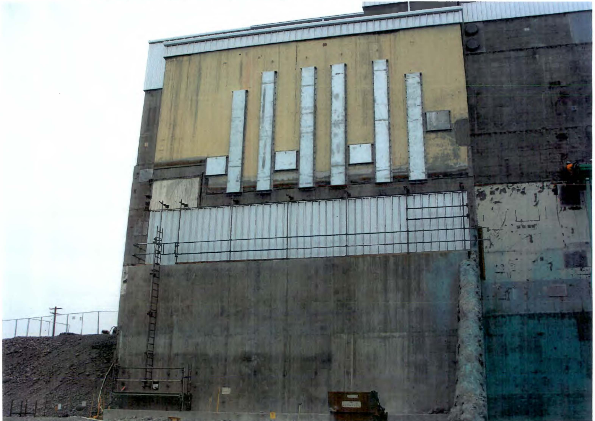
PHOTO # 541/105N/Corridor #22 W. Exterior Wall & W. Wall of Rod Rm./El.Varies/07-19-2012
