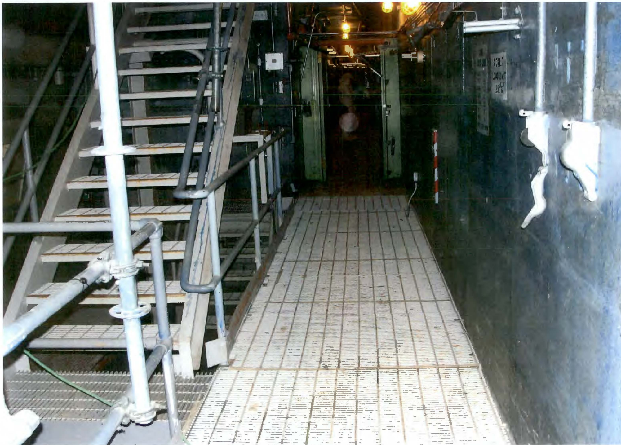
PHOTO # 526/105N/Corridor#7 Center Looking East/EI.+5'-0"/06-05-2012
