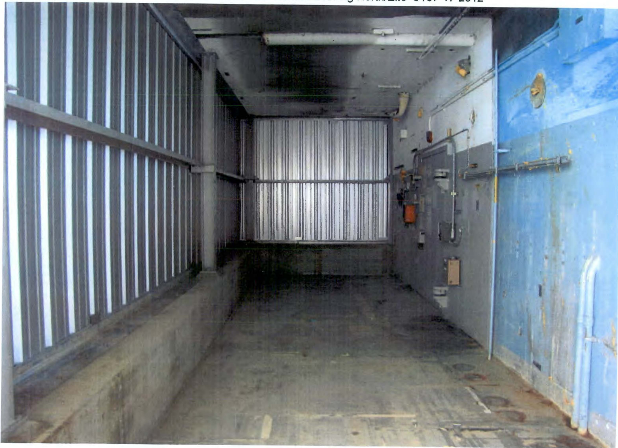
PHOTO # 534/105N/Corridor#22 Looking North/EI.0'-0"/07-17-2012
