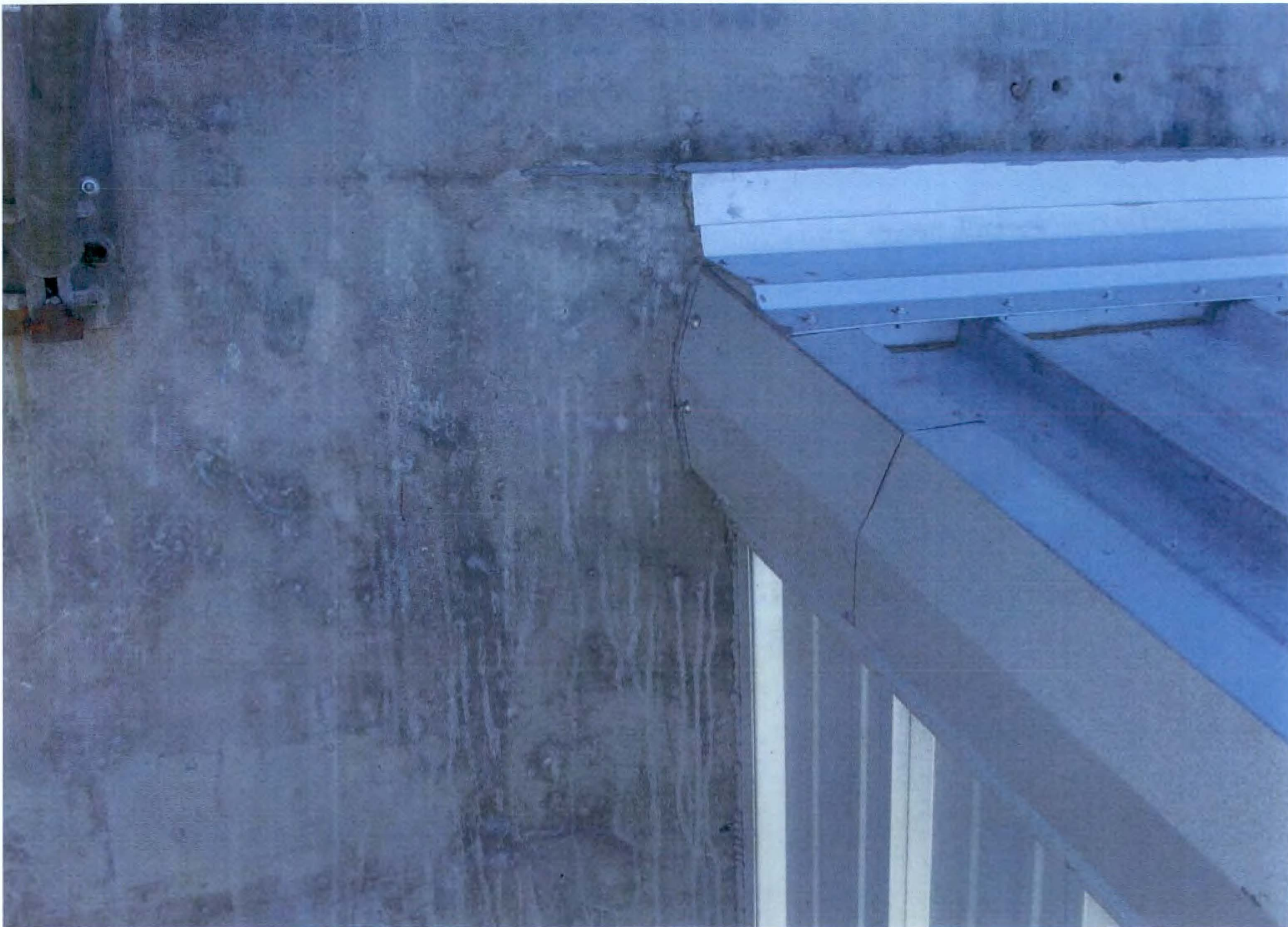
PHOTO # 505/105N/Rod Rm. SSE Roof-Flashing at NE Corner/EI.Varies/08-18-2011
