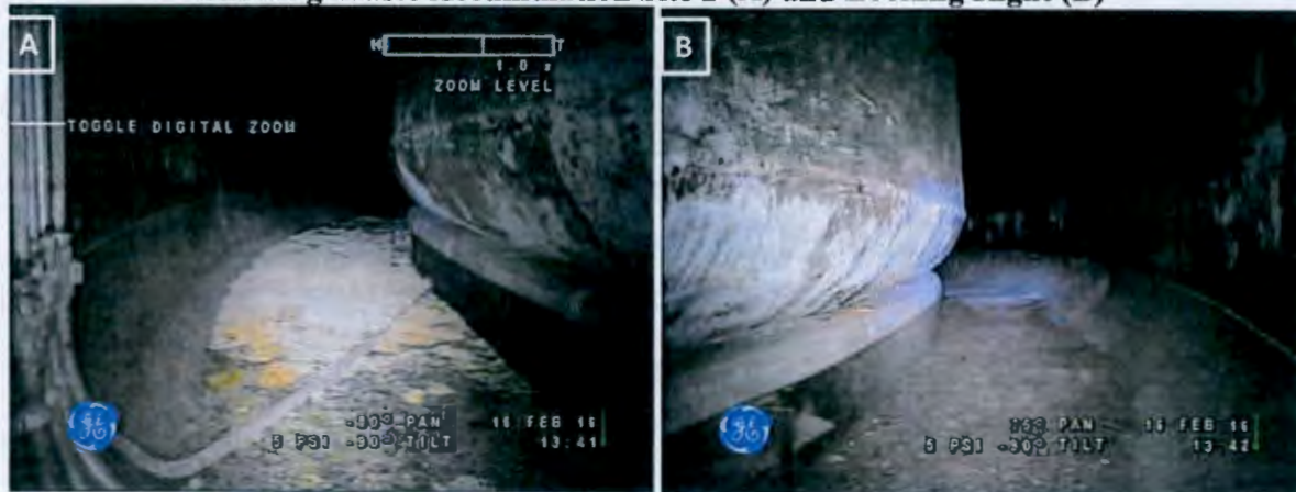
Figure 10. General Condition of the Annulus Floor on 2/16/2016 at 325° Looking Left Showing Waste Accumulation Site 2 (A) and Looking Right (B)
