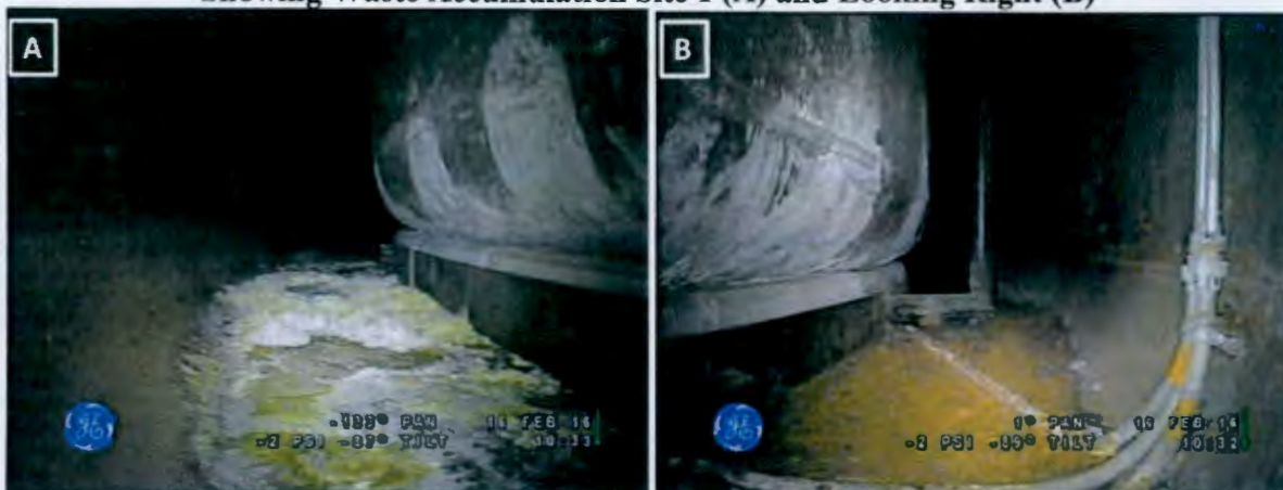
Figure 8. General Condition of the Annulus Floor on 2/16/2016 at 215° Looking Left Showing Waste Accumulation Site 1 (A) and Looking Right (B)
