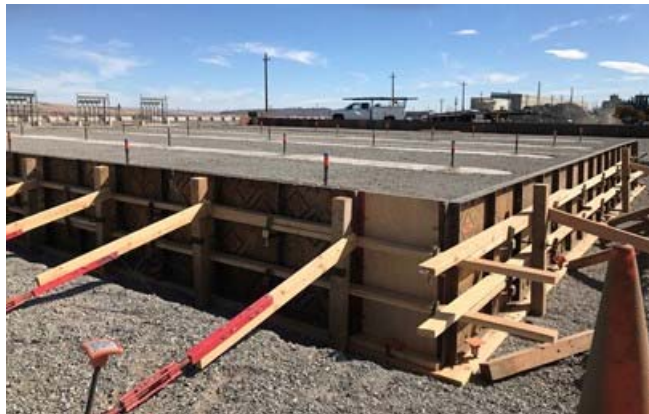
Capsule Storage Pad Formwork
