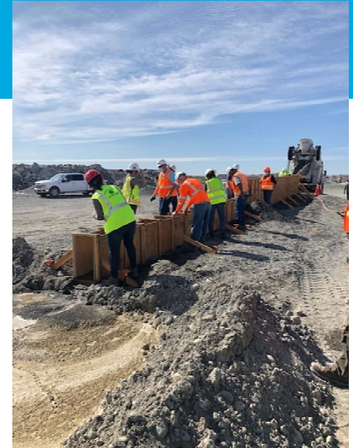
Aging structures team demonstrates grout flowability mix design at American Rock
