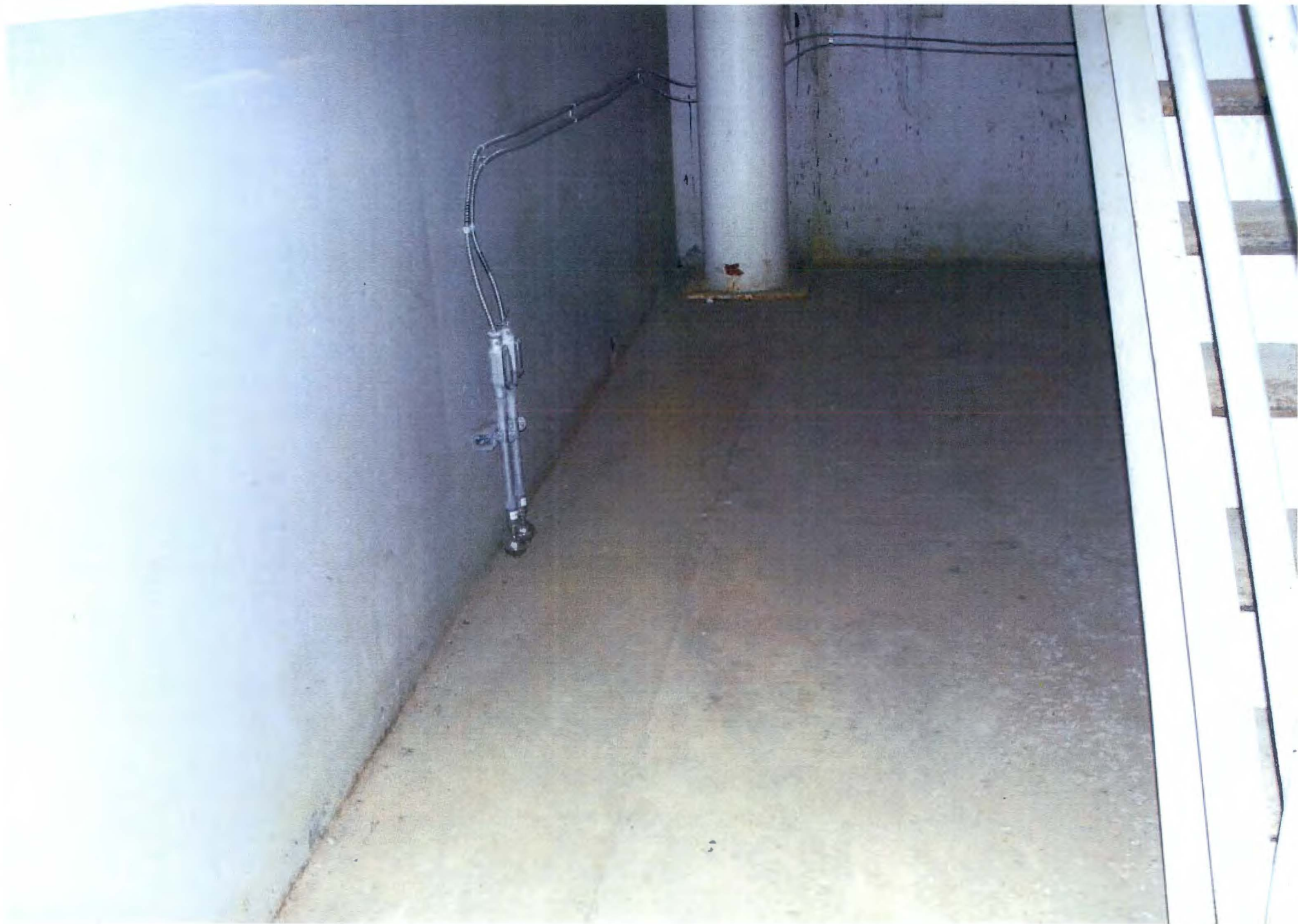
PHOTO # 429/105N/Stair#6 Level Switches-Bottom of Stair/EI.(-)24'/02-15-2012
