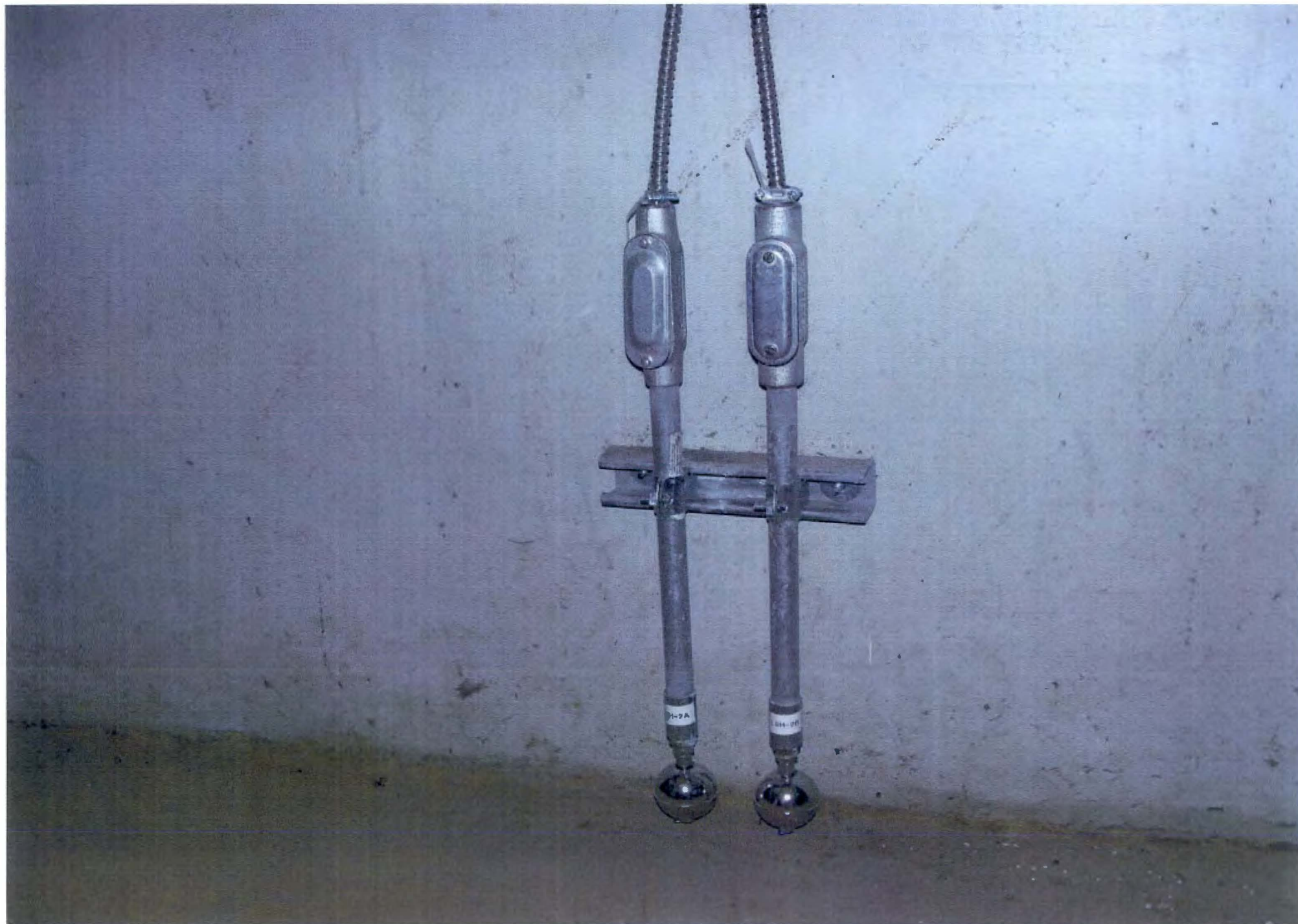
PHOTO # 430/105N/Stair#6 Level Switches-N. Wall Bottom of Stair/El.(-)24'/02-15-2012
