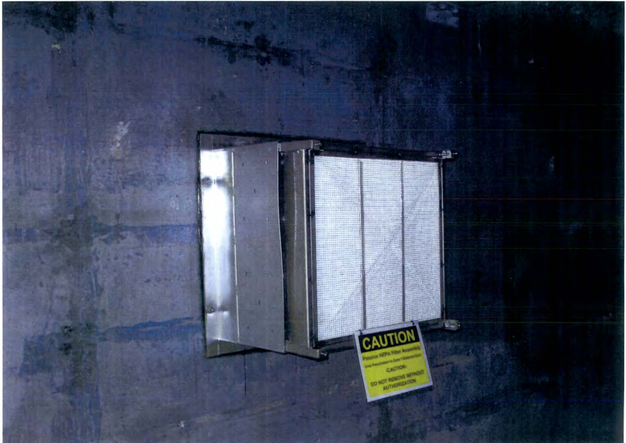
PHOTO # 420/105N/Rm.#607 Passive HEPA Filter in Wall of Zone I Duct-South Wall/EI.+60'-6"/02-07-2012
