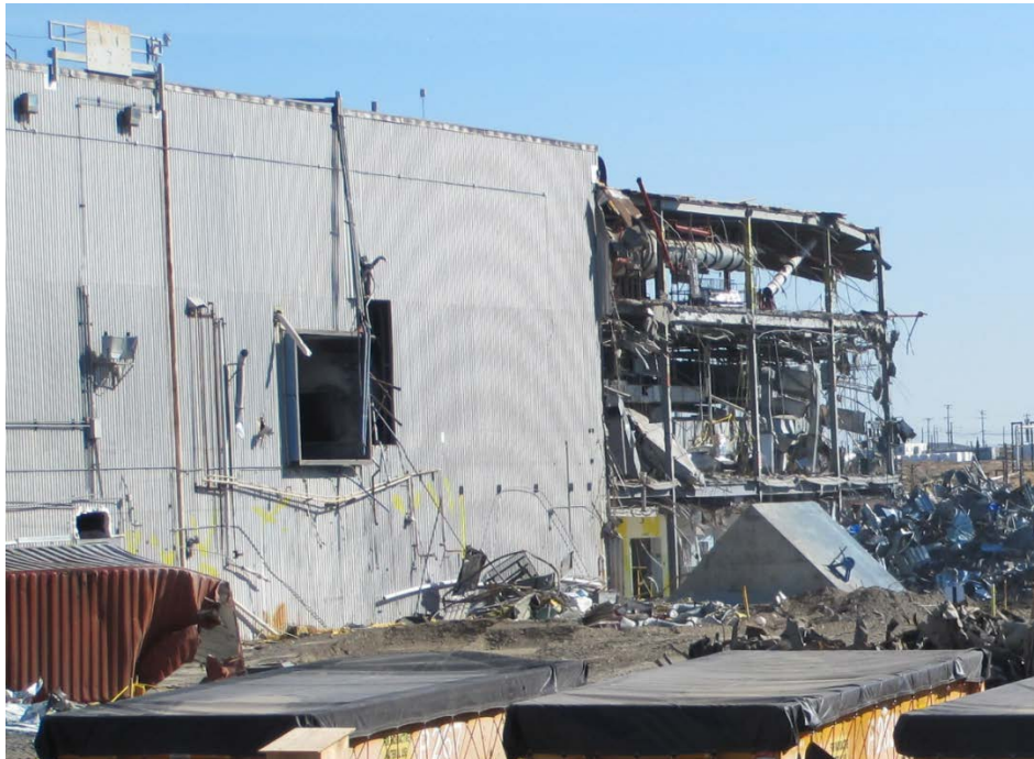
Figure 2. 2734ZC Post Demolition
