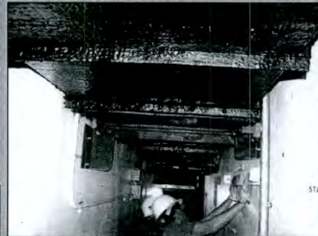
Application Of Polyurea To Stabilize Duct In Building 291-Z
