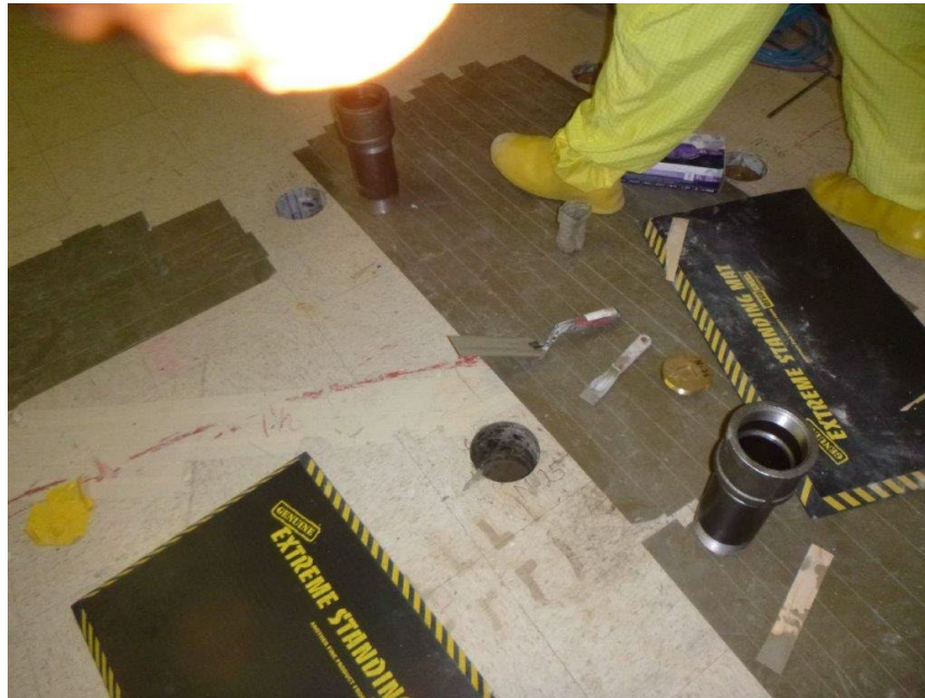
Preparing to install nipple into Room 131 drilled core
