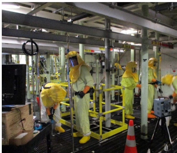
Team Manipulating Debris with Long-Pole Tools
