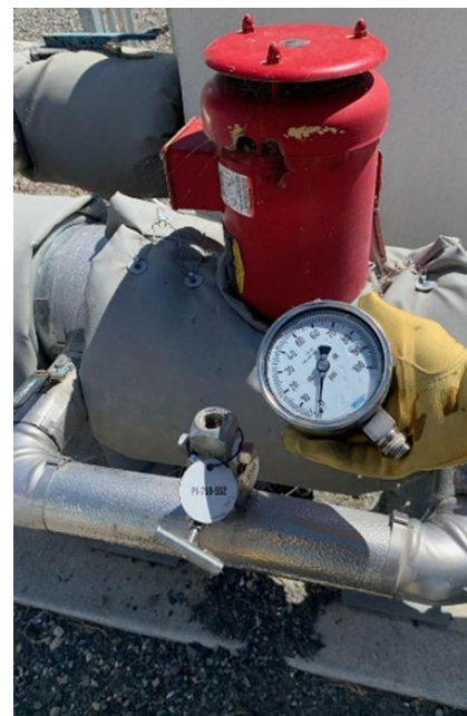
Leak Checking Backflow Preventor (Left) and Glycol Supply Instrument Removal (Right)
