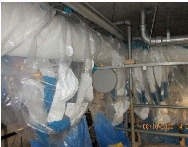
Glove Bag Installation in 105KW Pipe Gallery
