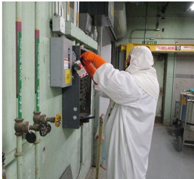
Disconnecting Wiring Circuits and Safe-Off in Support of Rod Rack and Door 157 Deactivation
