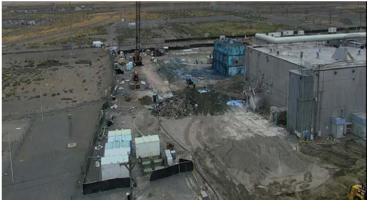
Figure 2. Bulk Chemical Storage Tank Farm Post-Demolition
