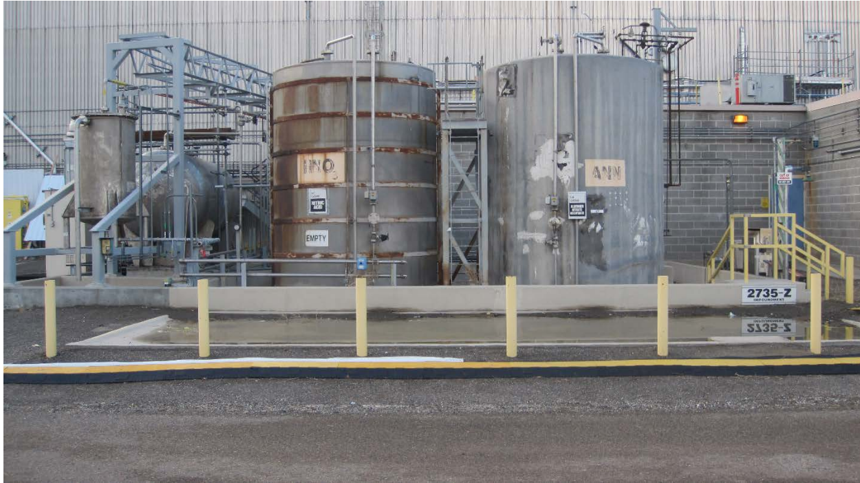
Figure 1. Bulk Chemical Storage Tank Farm Pre-Demolition
