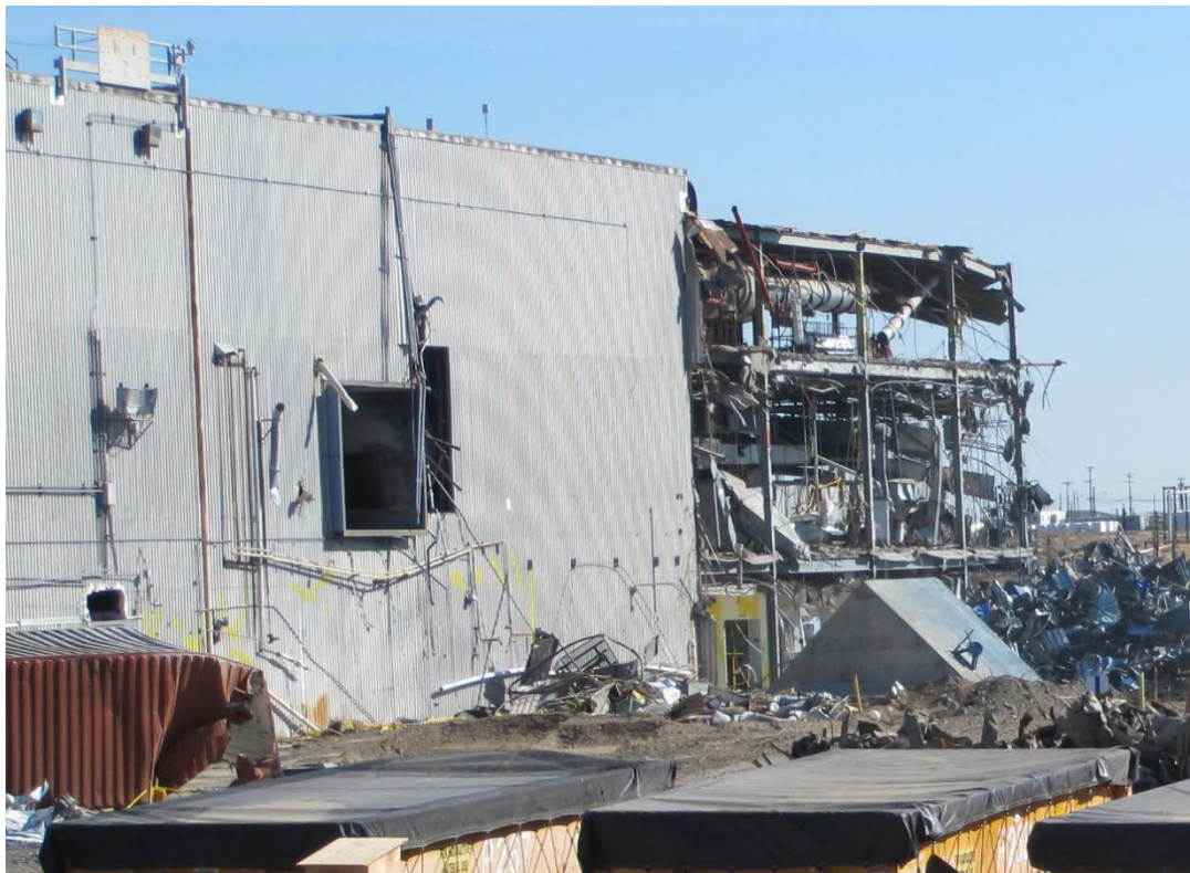
Figure 3. 2734ZB Post Demolition
