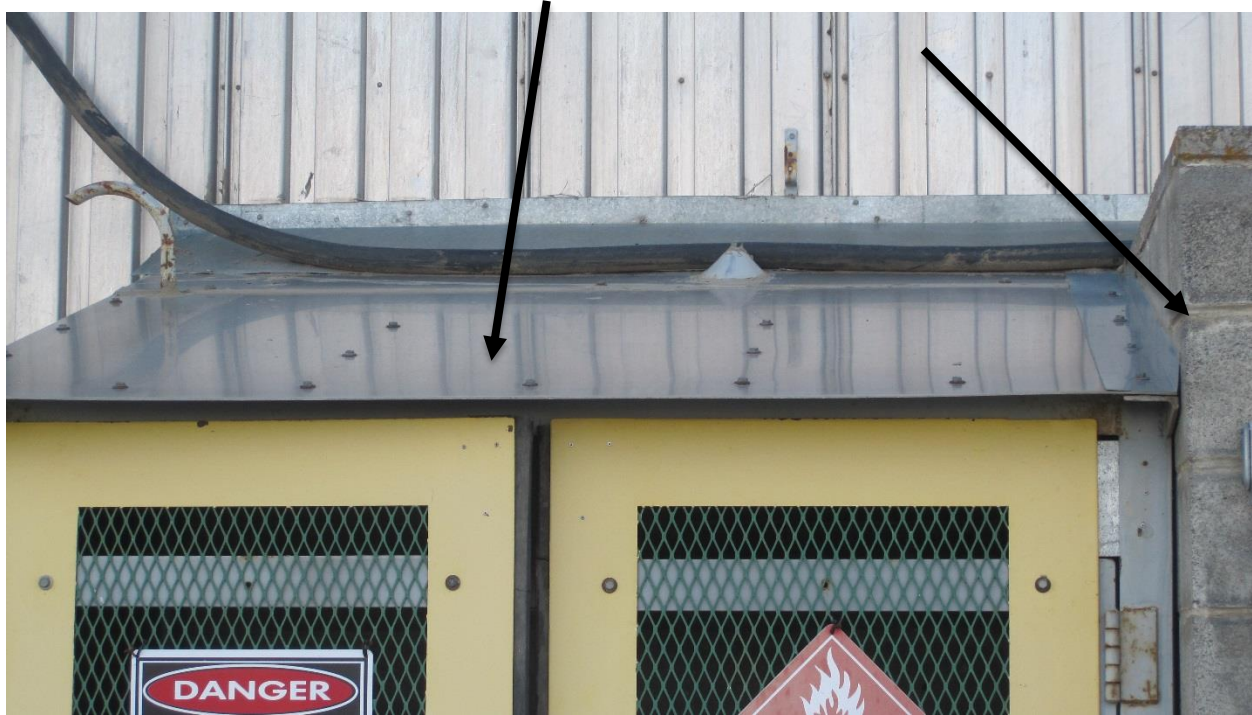
Figure 9. Close Up of Roof and Supporting Interior Cinderblock Wall
