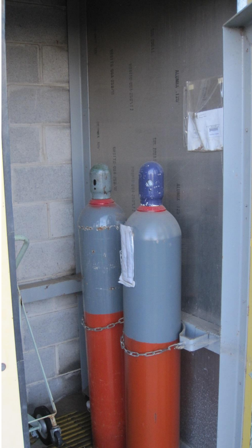
Figure 5. Photograph of Nonflammable Gas Storage Interior; Back Wall (Cinderblock), Sidewall (Aluminum)
