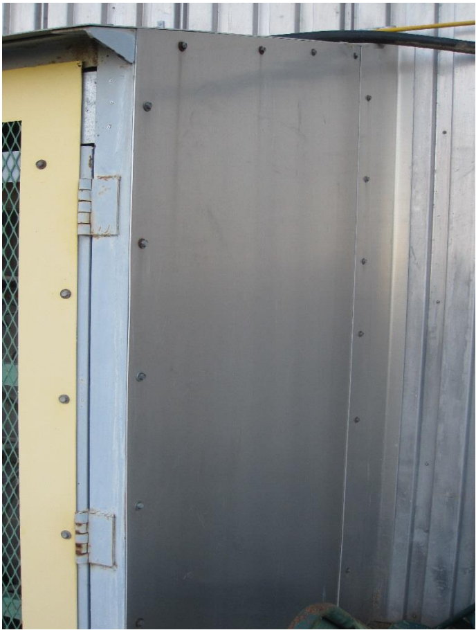
Figure 7. Exterior; West Wall
