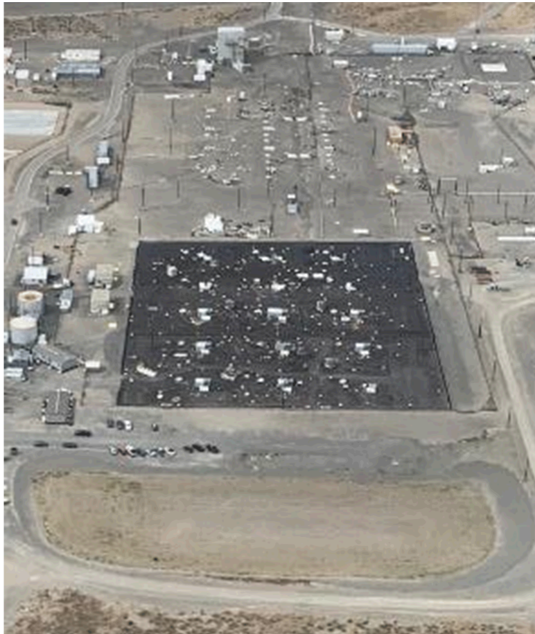
Figure 3. SX Tank Farm Interim Surface Barrier.
