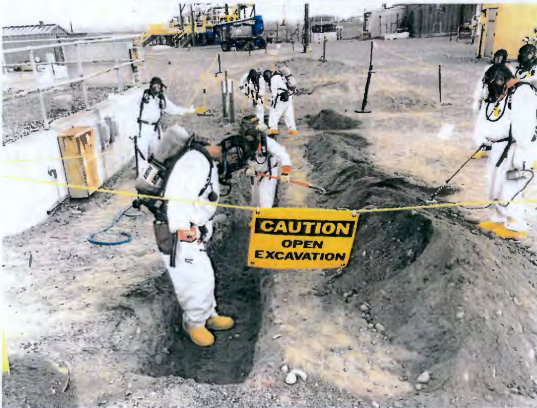
Excavations in the AX Farm to install the AY-102 waste transfer lines
