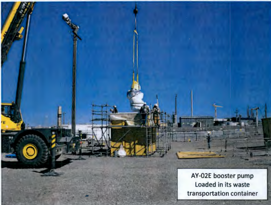
April 2015: Removal and disposal of the AY-02E booster pump
