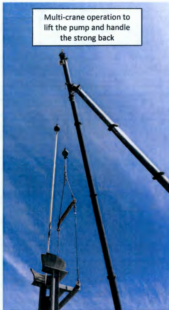
April 2015: Dry run on the AY-02E transfer pump removal lift
