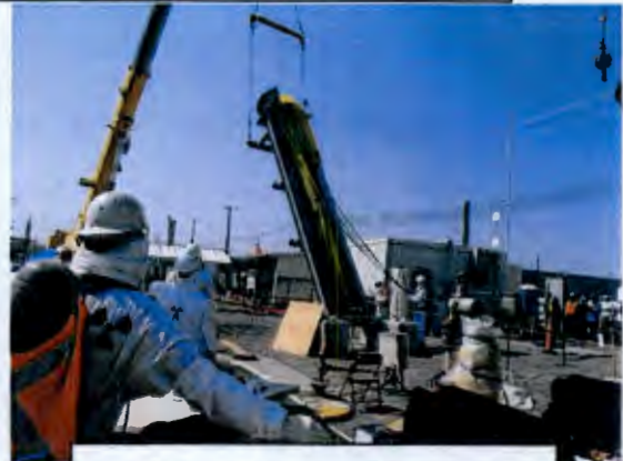
4 & 5- Lay down of the pump
