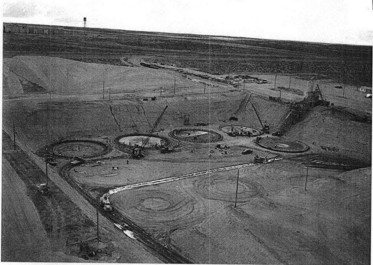
Figure C.2. Hard Packed Surface Caused By Construction Traffic
