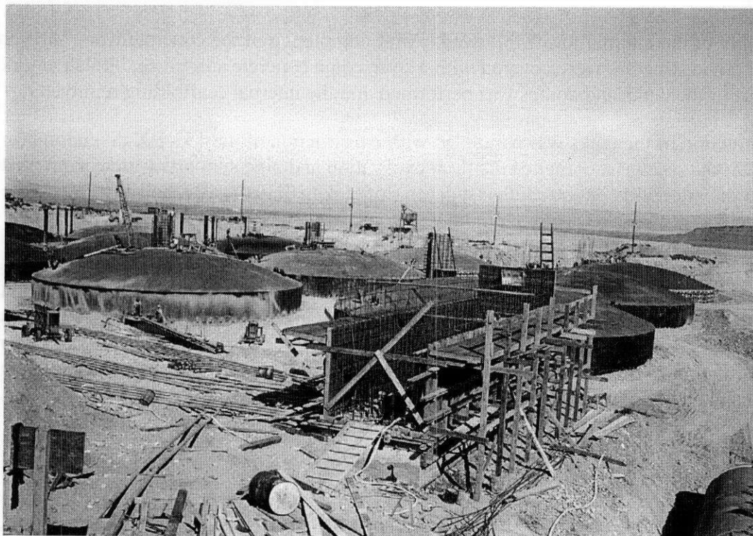
Figure C.8. Tank BX-153 with Feed Lines in Place
