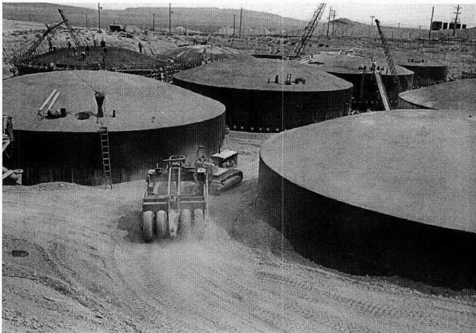
Figure C.11. Belly-Dumper During Backfill of BX Tank Farm
