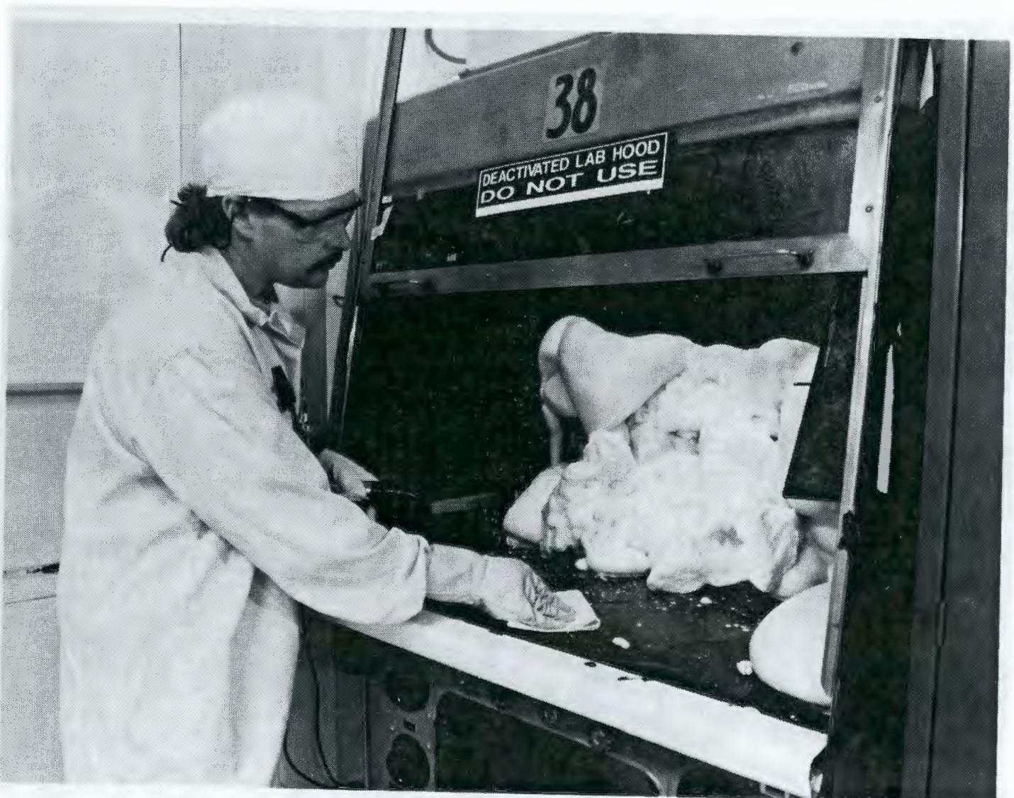
Figure 33. Foam is Spread Inside PUREX Laboratory Hood in Final Deactivation Step, 1996.
