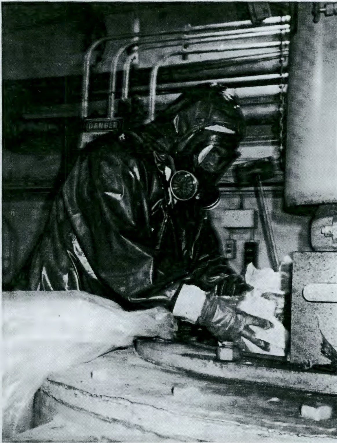
Figure 42. Worker Cleaning Calciner as Part of UO_3 Plant Deactivation, 1994.
