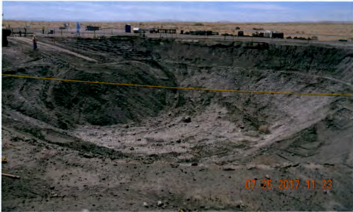
Figure 4. 600-63 Pit Post-Excavation (Looking South)
