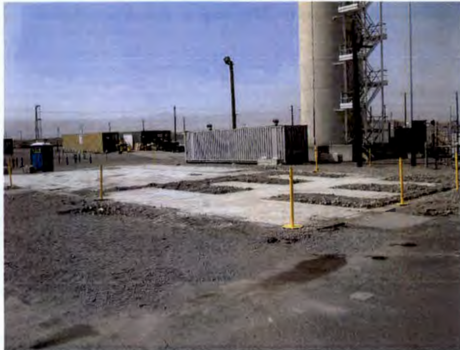
Figure 2. 243Z and 296Z015 Post-demolition
