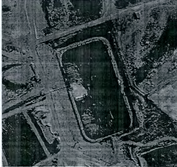
1312-N Liquid Effluent Retention Basin, Pre-Demolition, Aerial
