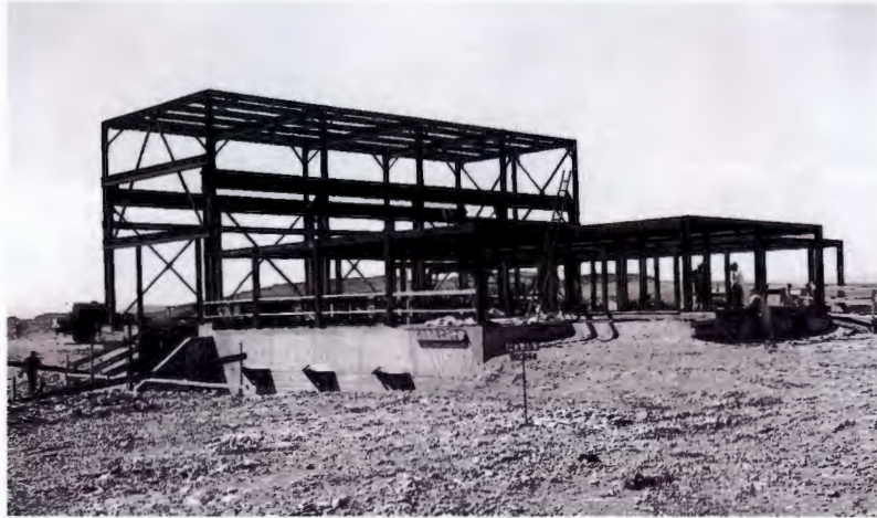
Figure 2-5. 212 Building Under Construction.
