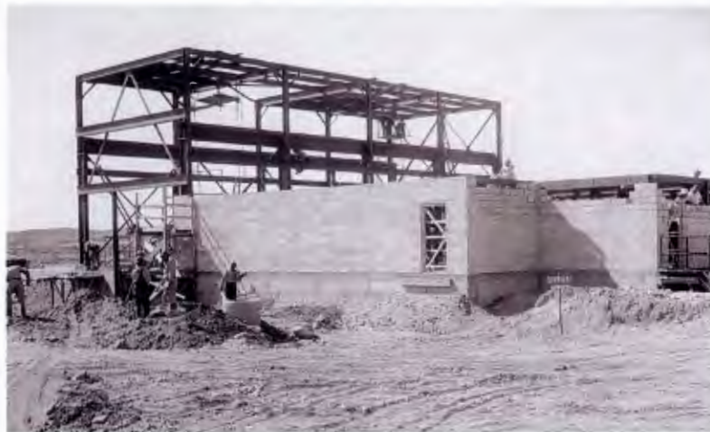
Figure 2-6. 212 Building Under Construction.
