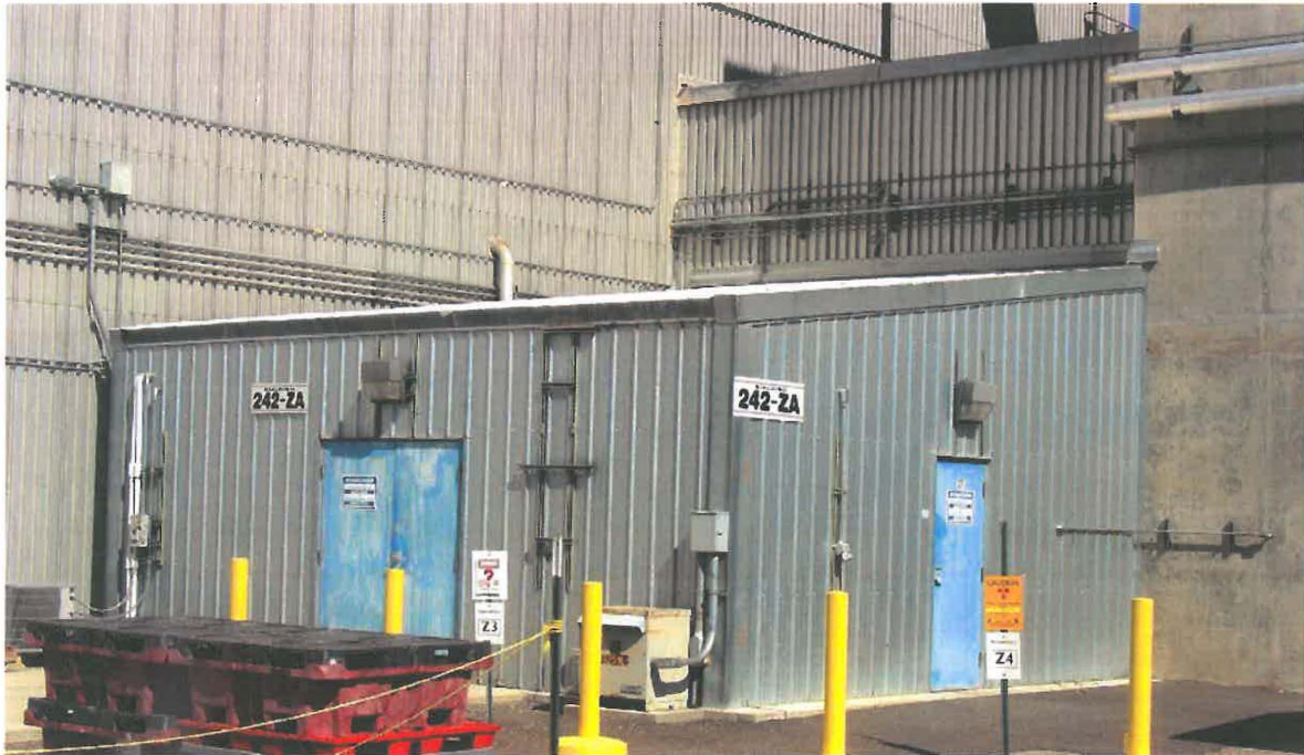
Figure 1. 242ZA Building Pre-Demolition
