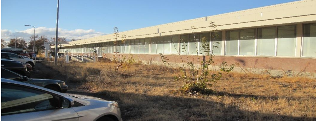
10 11 Figure 4. RTL 520 – Main Building
