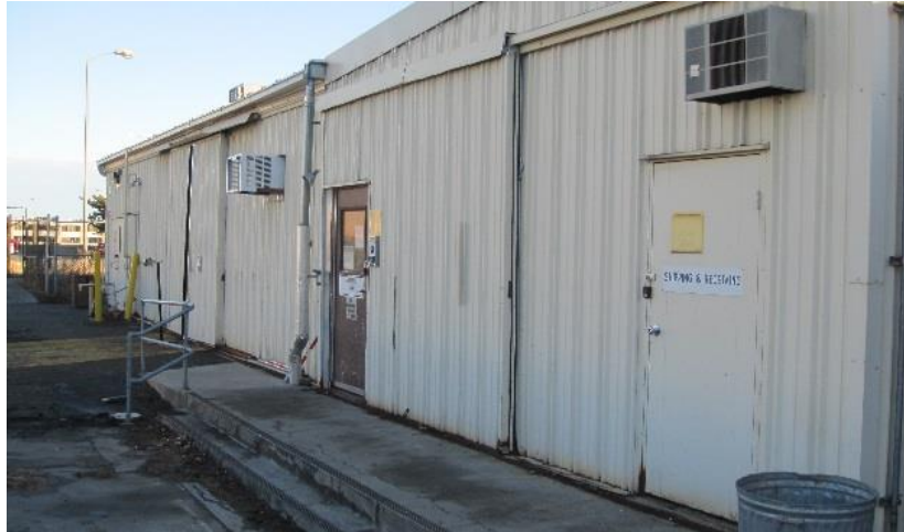
5 6 Figure 8. RTL 550 – Technical Services Building
