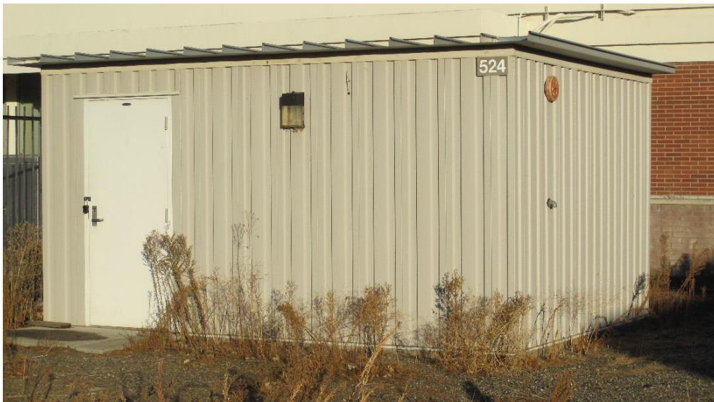
16 17 Figure 5. RTL 524 – Fire Riser Building
