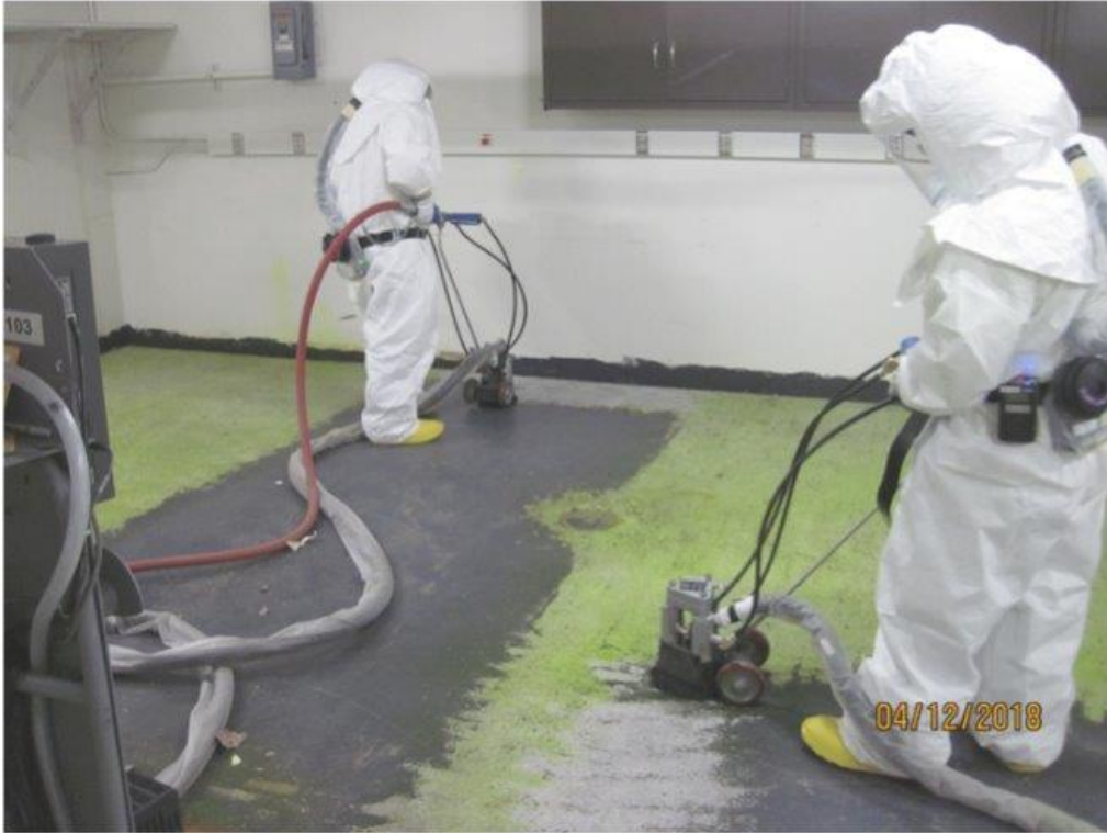
Figure 14. Fixed Radiological Decontamination (Scabbling)
