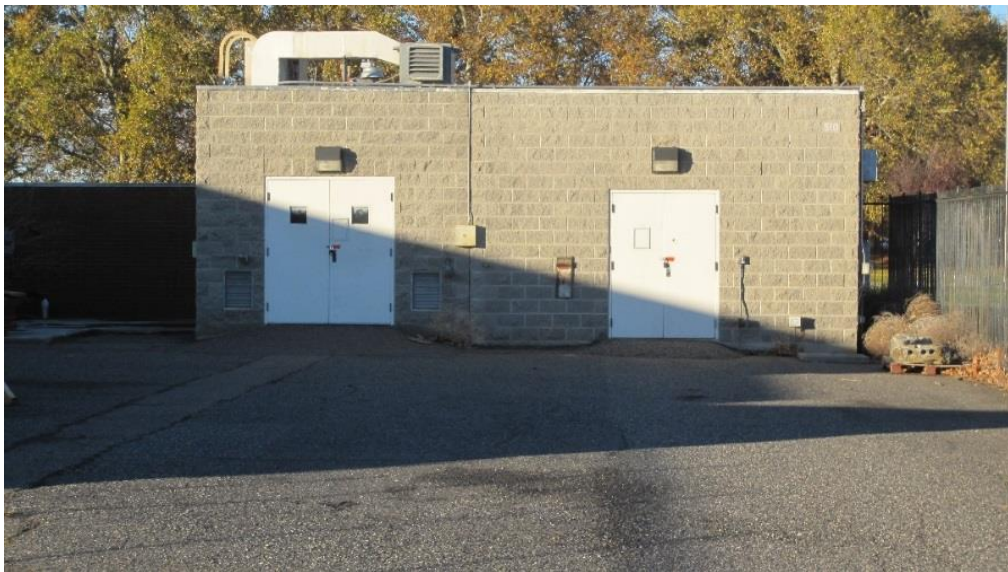
7 8 Figure 3. RTL 510 – Support Building
