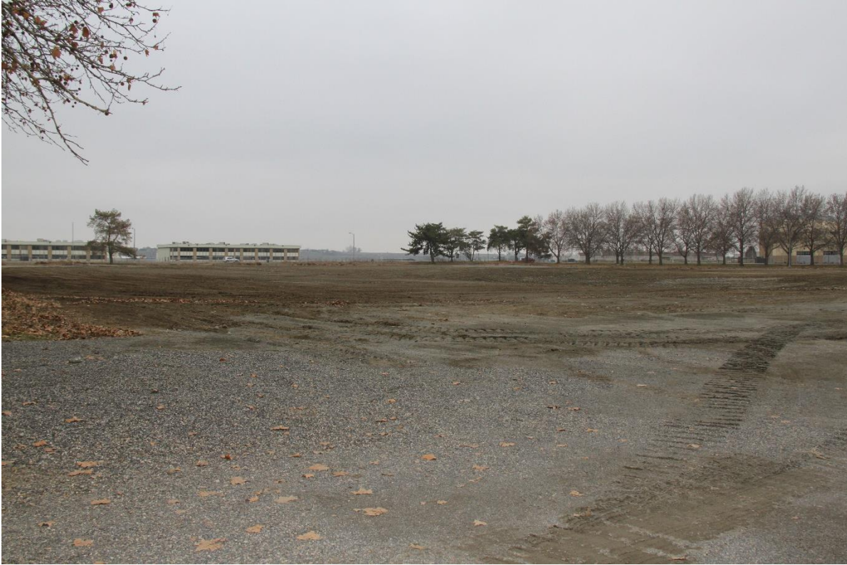
Figure 18. RTL Complex After Partial Backfill and Site Stabilization
