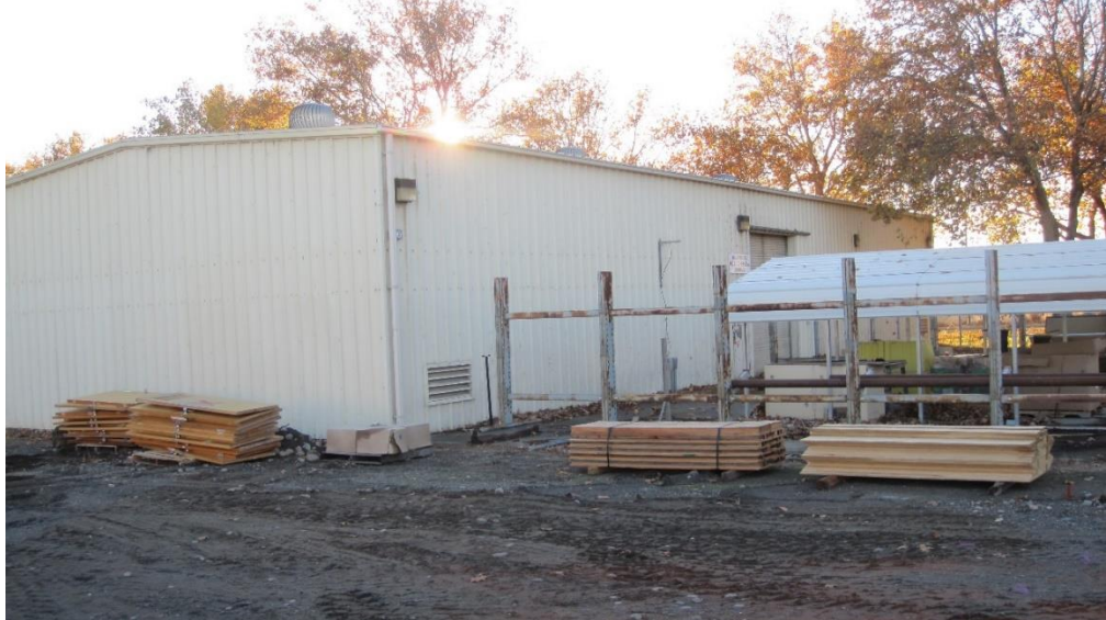
5 6 Figure 12. RTL 590 – Hazardous Waste Chemical Storage/Warehouse
