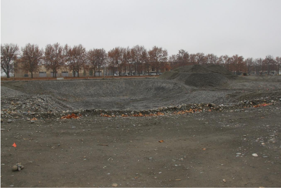
Figure 16. RTL Complex After Demolition and Excavation
