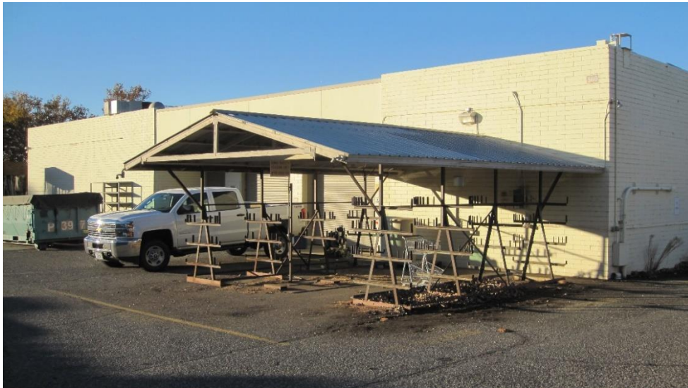
17 18 Figure 9. RTL 560 – Utility Building
