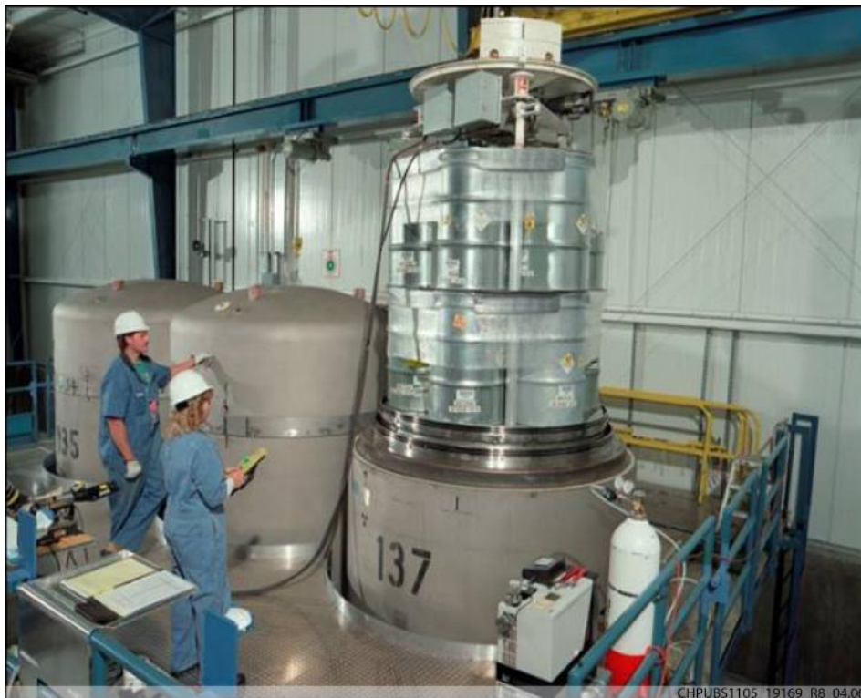
Figure 5-2. Loading a TRUPACT-II with TRUM Waste Drums at WRAP
