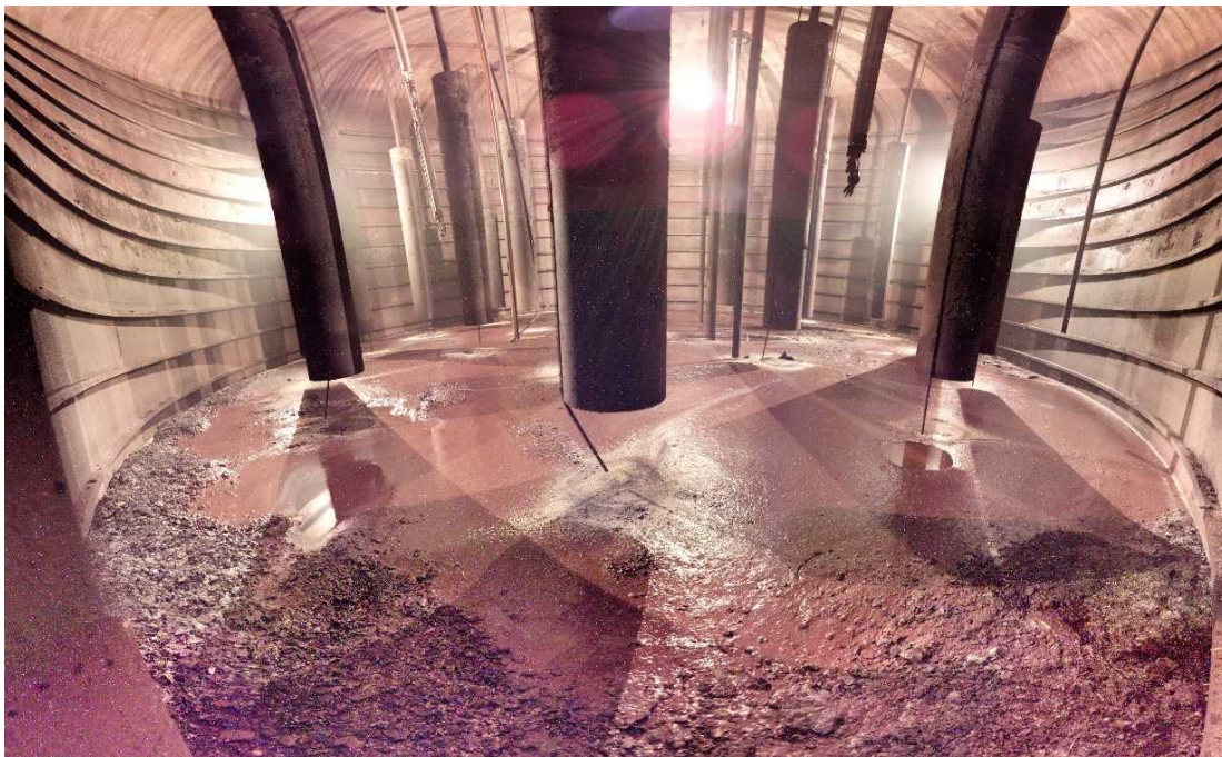
Figure 2-3. Tank 241-AX-103 High-Resolution Photo of the Tank Interior, June 6, 2022.
