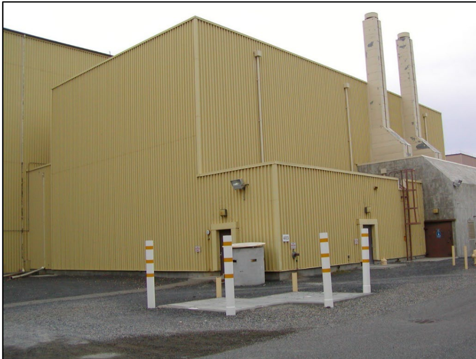
Figure 2. 403 Fuel Storage Facility
