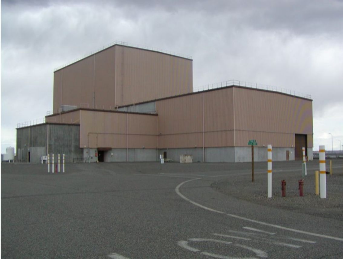
Figure 22. 437 Maintenance and Storage Facility (MASF)
