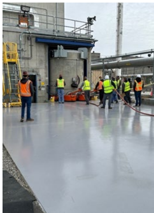
APT/Production CSS Being Staged for Loading
